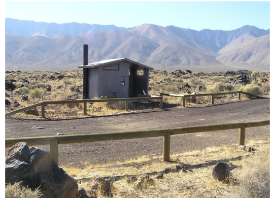
Fossil Falls Campground Accessible Vault Toilet
