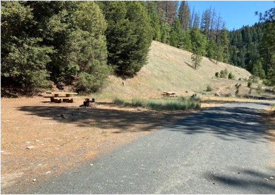
Steiner Flat Campground - proposed for improvement
