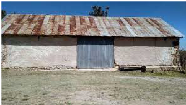
New metal roof for the Adobe Hay Barn
