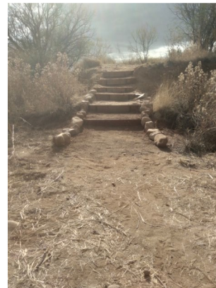
New trail steps constructed at Murray Springs
