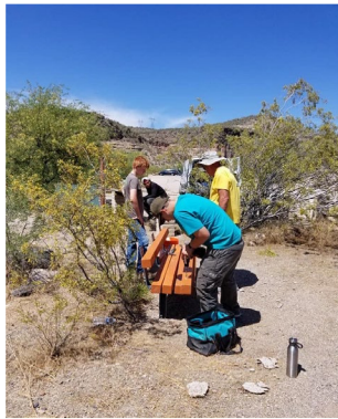
Scouts refurbish benches at Burro Creek Campground
