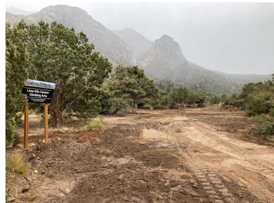
Completed Parking Area at Lime Kiln Canyon Climbing Area
