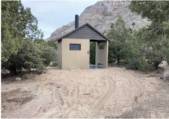
New Vault Toilet at Lime Kiln Canyon Climbing Area
