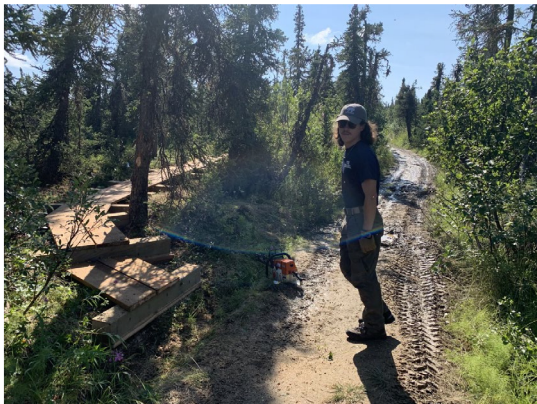
SCA crew members construct new boardwalk
