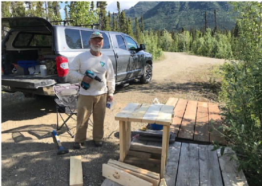
Volunteer working at Marion Creek Campground
