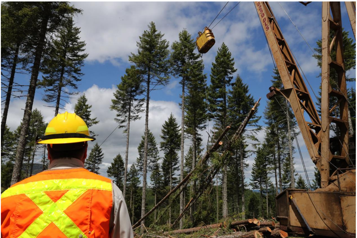
Photo of person watching log yarder at the Rowell Creek Timber Sale located nine miles southwest of Willamina, Oregon. Photo by Michael Campbell, BLM, June 2018.
