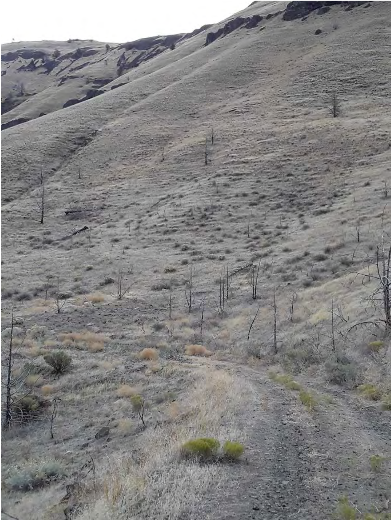
Image 2. Road making a curve.
