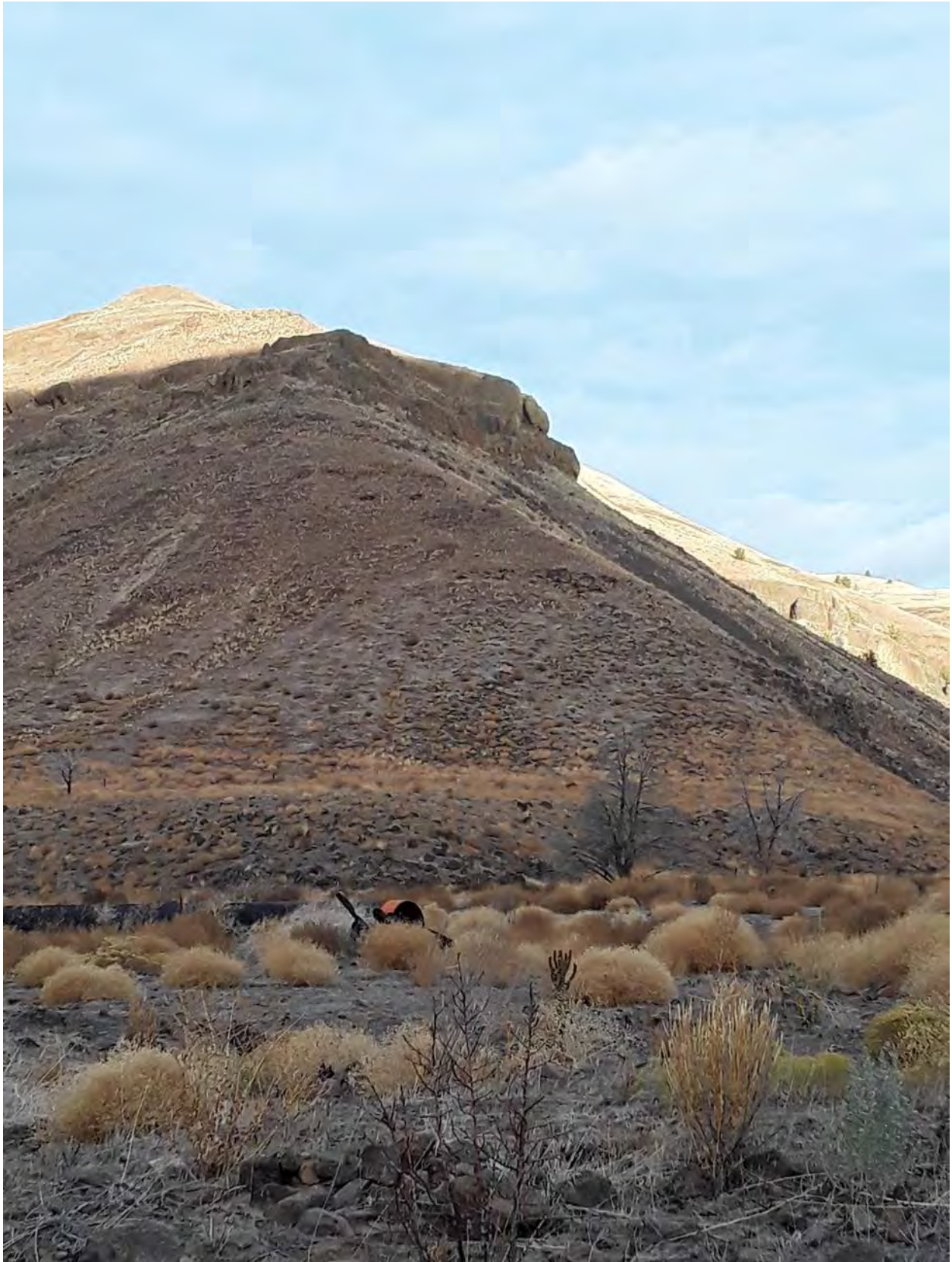
Image 1. TransCanada GTN Pipeline adjacent to road
