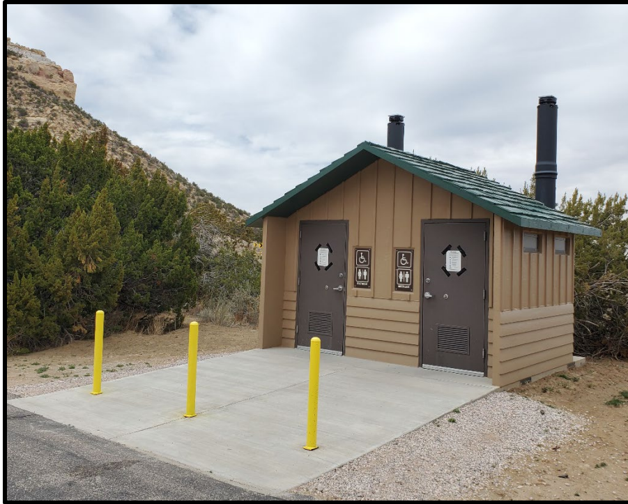
La Ventana ADA Accessible Vault Toilets
