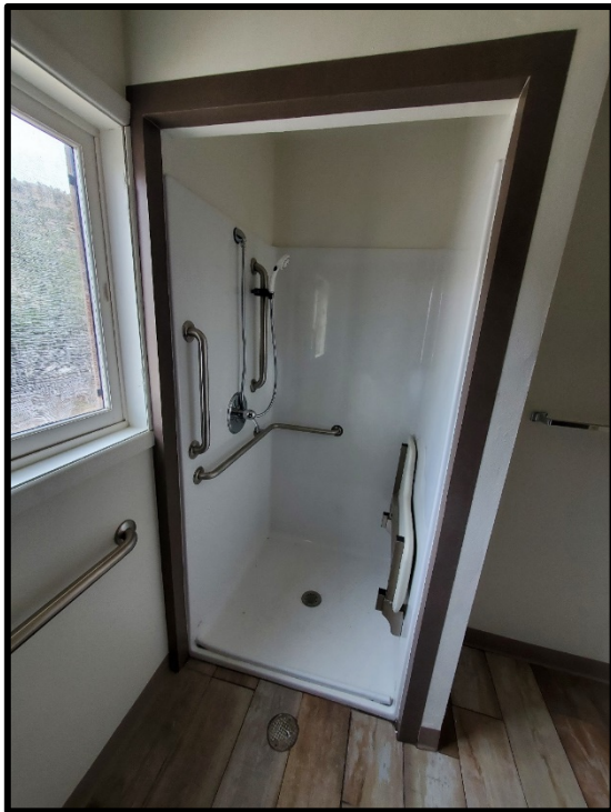
Ranger Station Newly Renovated ADA Accessible Shower
