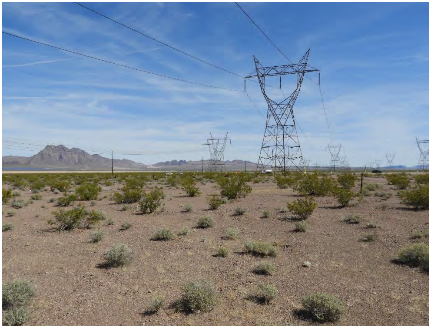
Figure 3. Boulder City to Primm South Utility Corridor @ 0 miles distance.
