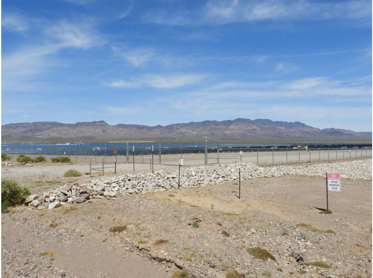
Figure 7. Boulder City to Primm South Utility Corridor @ 1.9 miles distance.
