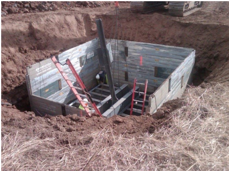
Figure 5-21. Grillage Foundation in Form
