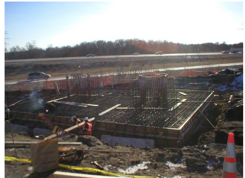
Figure 5-20. Spread Footing Foundation
