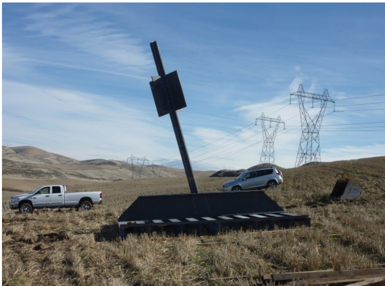
Figure 5-22. Grillage Structure
