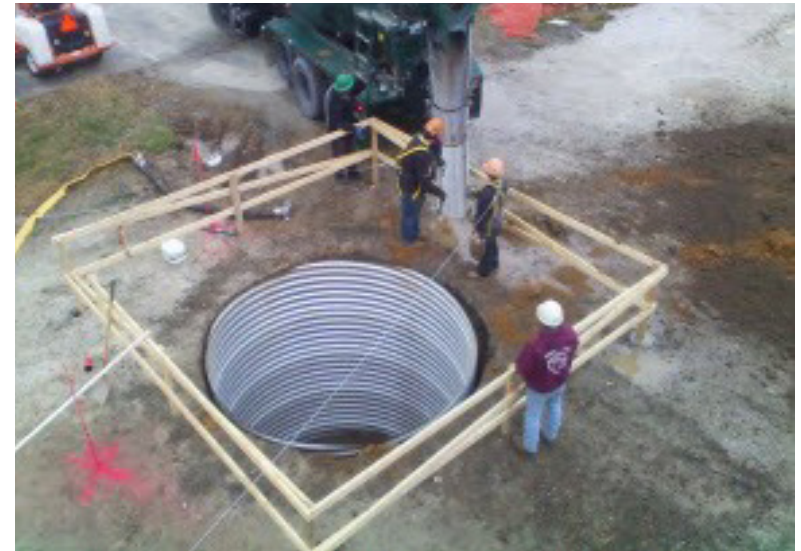
Figure 5-19. Caisson Concrete Pier Foundation
