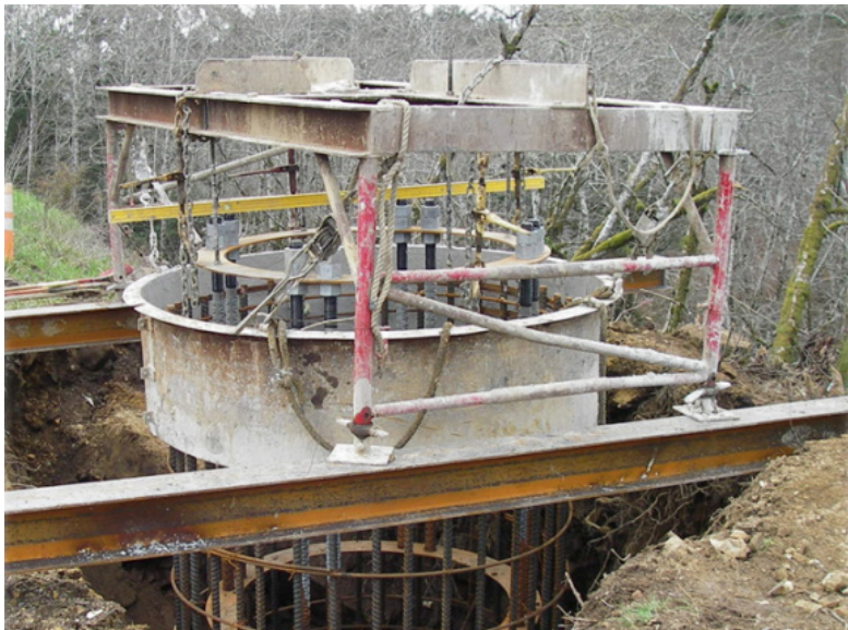
Figure 5-16. Mounting Bolt Cage with Concrete Forms
