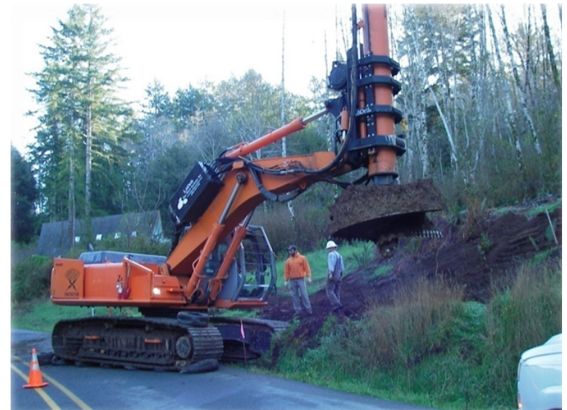
Figure 5-13. Drilling hole for Concrete Pier Foundation
