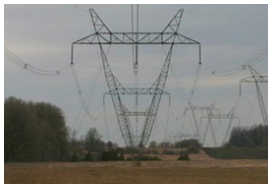
Figure 5-10. 765 kV guyed V structure with guy wires and four conductors per phase
