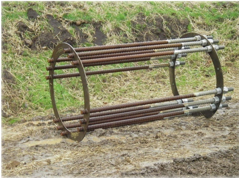
Figure 5-15. Foundation Bolt Cages
