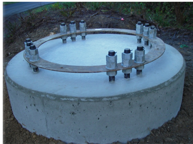
Figure 5-17. Concrete Pier Foundation
