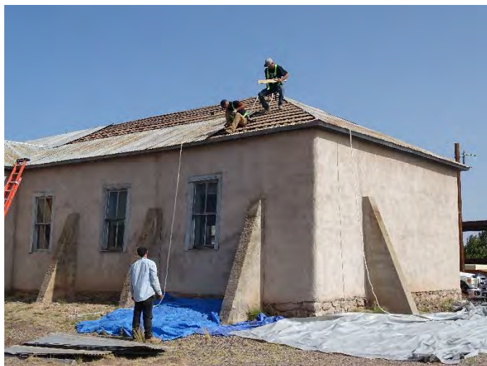
Photo 13. Removal of original sheet metal roof of the School House by personnel from Cornerstones.
