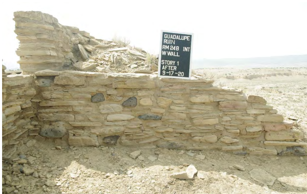
Photo 11. West wall after restoration.
