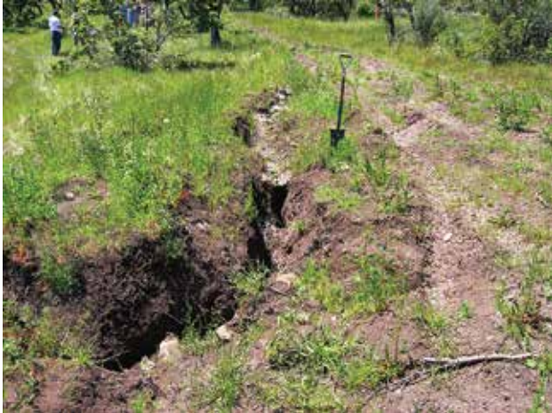
Formation of a gully from runoff from a large rill off the road. Note the beginning of the gully at the headcut near the shovel.
