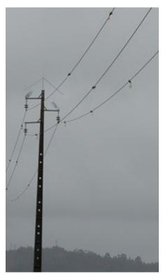
Impacts with conductors have been known to cause blunt force trauma to avian species and it is common to place bird diverters on the conductors to mitigate collisions (as shown in Figure 5-8) particularly in areas with significant migratory and raptor bird populations. Avian impacts must be considered, if possible, in any study related to siting a transmission line and the APLIC publication on reducing avian collisions with power lines can be referenced.
