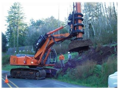
Figure 5-14. Positioning Rebar Cage
