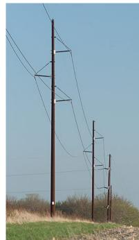
Disadvantages of wood poles include generally shorter life spans than steel poles or lattice poles, less control over the quality, higher susceptibility to fire damage, and increased risk of damage from wildlife. The high probability of damage from woodpeckers and insects can affect the decision on whether wood versus steel should be used for a given transmission line.
