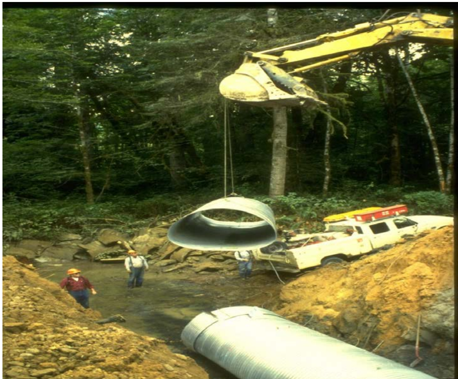
Culvert construction in western Oregon.
