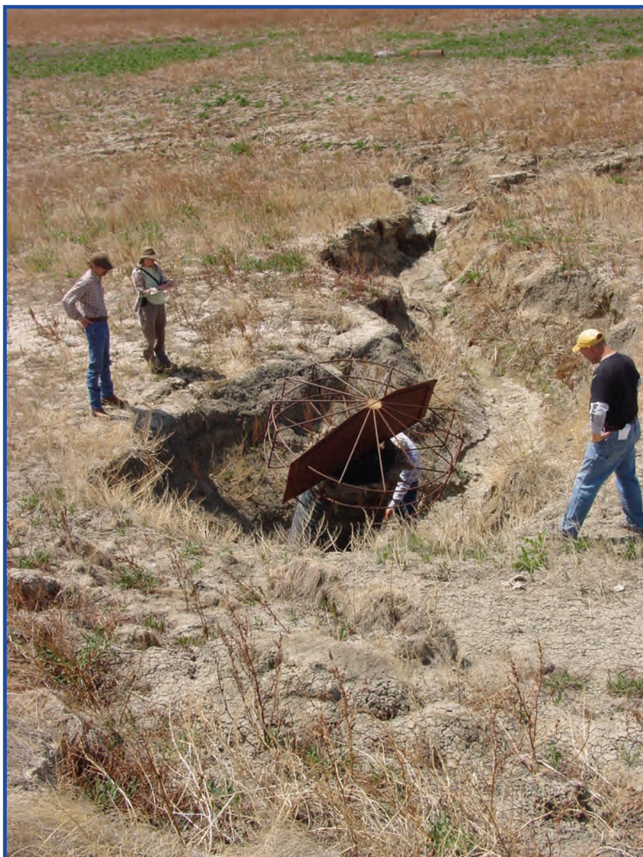
The Blackfoot Dam's failed drop pipe in May 2012 and the eroding channel in the drained reservoir.
