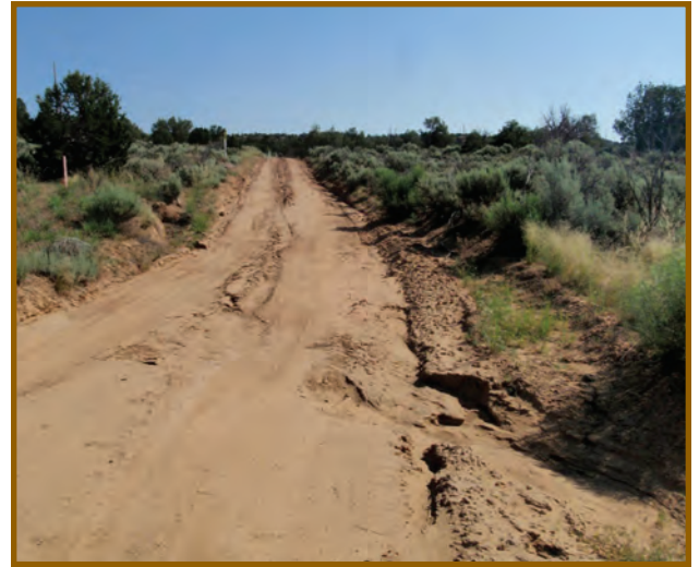
An eroding and below grade road prior to making treatments to reduce sedimentation in the Simon Canyon watershed.
