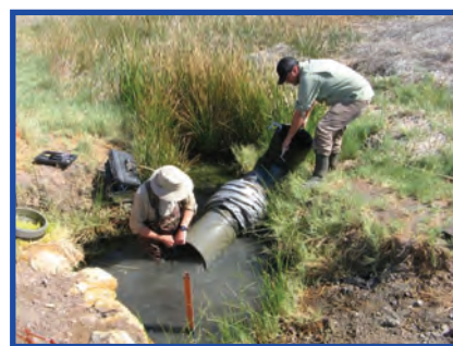
California Department of Fish and Wildlife employees install standpipe to increase inundation and soil moisture in critical habitat for the Amargosa vole.
