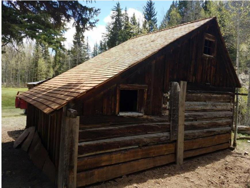
After stabilization with a new shingle roof and three new foundation logs.
