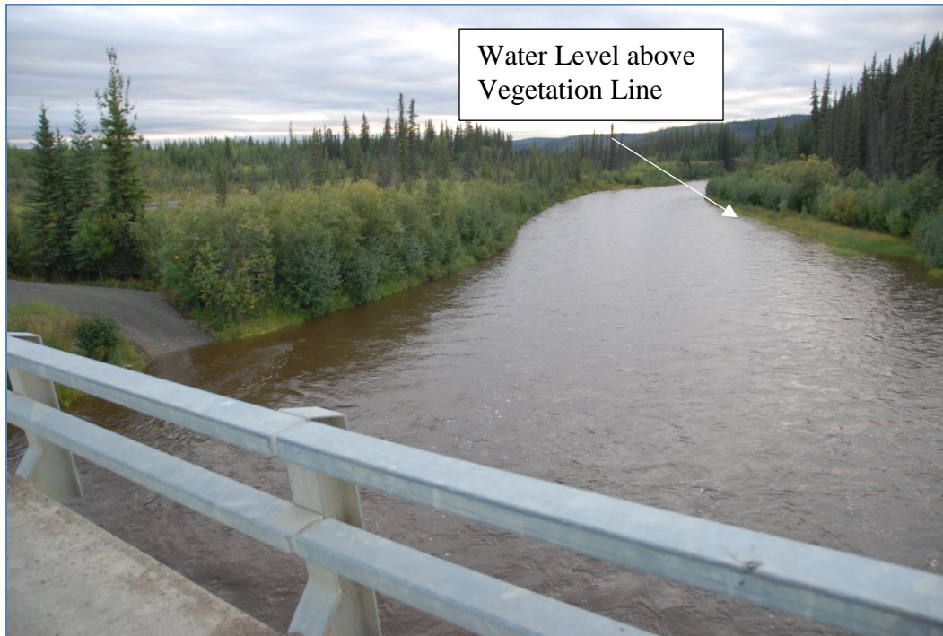
Figure 3a. Upstream view of West Fork Dennison channel at high flow, stream gage water level = 7.7 feet. Taylor Highway Bridge MP49, 2015 hours, August 22, 2018.
