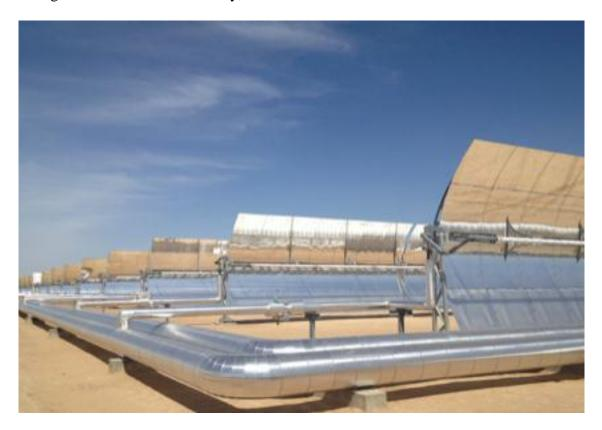
The project will consist of two independent solar electric generating facilities with a nominal net electrical output of 125 megawatts (MW) each, for a total net electrical output of 250 MW. Electrical power will be produced using steam turbine generators fed from solar steam generators. The solar steam generators receive heated transfer fluid from solar thermal equipment comprised of arrays of parabolic mirrors that collect energy from the sun.
