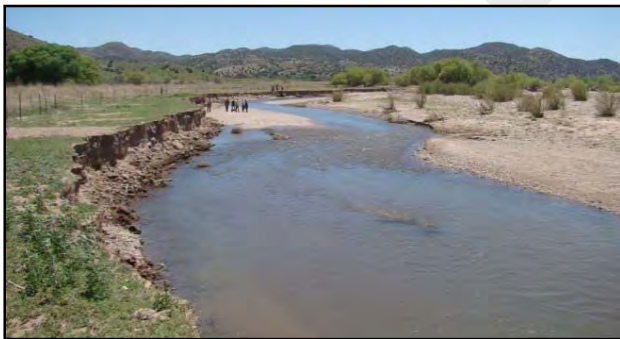
Figure 33. Bank erosion in an unstable channel.
