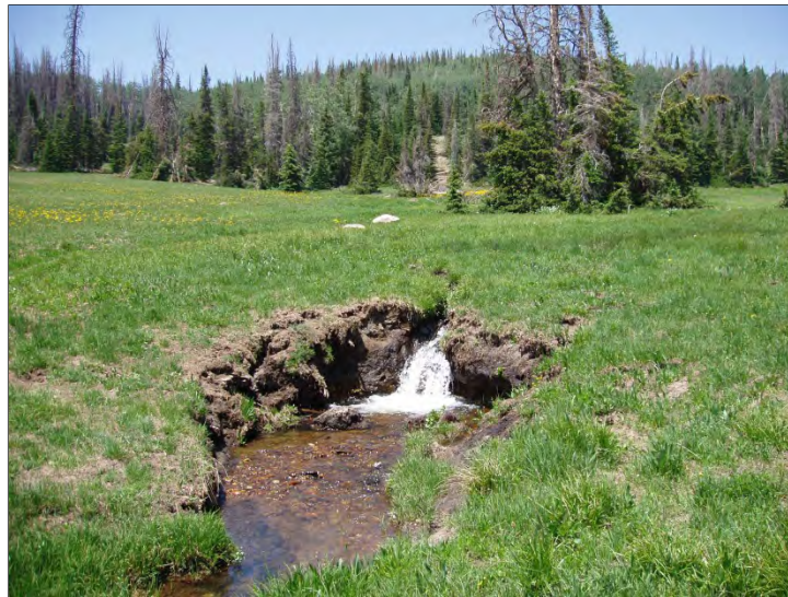
11 12 Figure 7. Headcut is moving up through a meadow, making the area above functional-at-risk. 13 14
