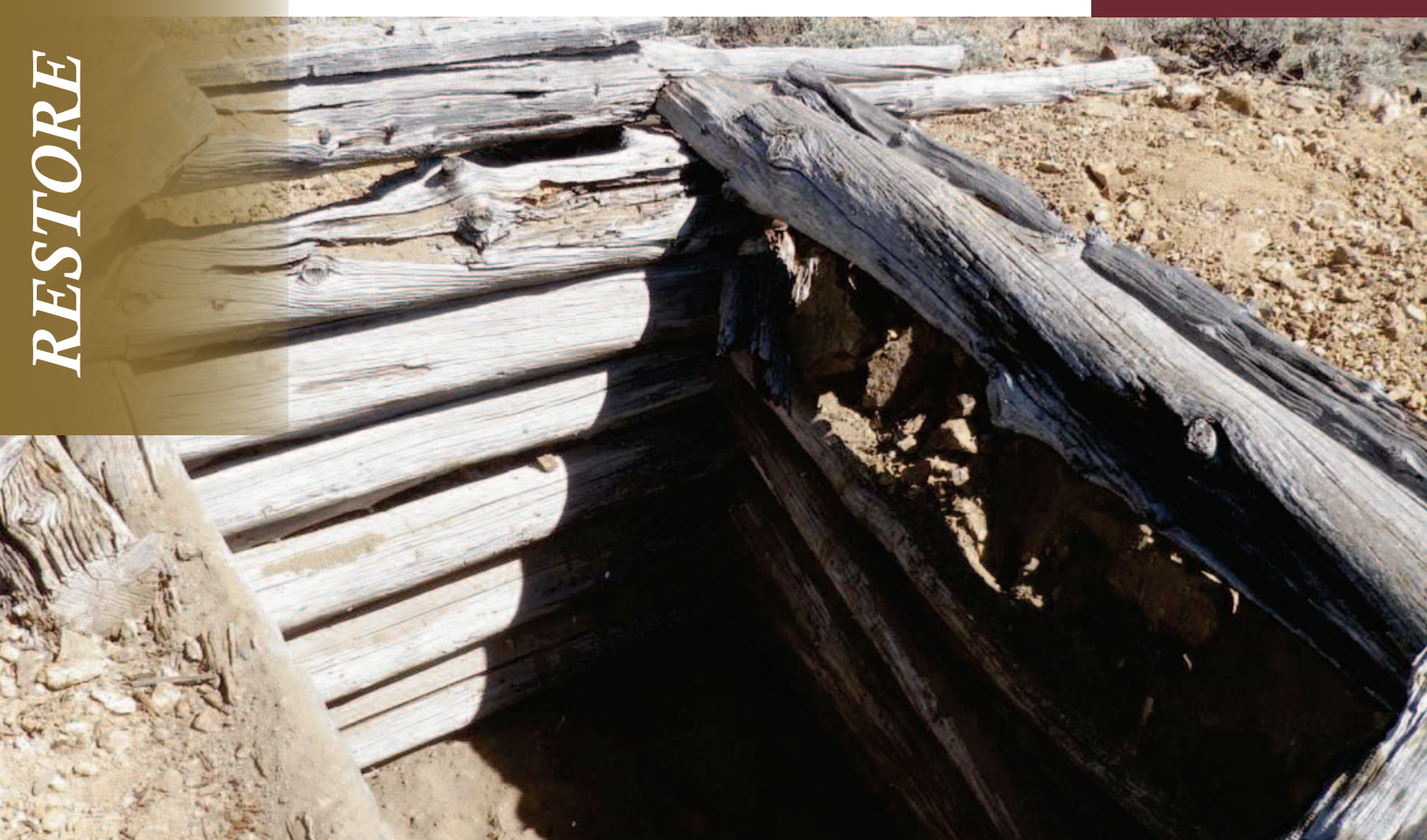
Cribbed shaft closed with polyurethane foam (PUF) plug and backfill at Duncan abandoned mine site.
