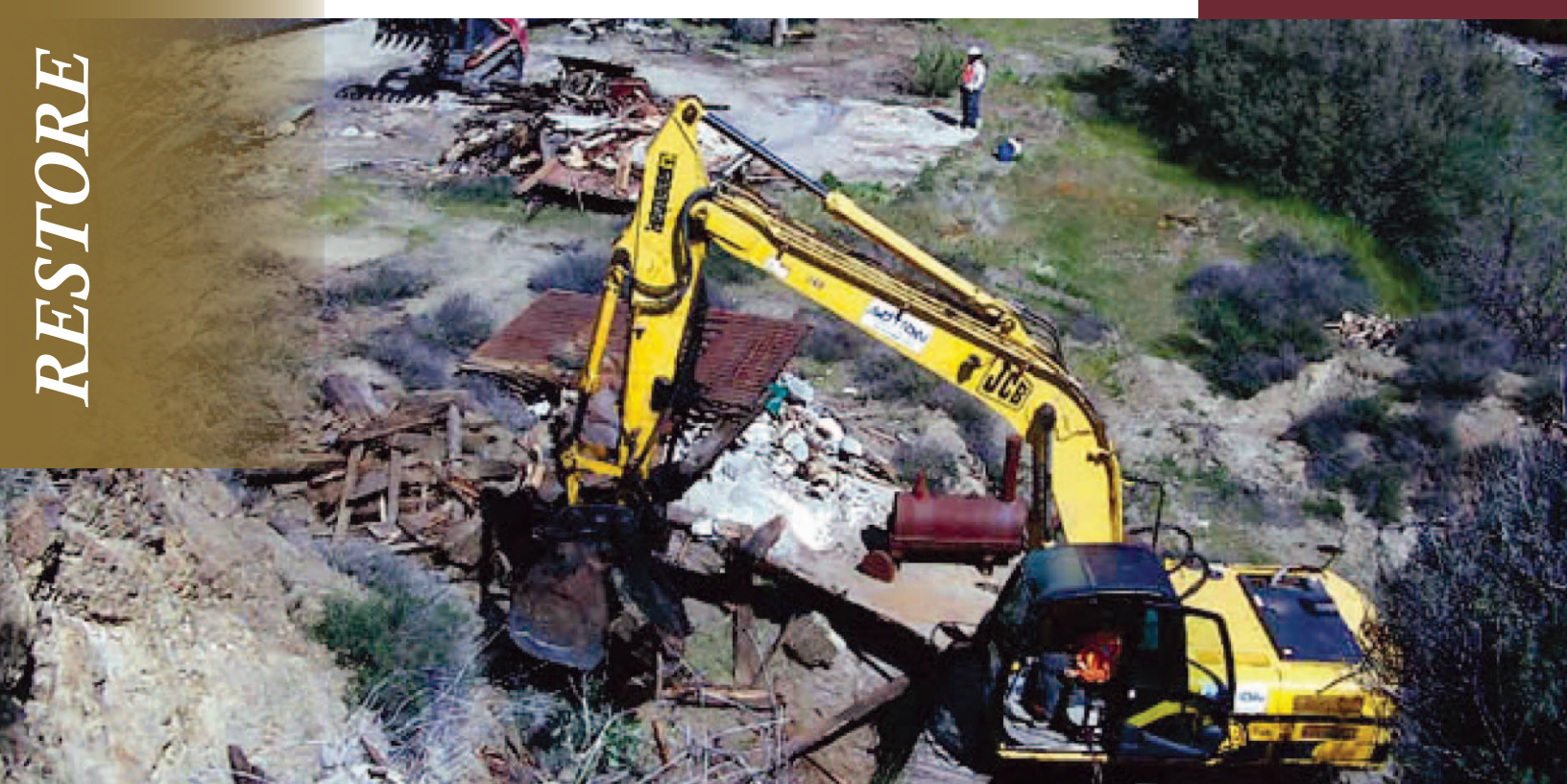
Removed 50 tons of contaminated mercury mine waste from the abandoned Archer mine and mill site in Fresno County, CA protecting the White Creek watershed and the wildlife and local residents downstream.
