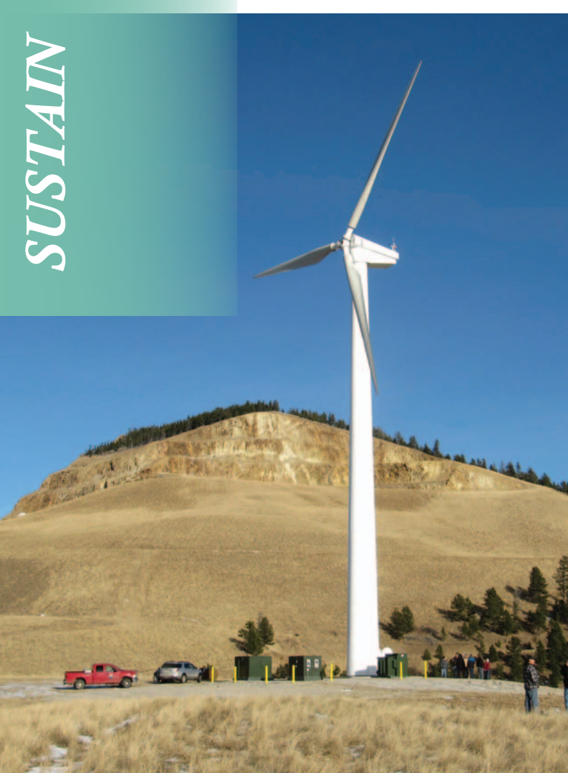
Installation of a 225kW wind turbine at the Zortman-Landusky abandoned mine to offset the long-term water treatment and monitoring energy costs.
