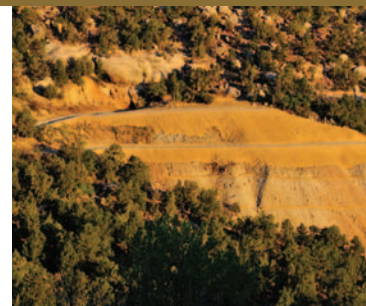
Stabilizing slopes and planting vegetation prevents runoff from the abandoned mines sites from impacting the Sal Creek Watershed.
