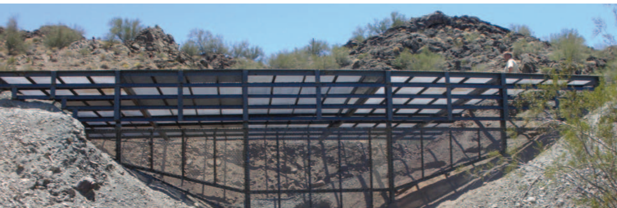
Bat-friendly gate constructed to cover a large open shaft at the Old Swansea abandoned mine in Arizona.
