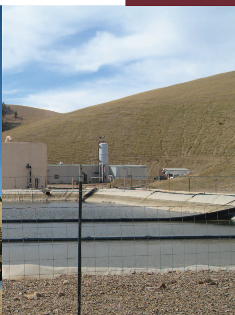
Long-term groundwater monitoring and treatment system at Zortman-Landusky abandoned mine.
