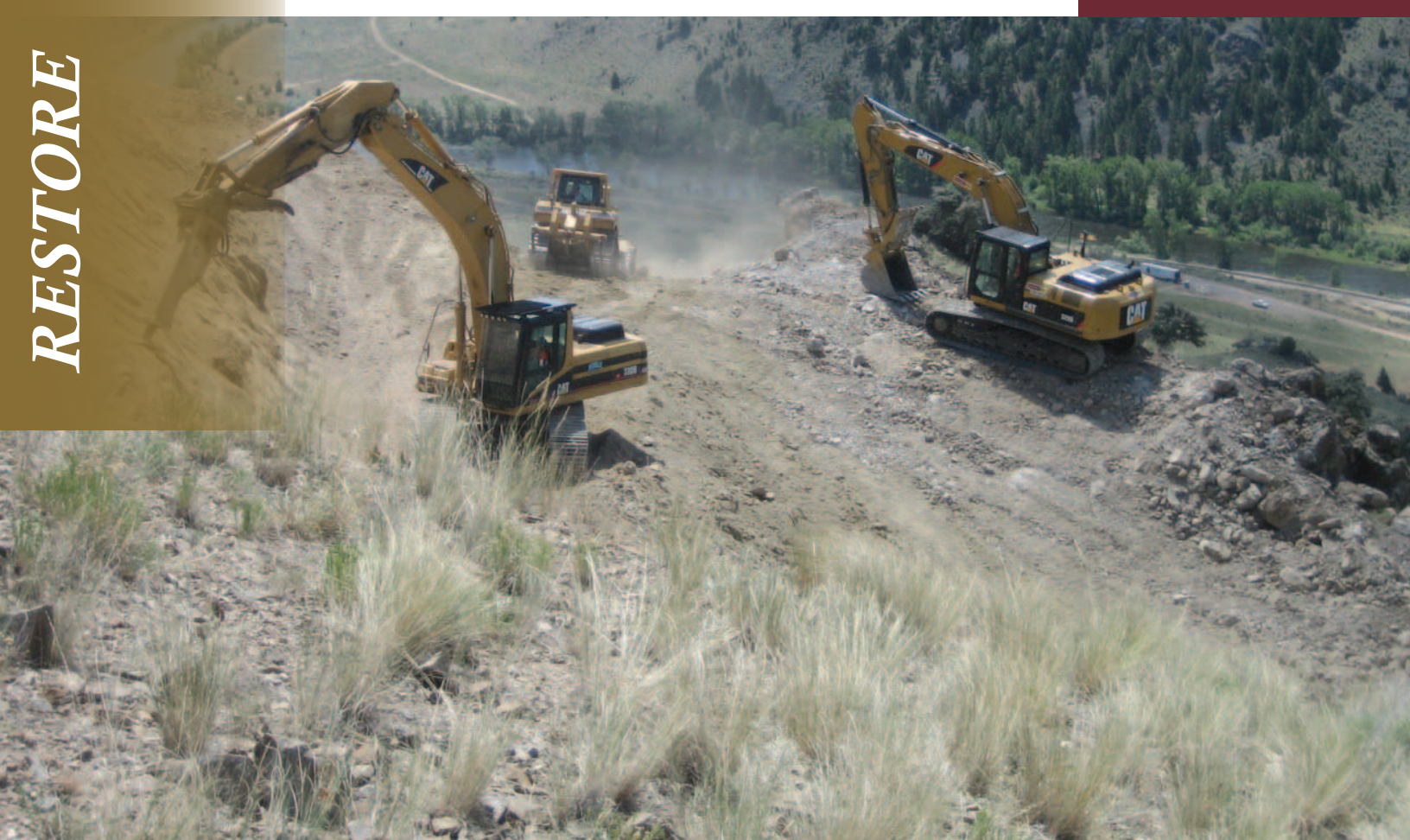
Backfilling collapsed mine features at the Maiden Rock with the Big Hole River in the background.
