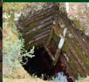
Documented cribbed shaft entrance in the Fairbanks Creek drainage in Alaska.
