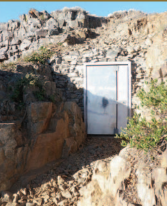
Adit closure at the Duncan abandoned mine site.
