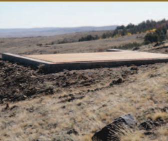
Closure of open shaft at the Duncan abandoned mine site.
