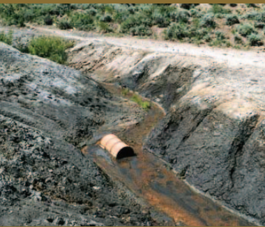
Before restoration shows acidic seepage from the Rip Van Winkle tailings in Coon Creek, a tributary of Maggie Creek and the Humboldt River in northeastern Nevada.
