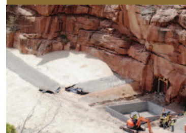
Sealing of horizontal mine adits to stop arsenic and radioactive materials from impacting the Sal Creek Watershed in Utah.
