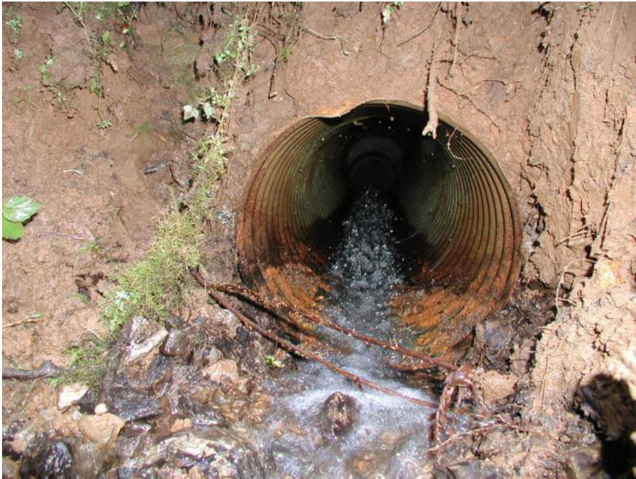
Culvert at North Fork Alsea Access Road. Photo by BLM Northwest Oregon District.
