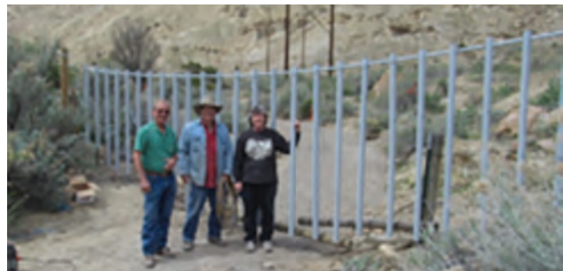
Members of Friends of the Mustangs construct a fence stream crossing.
