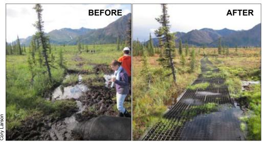
The difference after a year's work on the lack River Trail easement. There is trail braiding, ruts, mud, and trail damage before installing porous grid system trail stabilizers.
