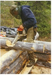
Notching logs with chainsaw.
