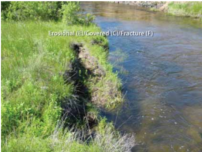
Figure E4. This large fracture has at least 50 percent vegetation cover and is thus recorded as erosional (E), covered (C), and fracture (F).
