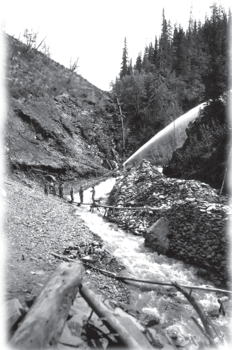
Figure 1: Sluice box operation on Lynx Creek in 1904. Gold-bearing gravel from the stream cut on the right of the photo was shoveled into the sluice box.
