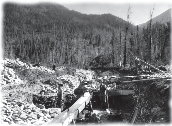
Figure 1: Sluice box operation on Lynx Creek in 1904. Gold-bearing gravel from the stream cut on the right of the photo was shoveled into the sluice box.
