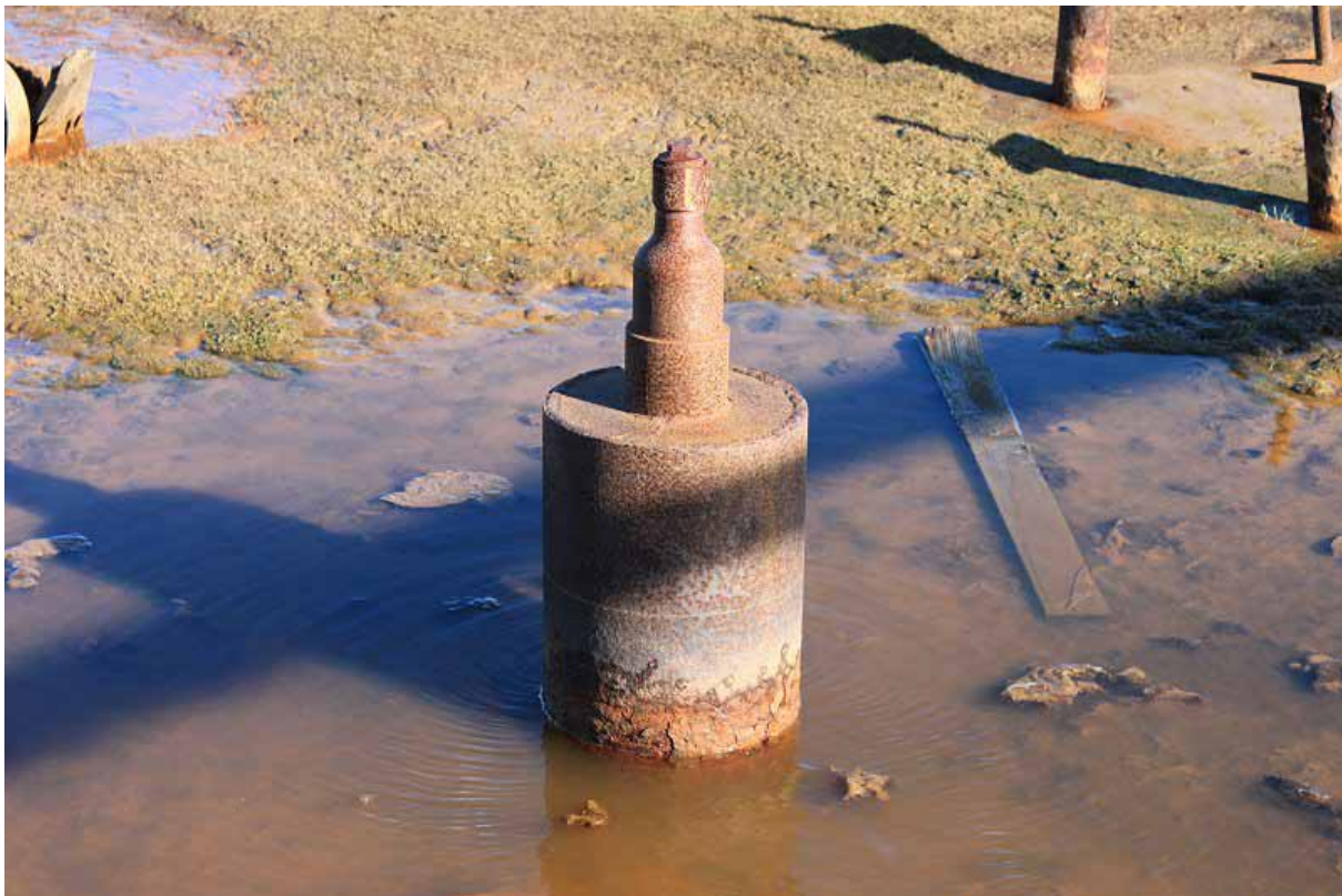
Figure 7: North Simpson #1 wellhead (August 2010).
