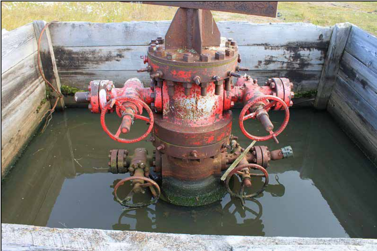
Figure 7: North Inigok #1 wooden cellar filled with water and wellhead (August 2010).
