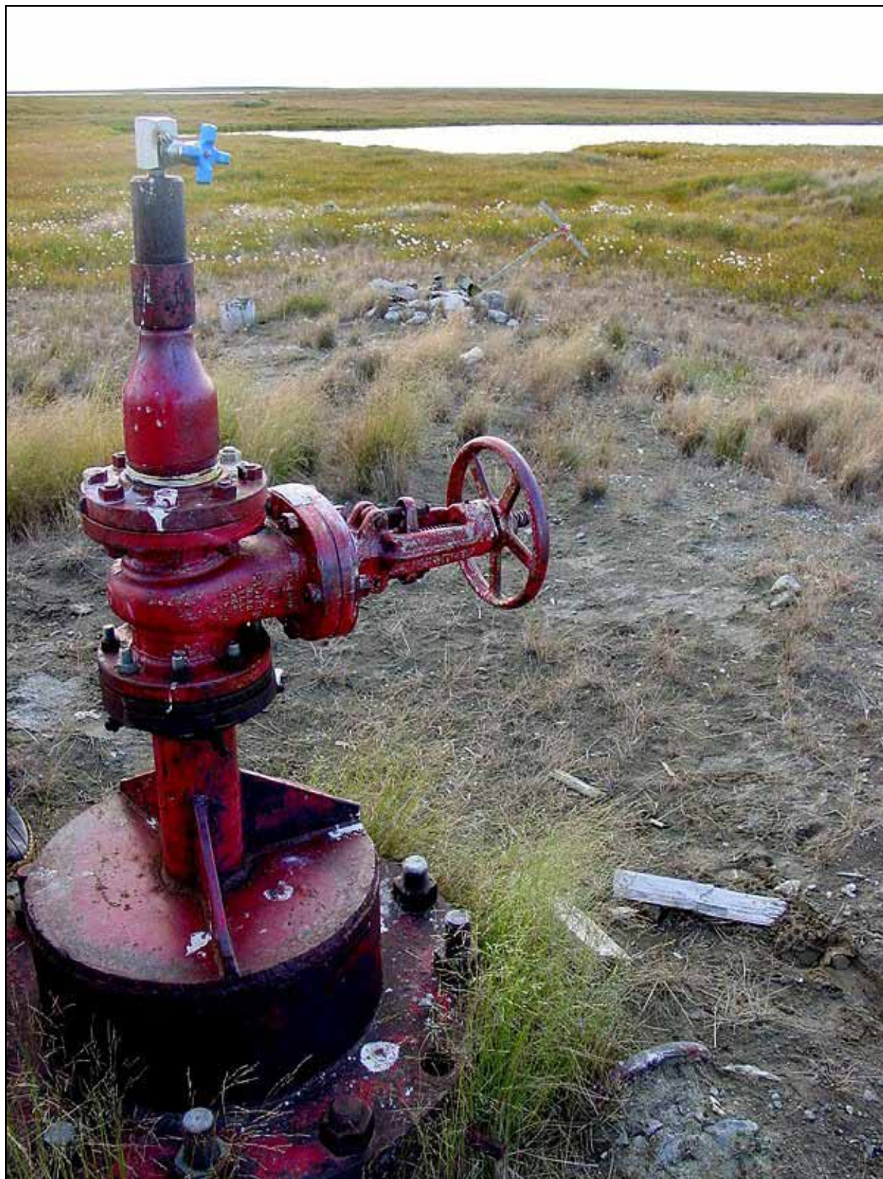
Figure 5: Wellhead on West Fish Creek #1 (August 2002).
