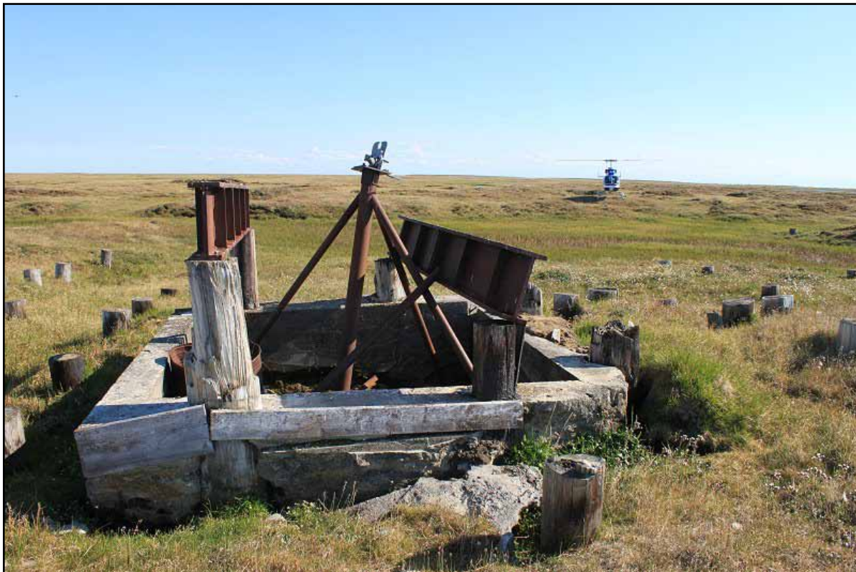
Figure 2: South Barrow #3 has a concrete cellar and steel beams stacked on pilings that were cemented into the cellar. The well is cut off at ground level inside the cellar.
