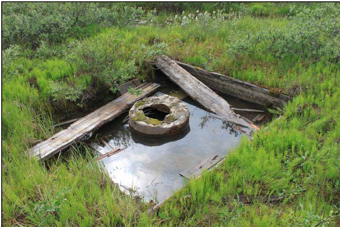
Figure 4: Square Lake #1 contains a wooden cellar full of water and cement around open casing (July 2012).
