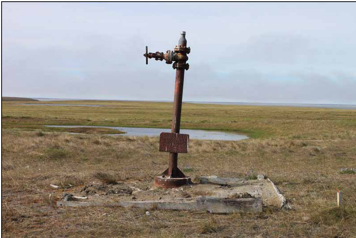
Figure 4: South Harrison Bay #1 wellhead and sandy cellar (July 2012).
