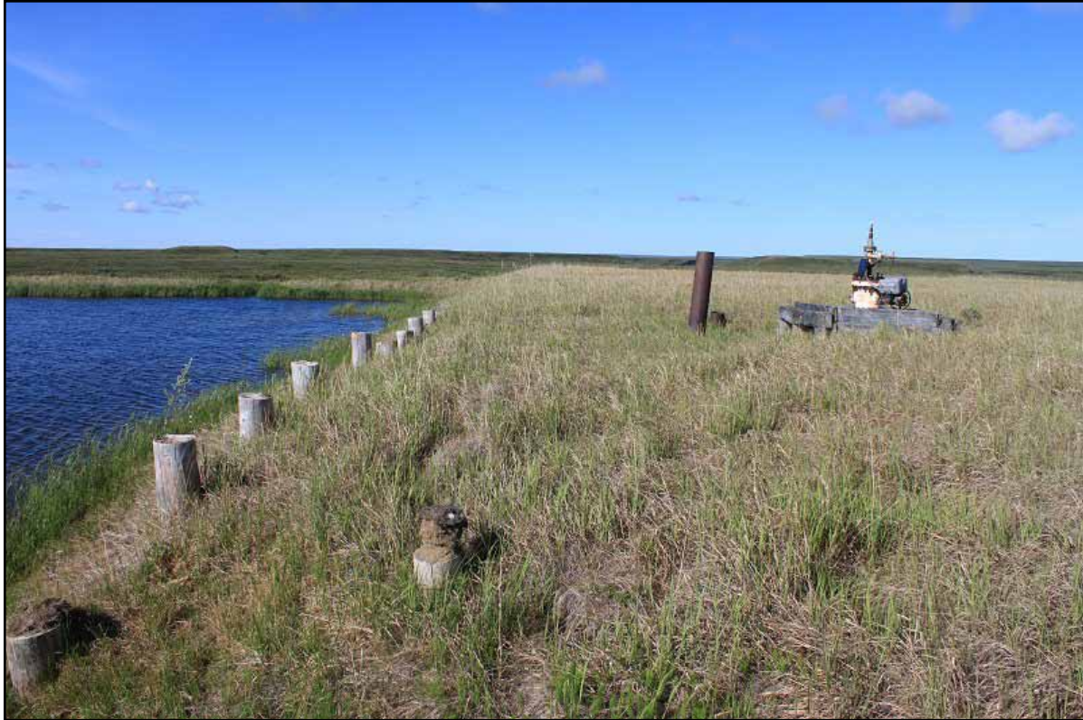
Figure 5: Exposed wooden pilings adjacent to the reserve pit at Koluktak #1 (July 2012).
