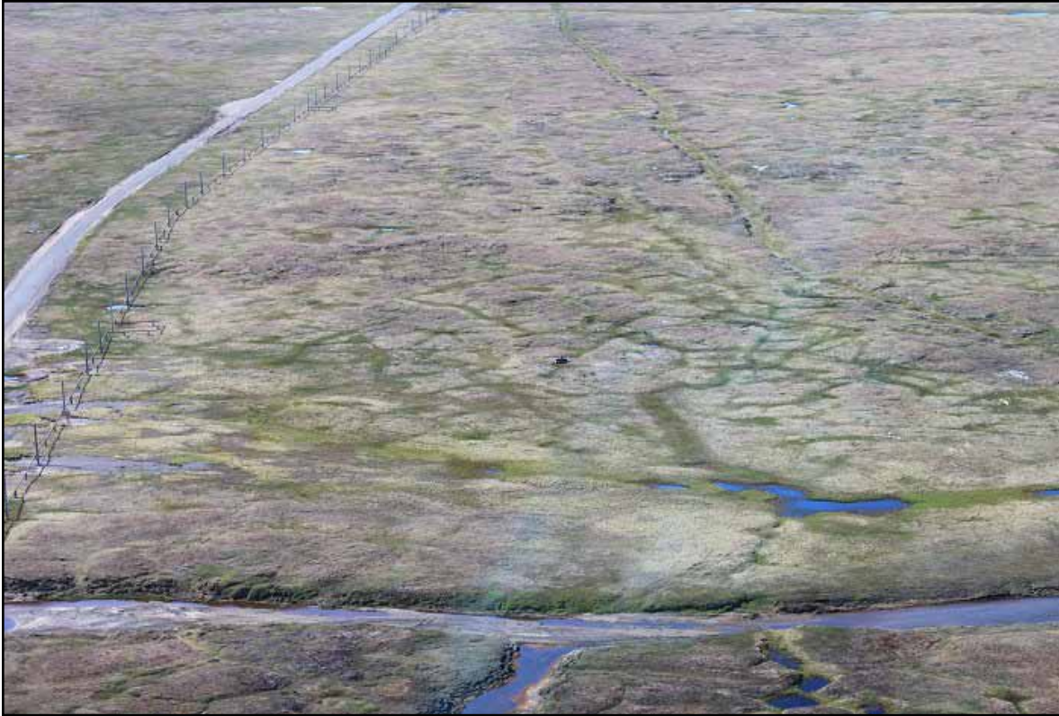
Figure 1: Aerial view of Avak #1 (in center of photo) and access road to the East Barrow Gas Field, with the associated pipeline running east to west. The Mayoek River is in the foreground of the photo.
