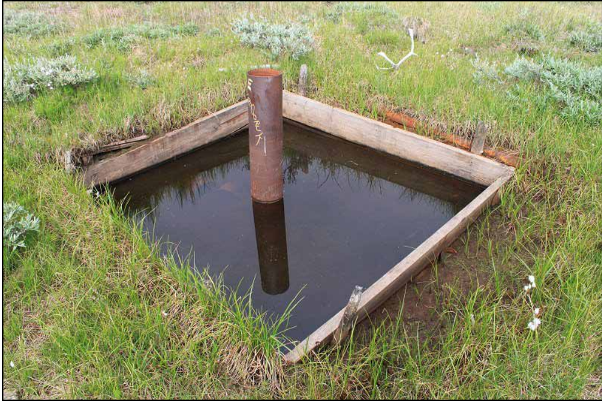
Figure 3: East Topagoruk #1 well and cellar after a normal precipitation pattern.
