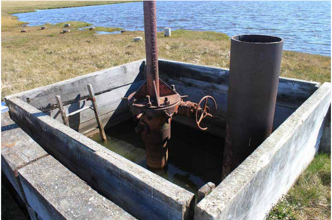
Figure 5: West Dease #1 cellar (filled with water), wellhead, rat hole (July 2012).
