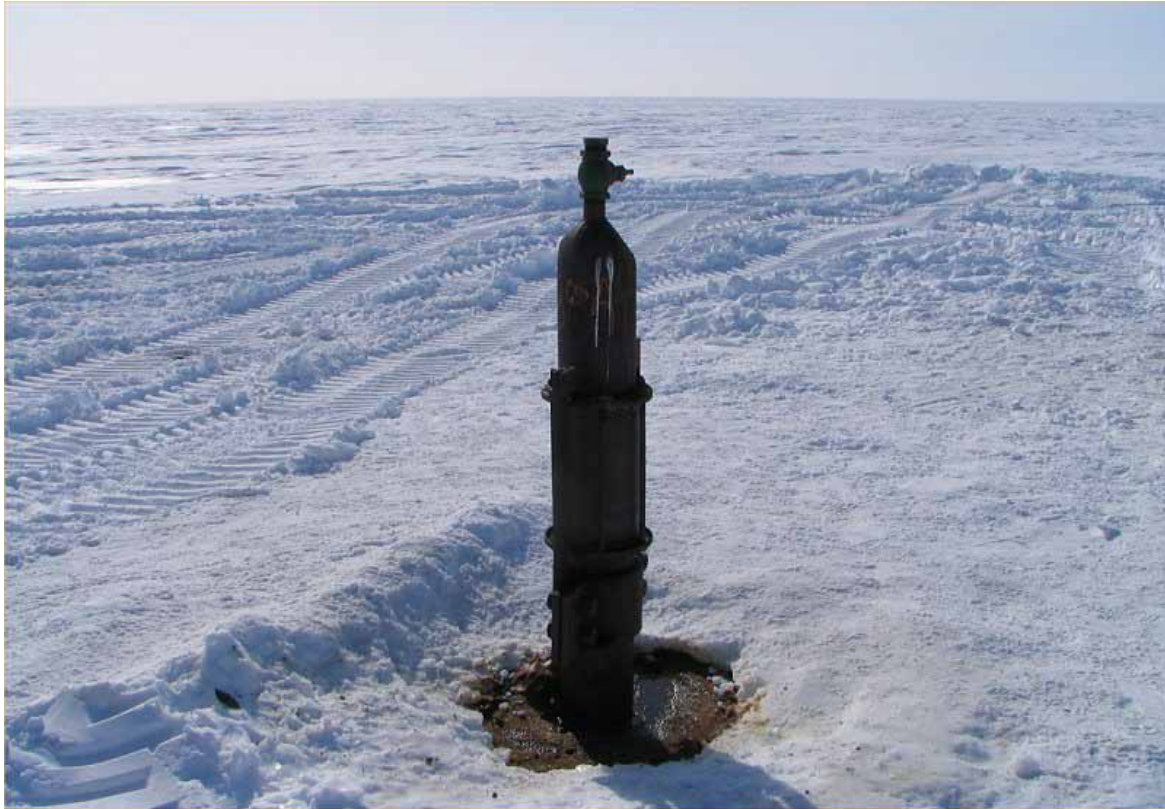
Figure 11: Simpson Core Test #30A after the construction of a thin ice pad used for plugging operations (April 2006).
