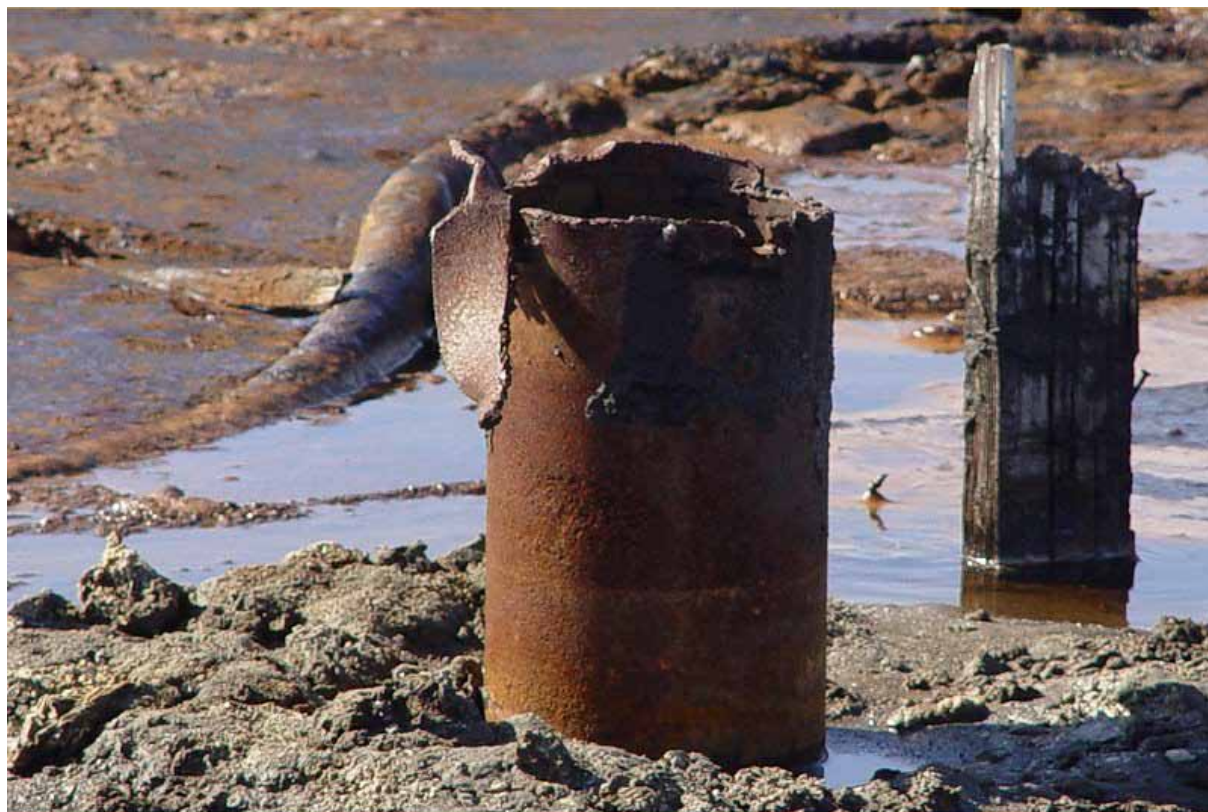
Figure 9: Sheared casing for Simpson Core Test #30 before plugging operations (June 2003).
