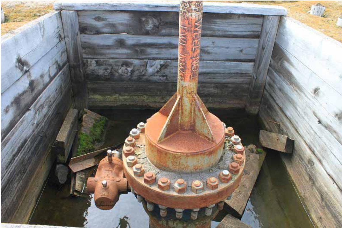
Figure 3: View of the Peard #1 wellhead inside the cellar (July 2012).
