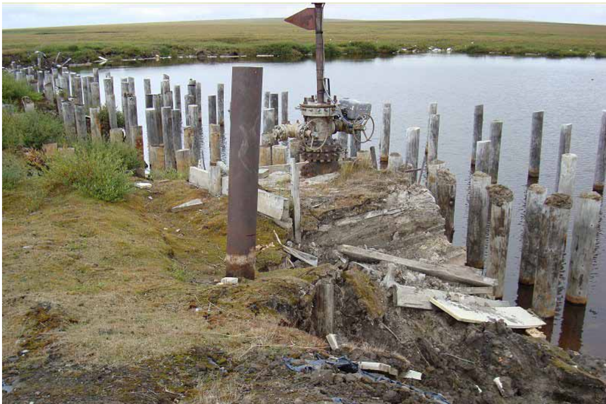
Figure 4: Condition of the Awuna #1 wellhead and pilings in August 2008.
