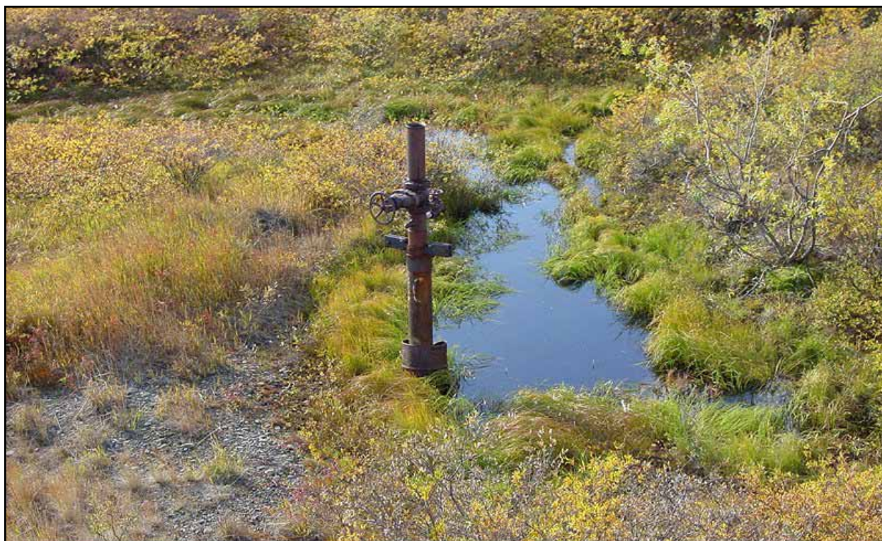
Figure 5: Umiat #10 prior to plugging operations (September 2002).
