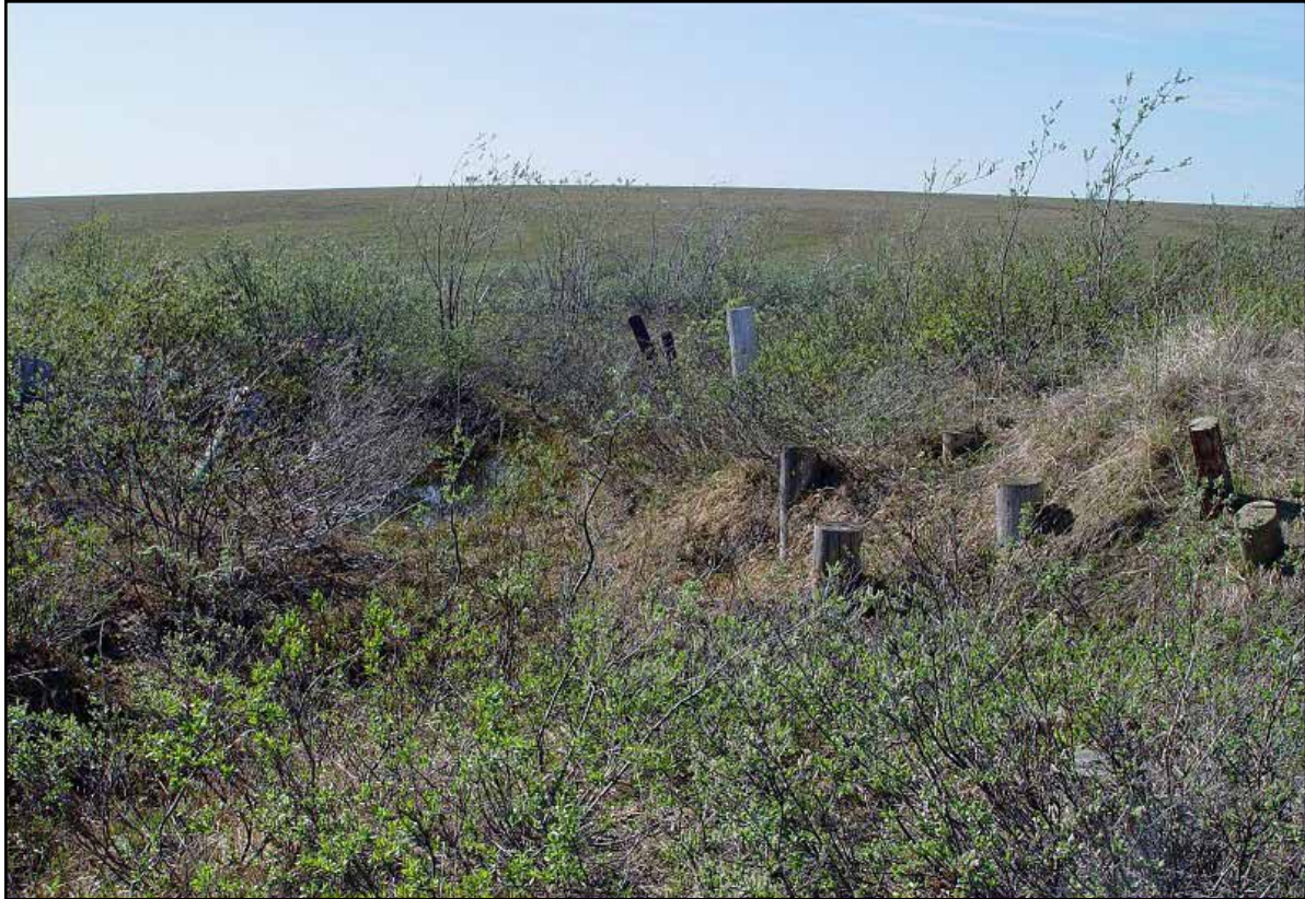
Figure 3: Wood pilings and pipe near Wolf Creek #3 (June 2003).
