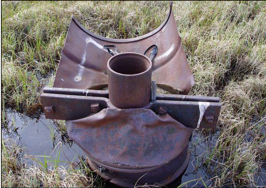
Figure 2: Umiat #7 prior to welding a cover for the open casing (June 2003).
