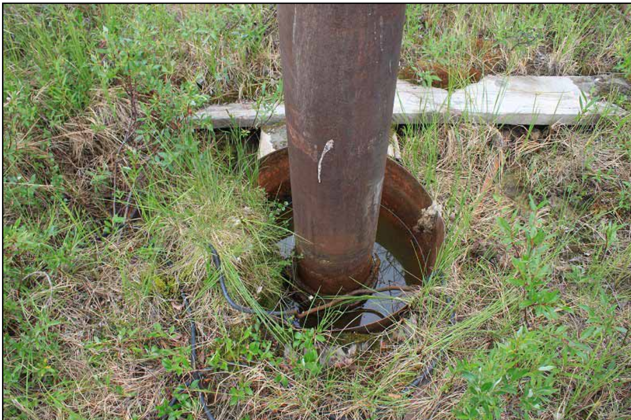
Figure 4: Thermistor cable laying on the ground next to the Umiat #11 well.
