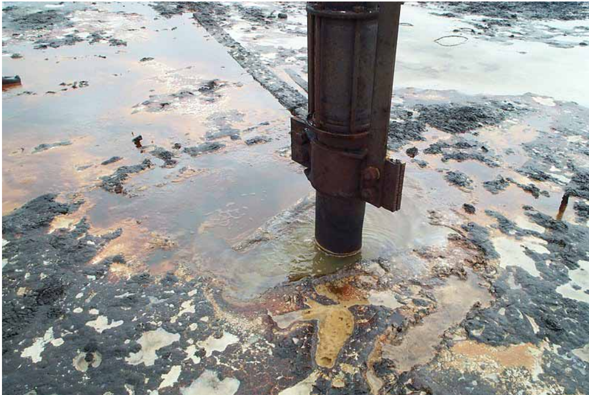
Figure 14: Bubbling around the surface casing of Simpson Core Test #30A (August 2001).
