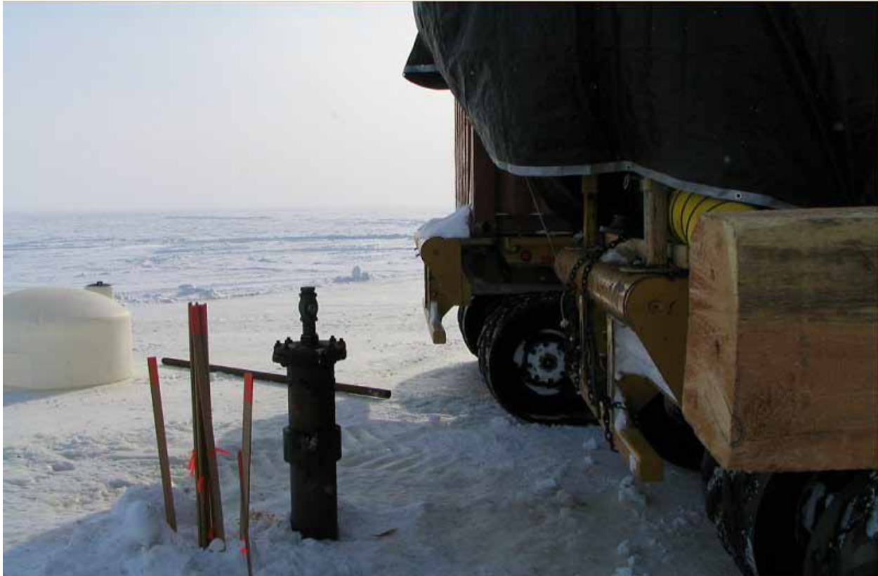
Figure 4: Plugging operations on Simpson Core Test #27 (April 2006).
