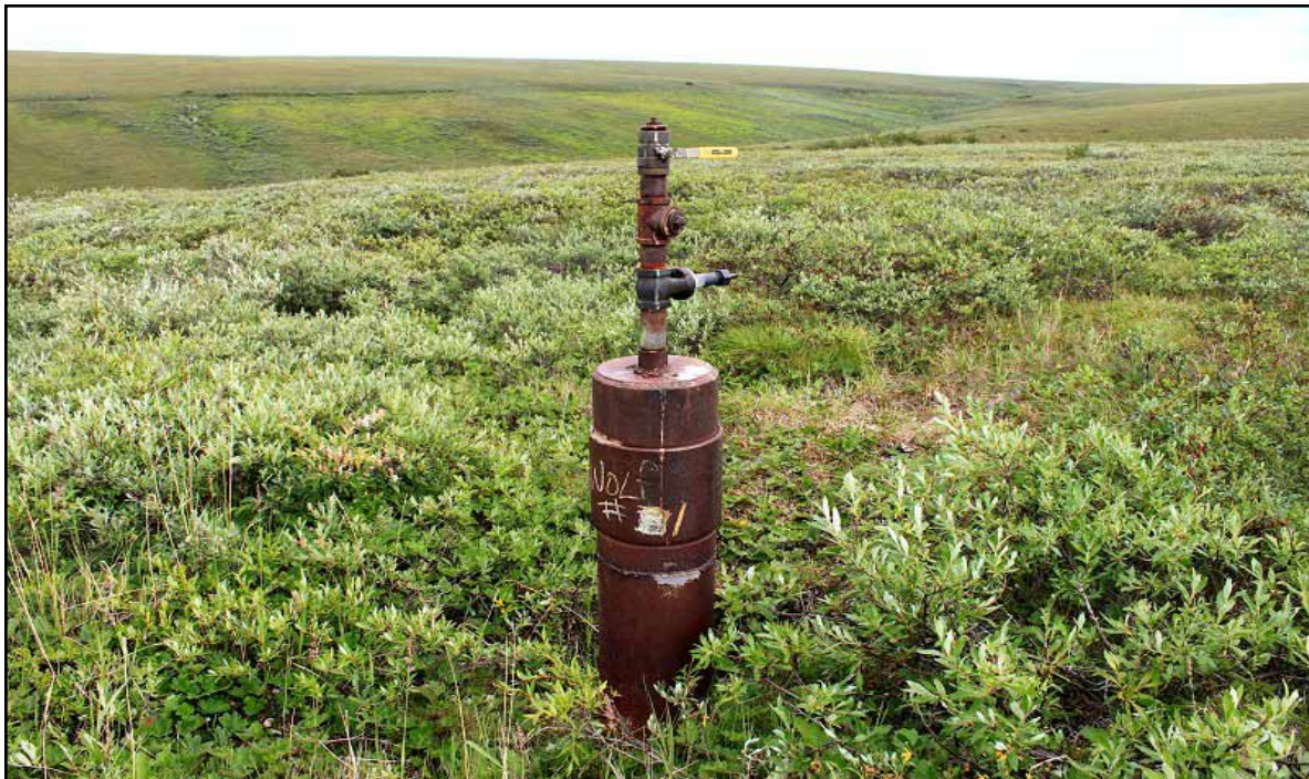
Figure 2: Wolf Creek #1 (July 2012) - The valve is closed and the J-B Weld is holding and in good condition.
