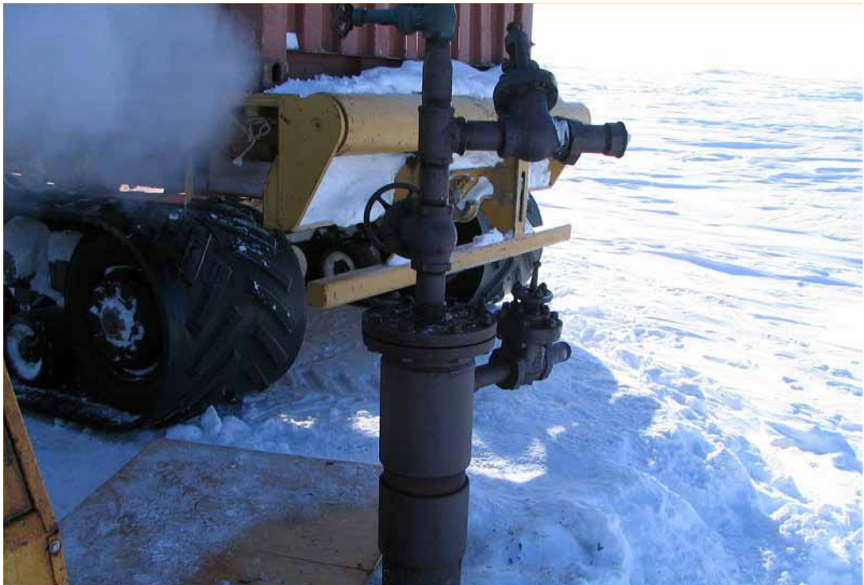
Figure 9: Plugging operations Simpson Core Test #26 (April 2006).
