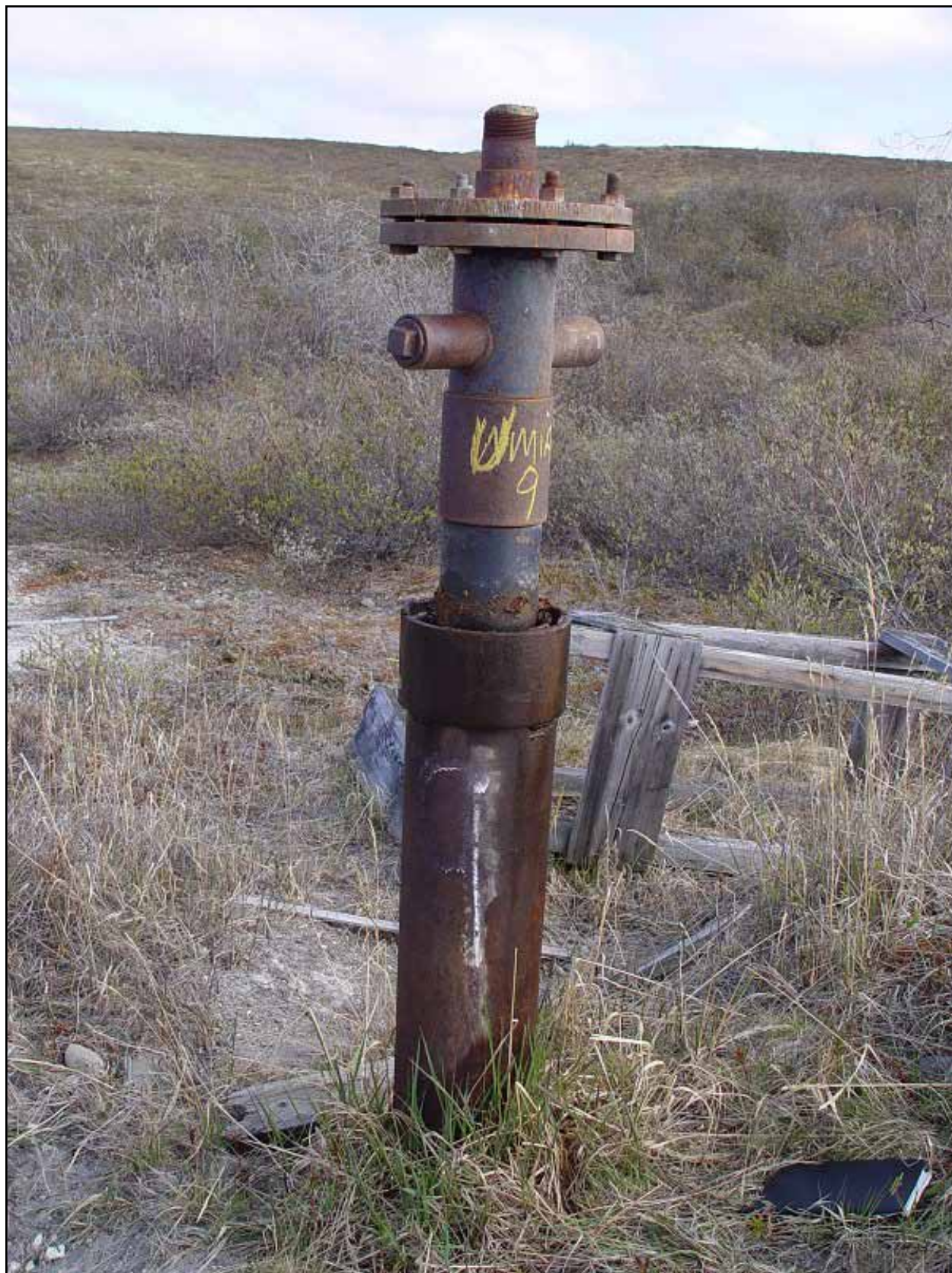
Figure 1: Umiat #9 prior to any remediation work or plugging operations (June 2003).
