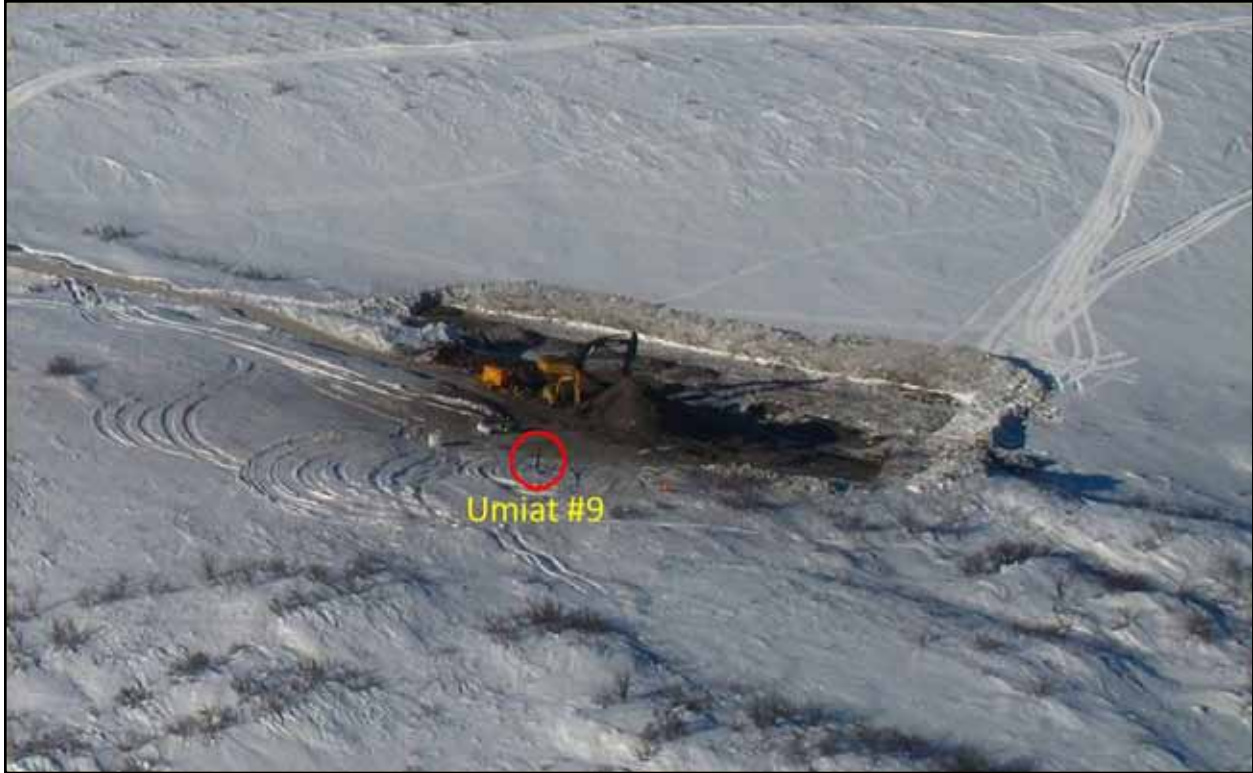
Figure 2: USACE conducting winter cleanup operations at Umiat #9 (March 2011).
