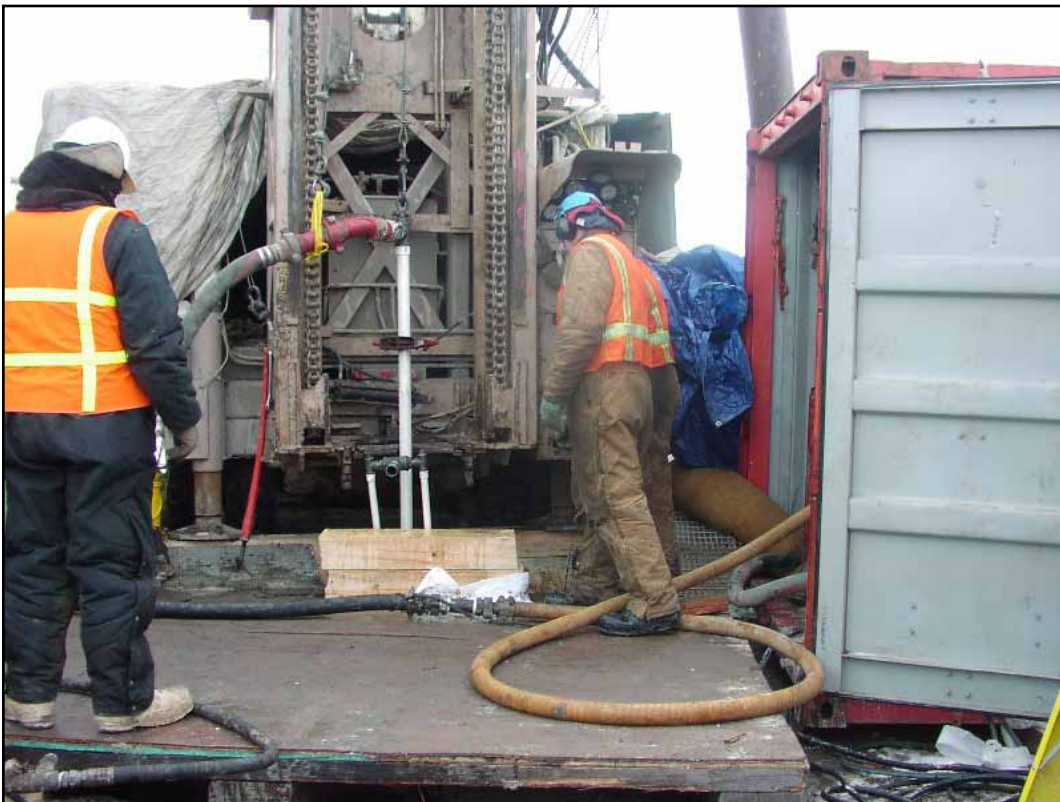
Figure 8: Plugging operations at Umiat #2 (April 2002).
