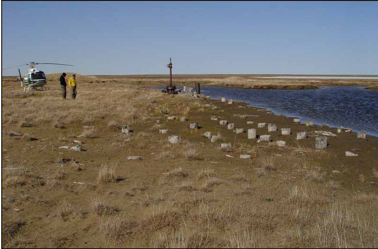
Figure 8: South Meade #1 wellhead and pilings (June 2003).
