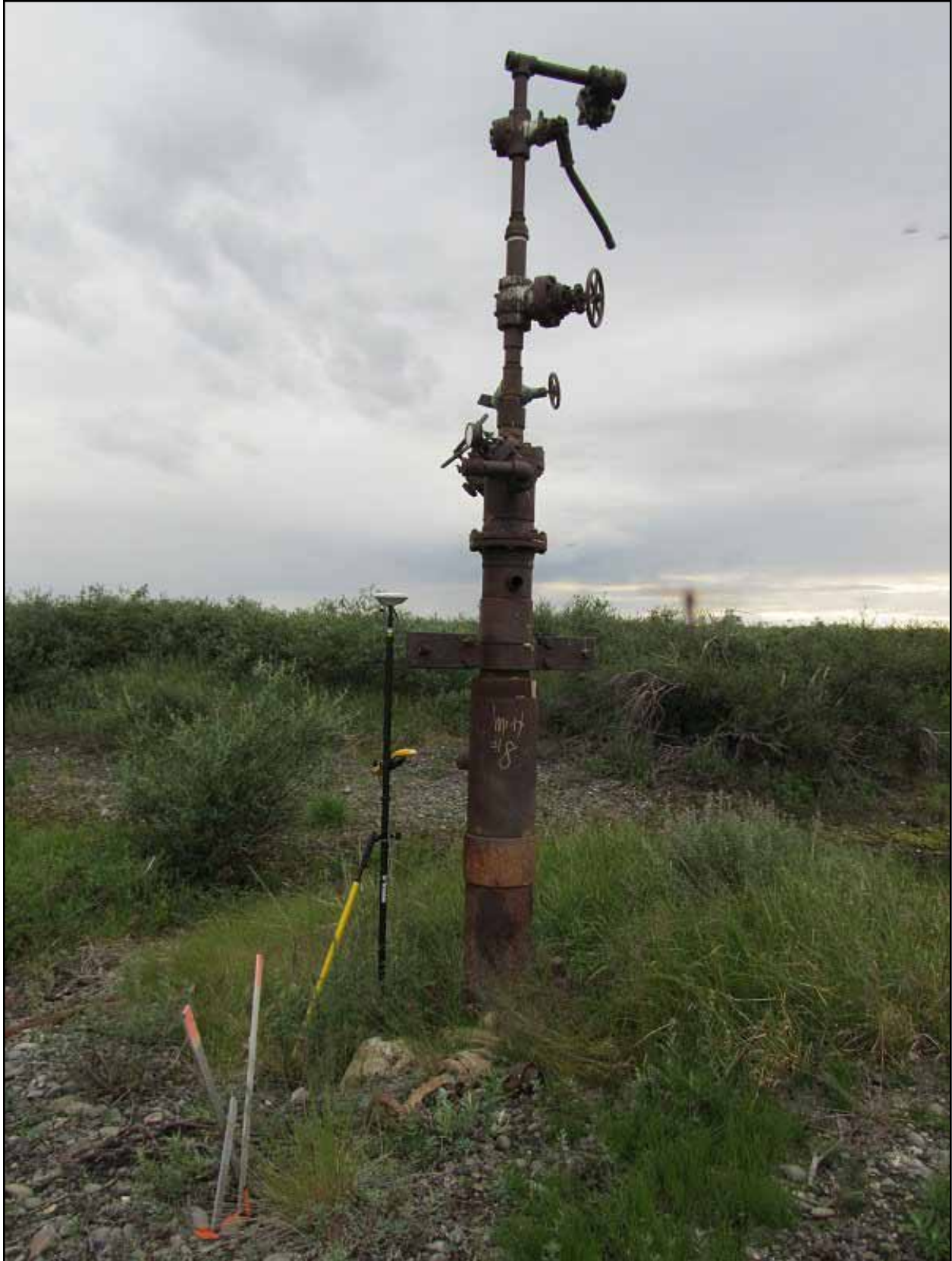
Figure 10: Umiat #8 wellhead 8 years after plugging occurred in 2004 (July 2012).
