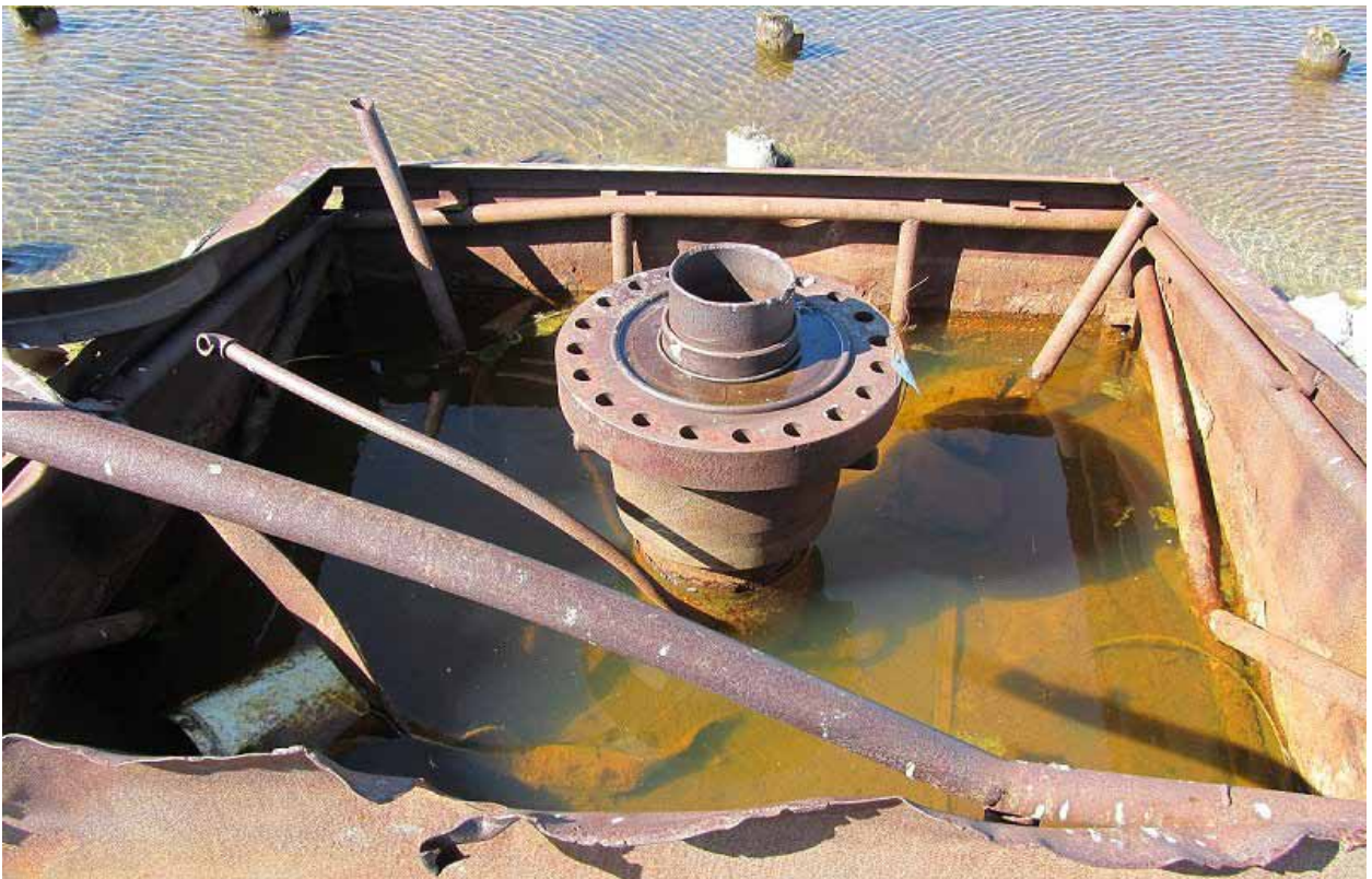
Figure 4: Cape Halkett #1 open casing and metal cellar (July 2010).
