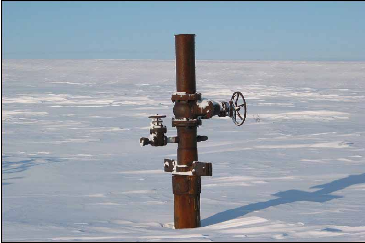
Figure 6: Umiat #10 prior to plugging operations (April 2004).
