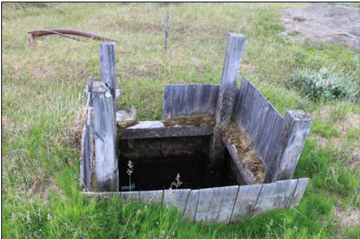
Figure 8: Undocumented cellar and no well pipe apparent at Topagoruk #1.
