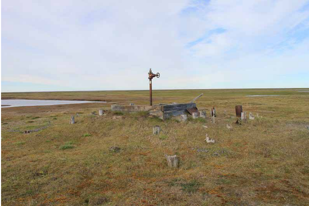
Figure 7: North Kalikpik #1 wellhead with the rat hole outside the cellar and a few wood pilings (July 2012).
