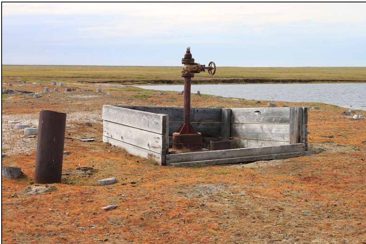
Figure 2: The cellar of Kugrua #1, with one side missing containing the wellhead and mouse hole. The rat hole is outside the cellar (July 2012).
