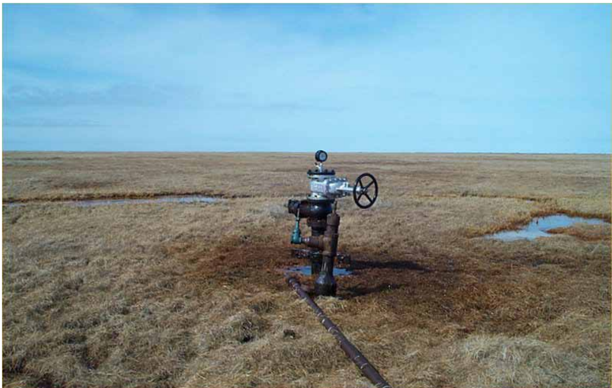
Figure 9: Simpson Core Test #31 replacing old valve (June 2001).
