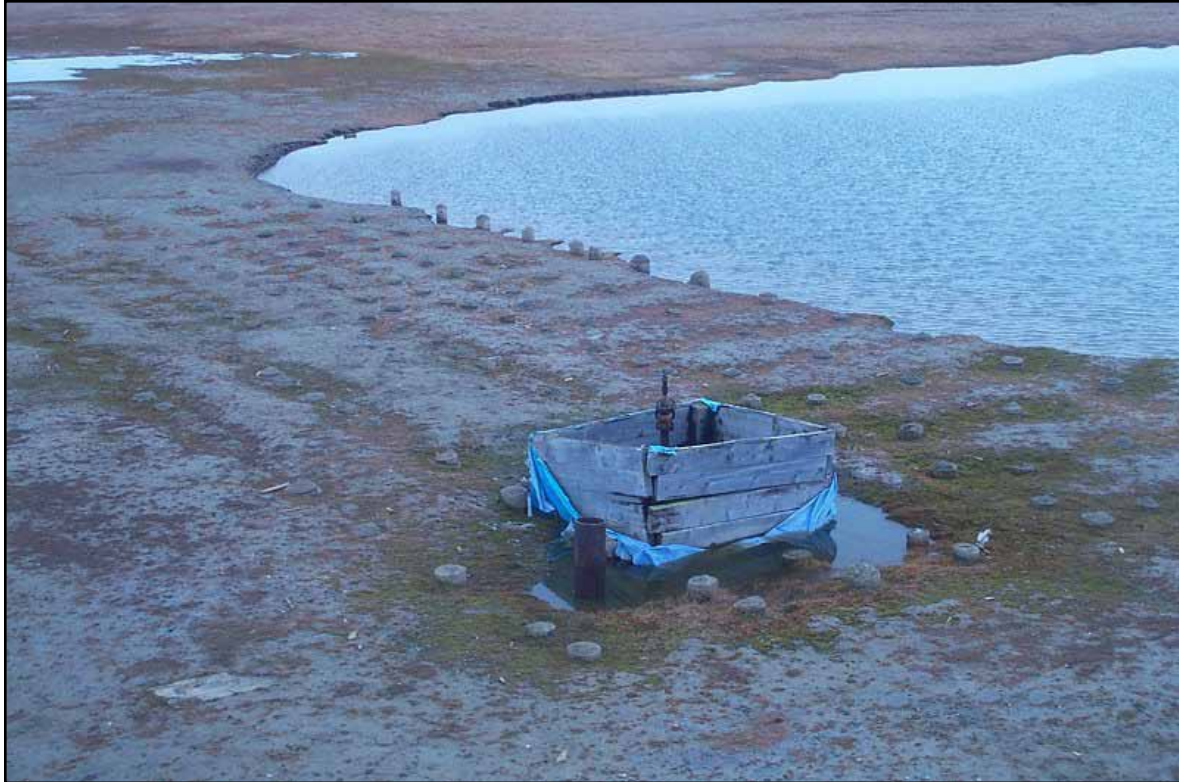
Figure 5: East Simpson #1 in June 2001. The cellar has been thrust by permafrost, but the pilings have not been exposed to the extent they are in 2012.
