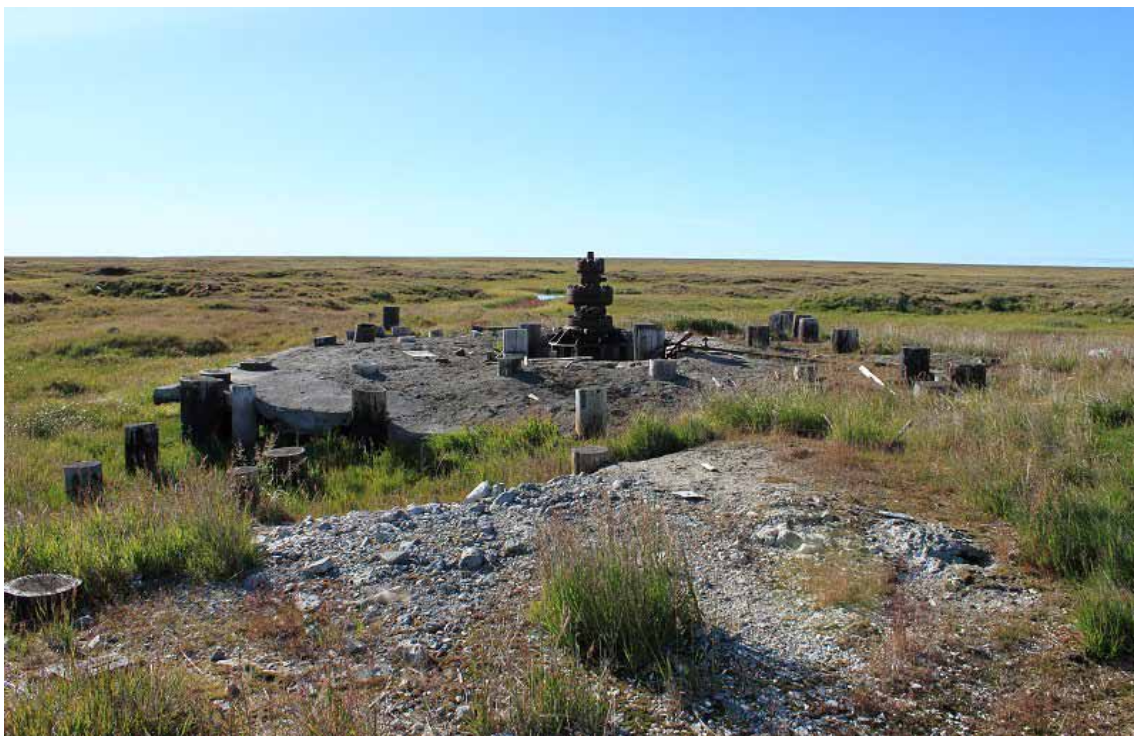
Figure 4: Simpson #1 well with concrete pad and pilings.
