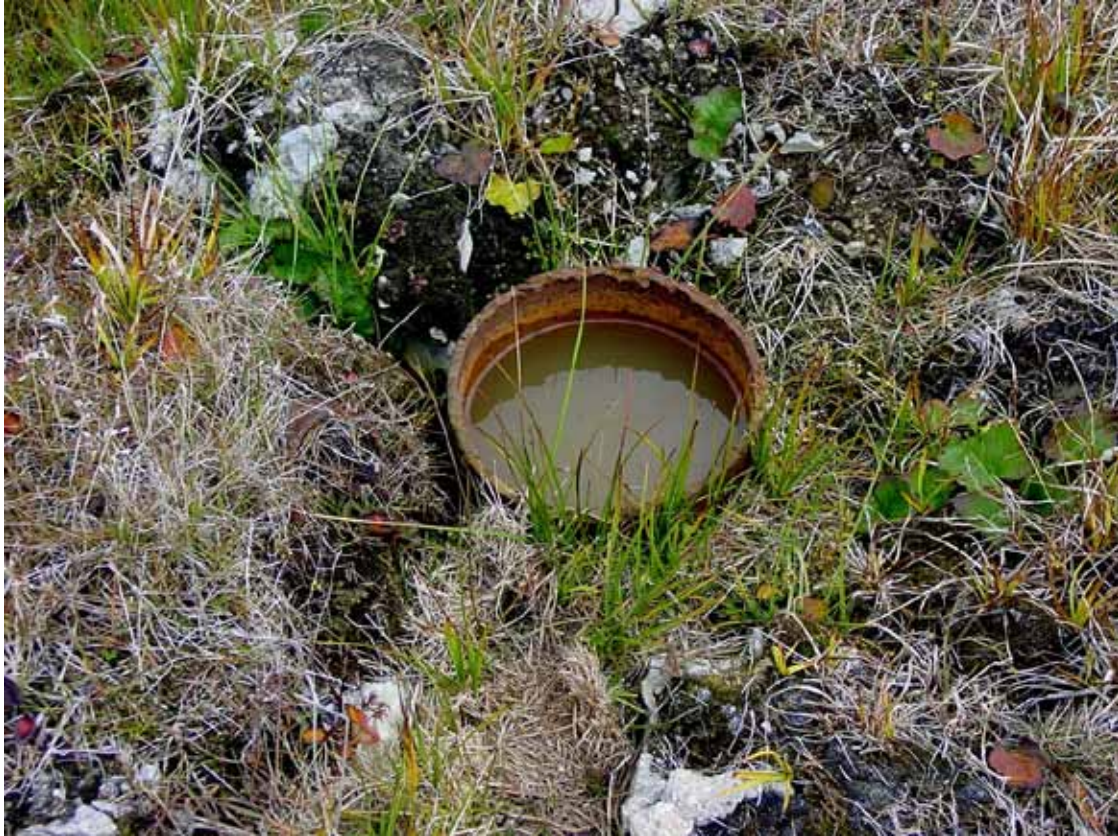
Figure 2: Simpson Core Test #13; note small chunks of concrete.
