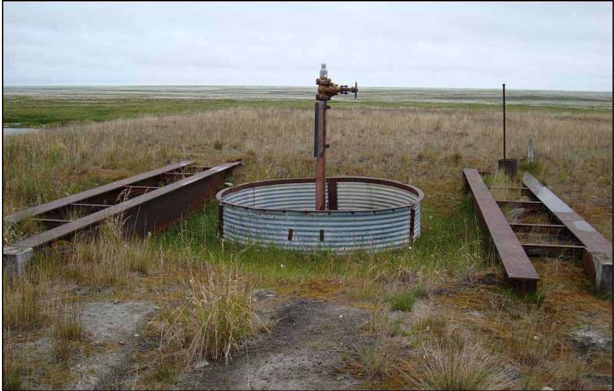
Figure 1: Wellhead with steel beams next to the metal cellar at Tunalik #1 (July 2008).
