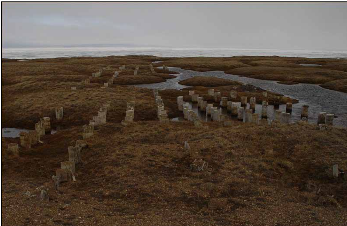
Figure 4: J. W. Dalton #1 pilings extending toward the Beaufort Sea (June 2003).
