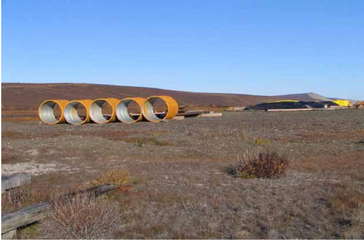
Figure 7: Equipment staged on the Seabee #1 pad (August 2008).
