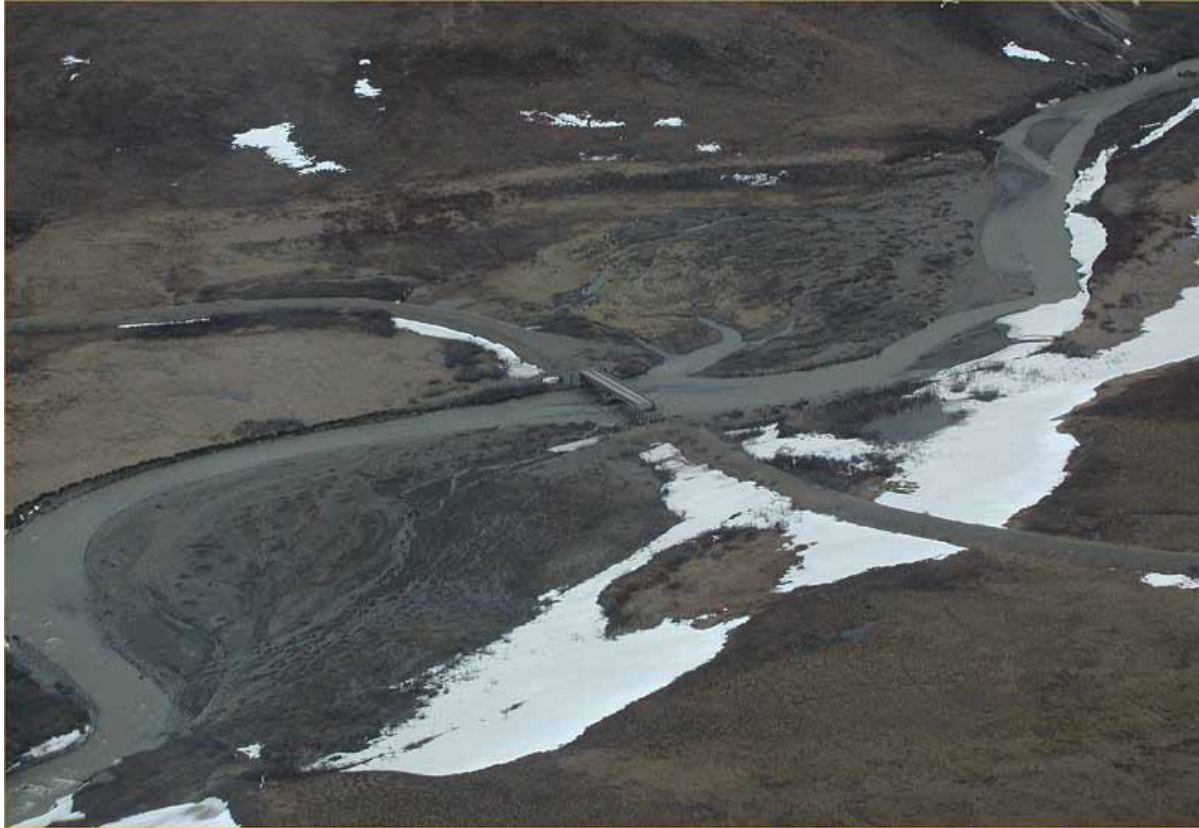
Figure 3: Otuk Creek bridge near Lisburne #1 was no longer usable even on foot from June 2006 to present.
