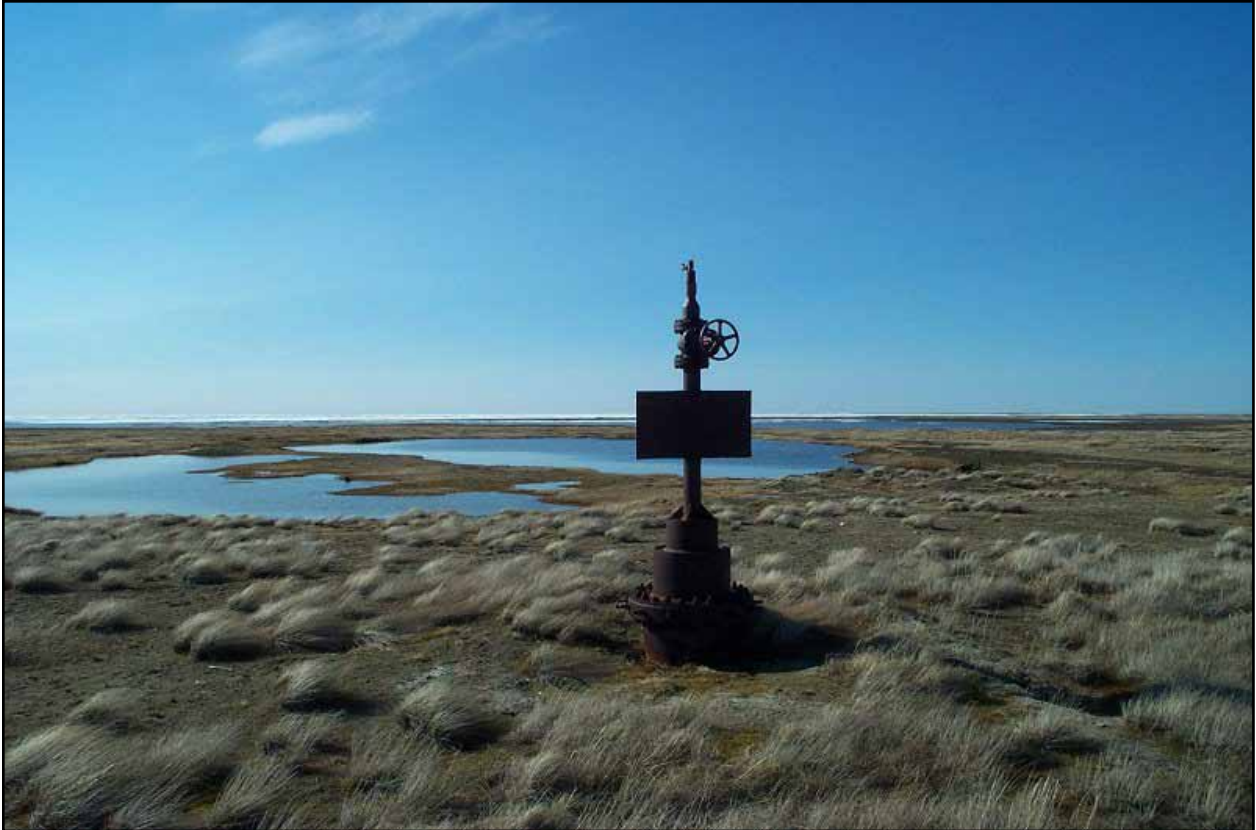
Figure 3: Atigaru Point #1 wellhead and reserve pit (June 2005).
