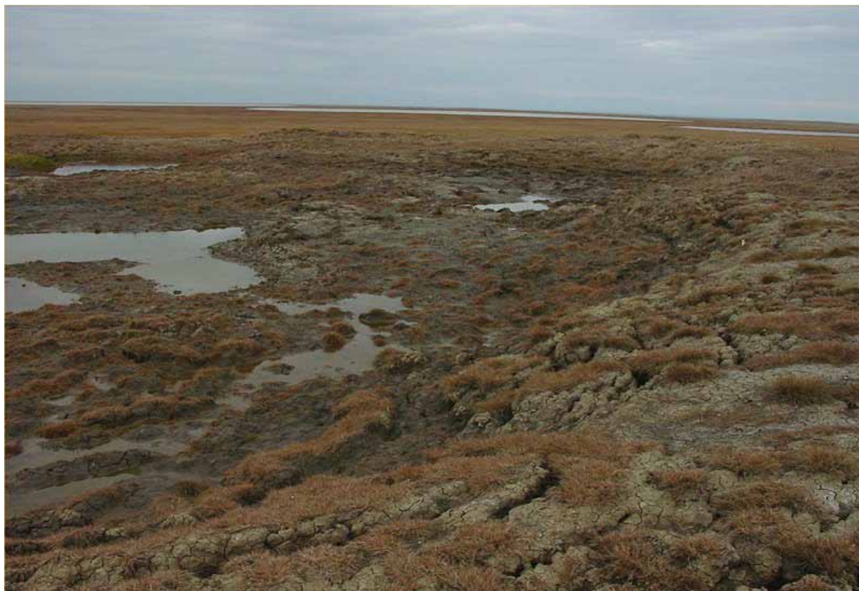
Figure 5: Slumping walls around the depression from the failed drilling operation at Simpson Core Test #16 (August 2002).
