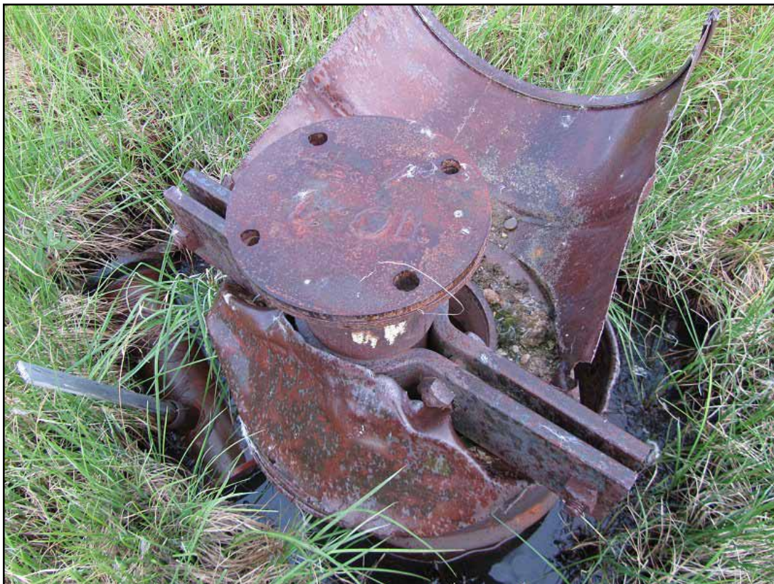
Figure 3: Umiat #7 prior to plugging; the hinged plate cover was installed in April 2004 (July 2010).
