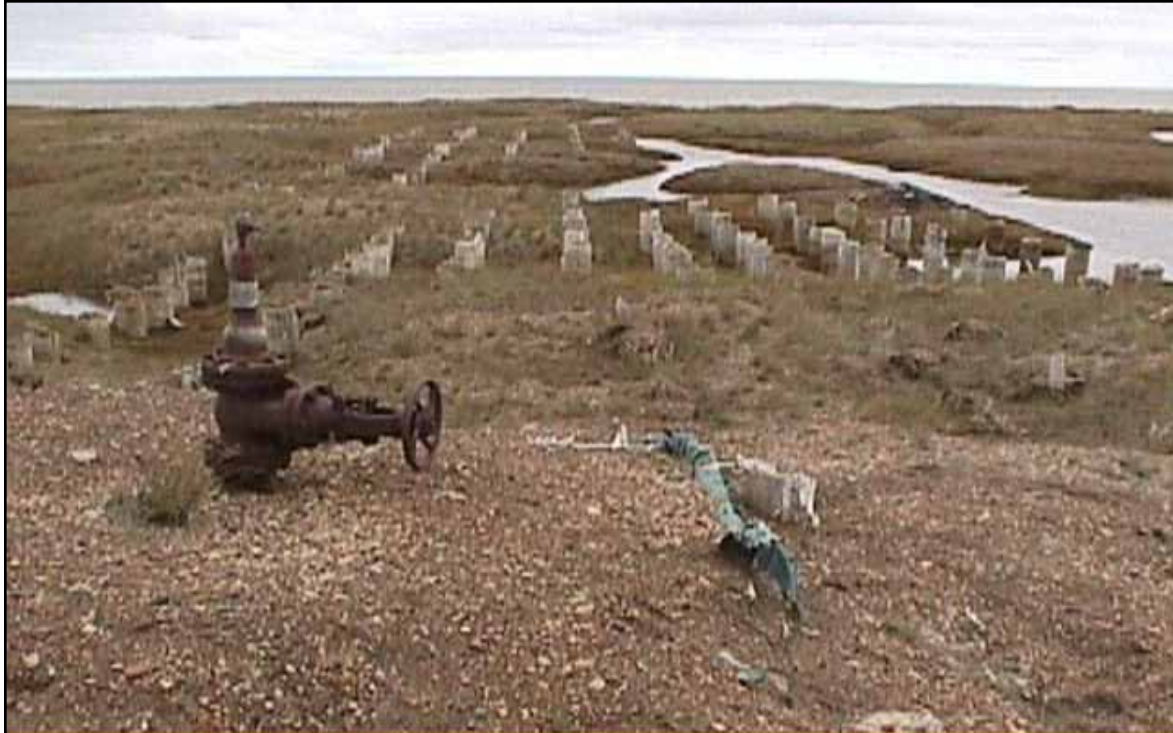
Figure 1: J.W. Dalton #1 wellhead, filled-in cellar, wooden pilings, and Beaufort Sea (August 2000).
