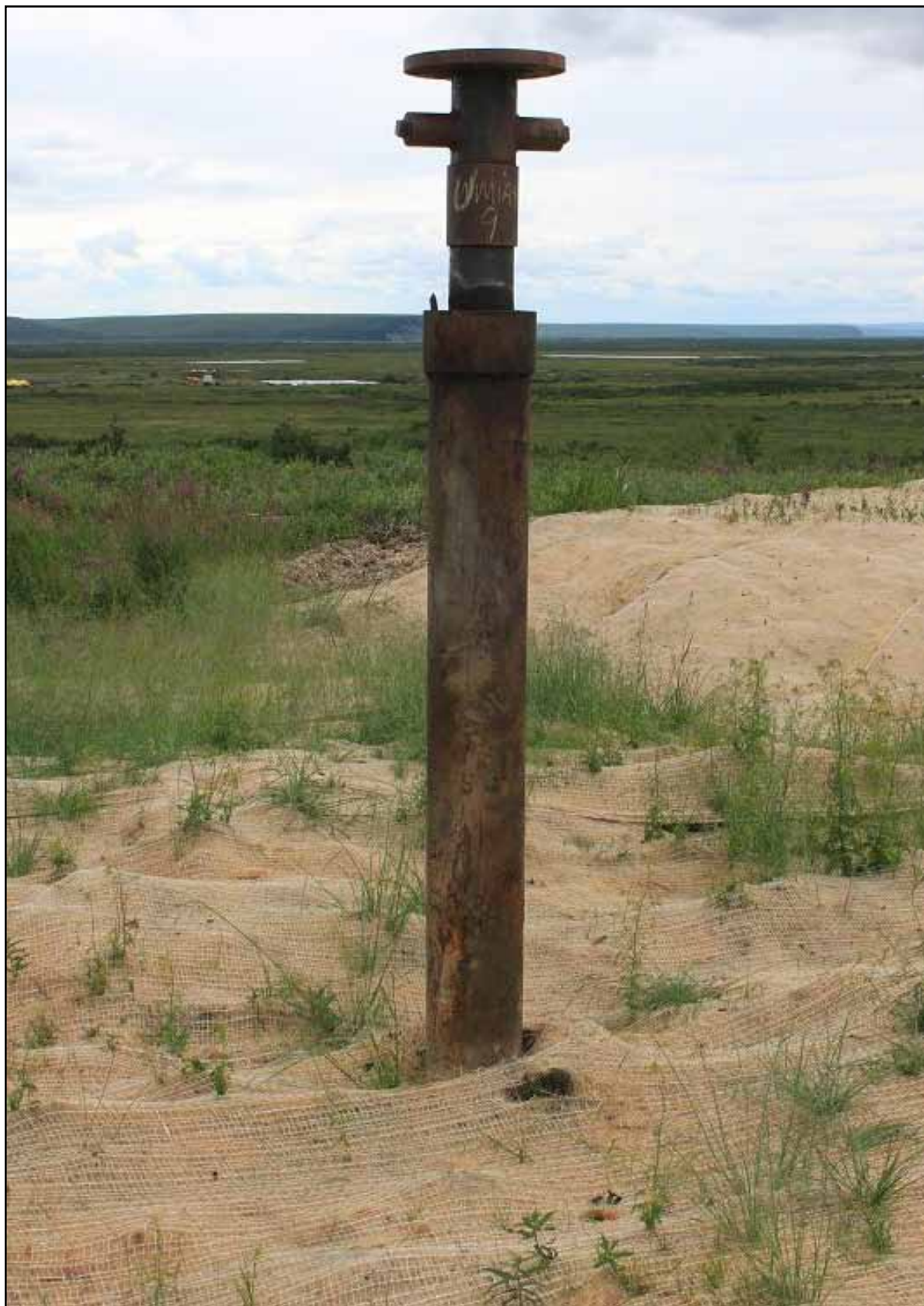
Figure 8: Umiat #9 is plugged and abandoned, with the wellhead left in place (July 2012).
