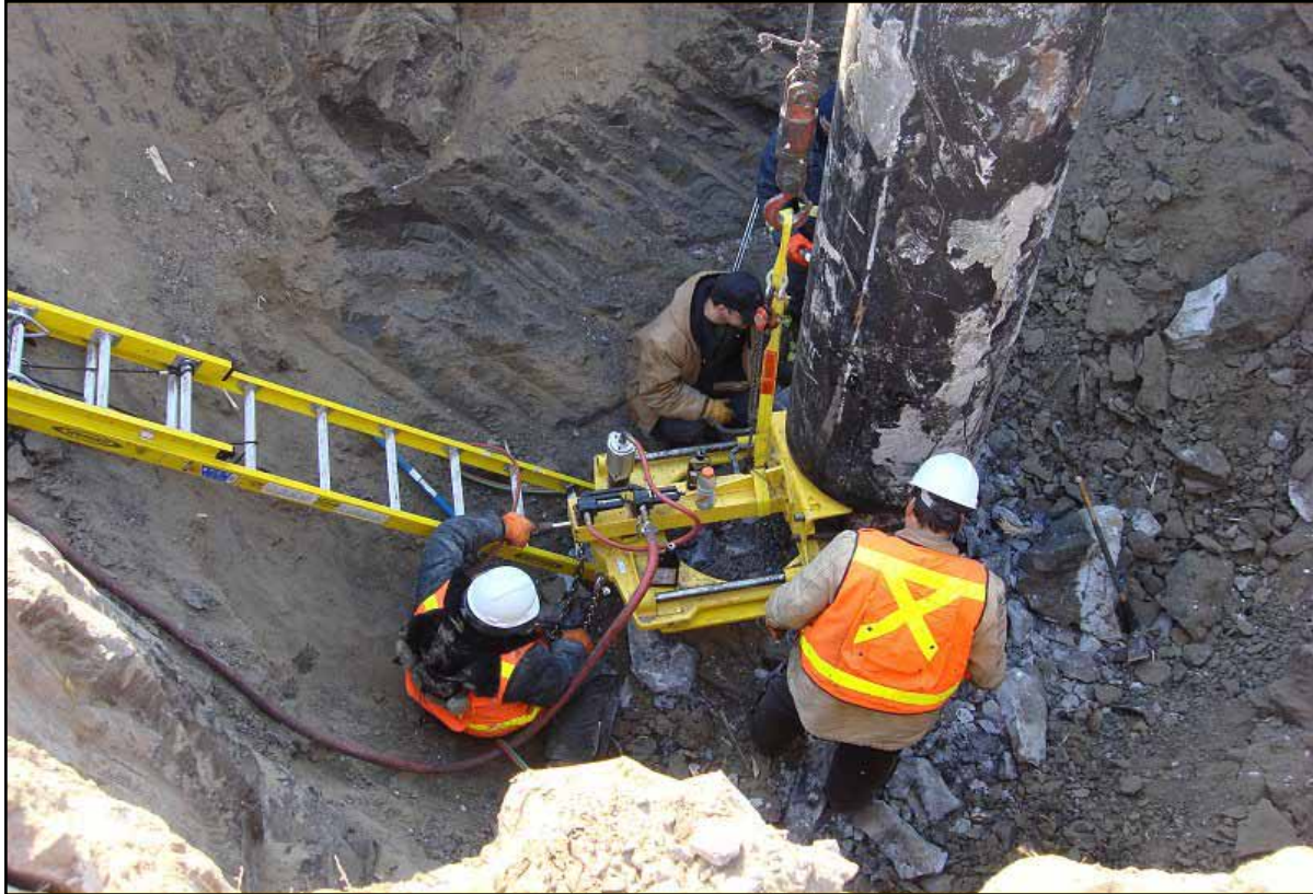
Figure 7: Cutting off the wellhead after plugging the East Teshekpuk #1 well (April 2008).
