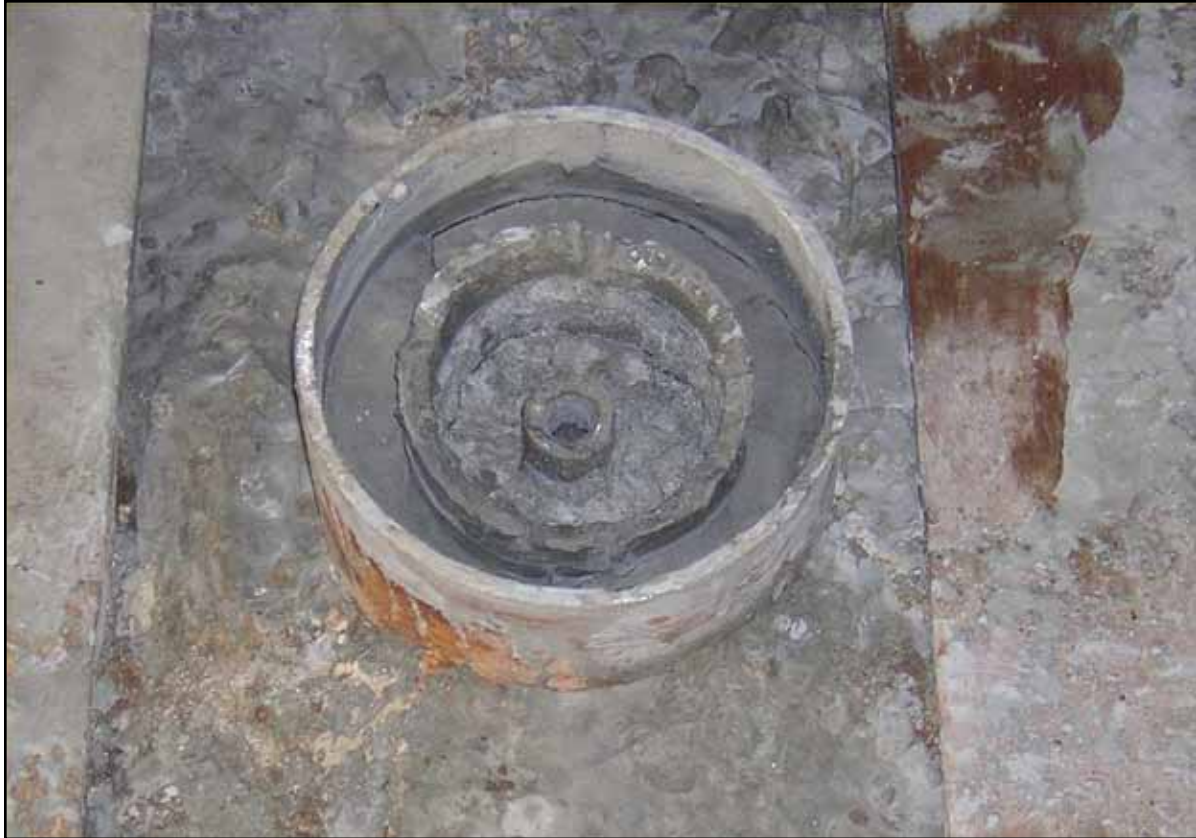
Figure 4: Umiat #9 wellbore cemented prior to welding identification plate (April 2011).
