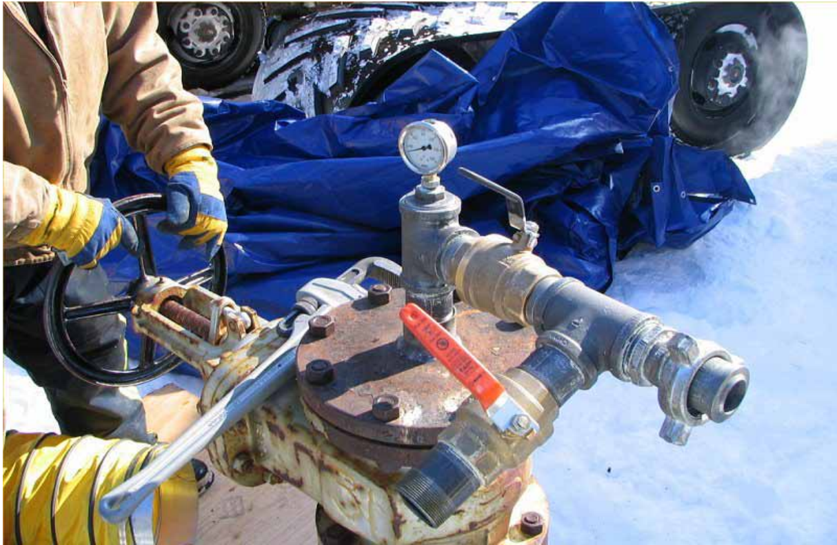
Figure 6: Plugging operations at Simpson Core Test #31 in March 2006.
