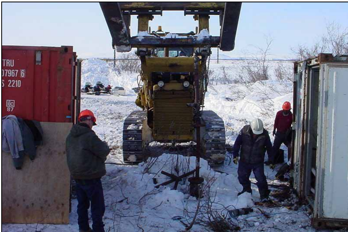
Figure 5: Extracting the wellhead to access the wellbore for plugging operations (April 2004).
