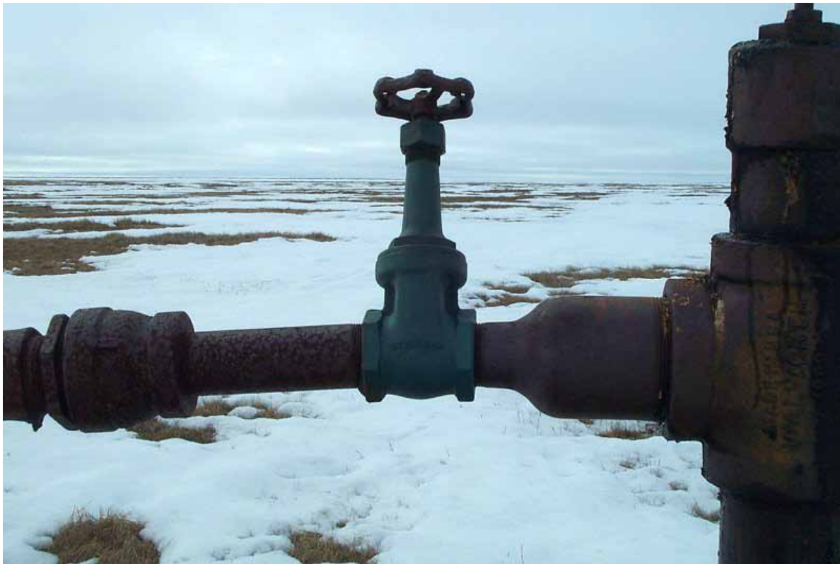
Figure 11: Old valve and arm from Simpson Core Test #31.
