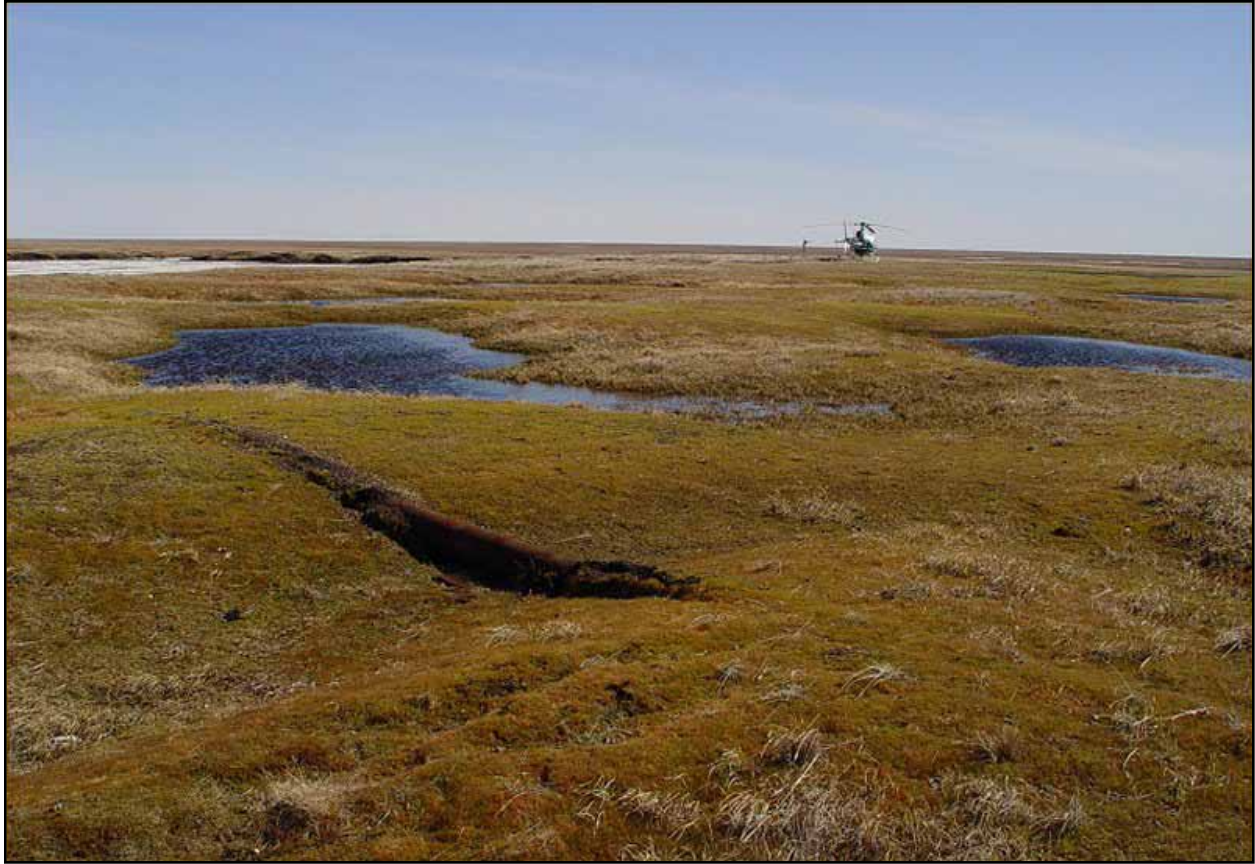
Figure 5: Exposed pipe from subsidence at Tunalik #1 (July 2003).
