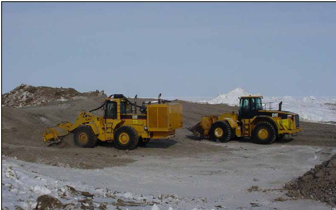
Figure 10: Excavation of the J.W. Dalton #1 reserve pit (April 2005).
