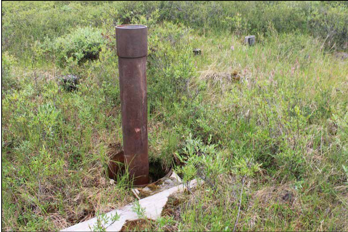
Figure 3: Open casing at Umiat #11; there is no indication of a concrete cellar.
