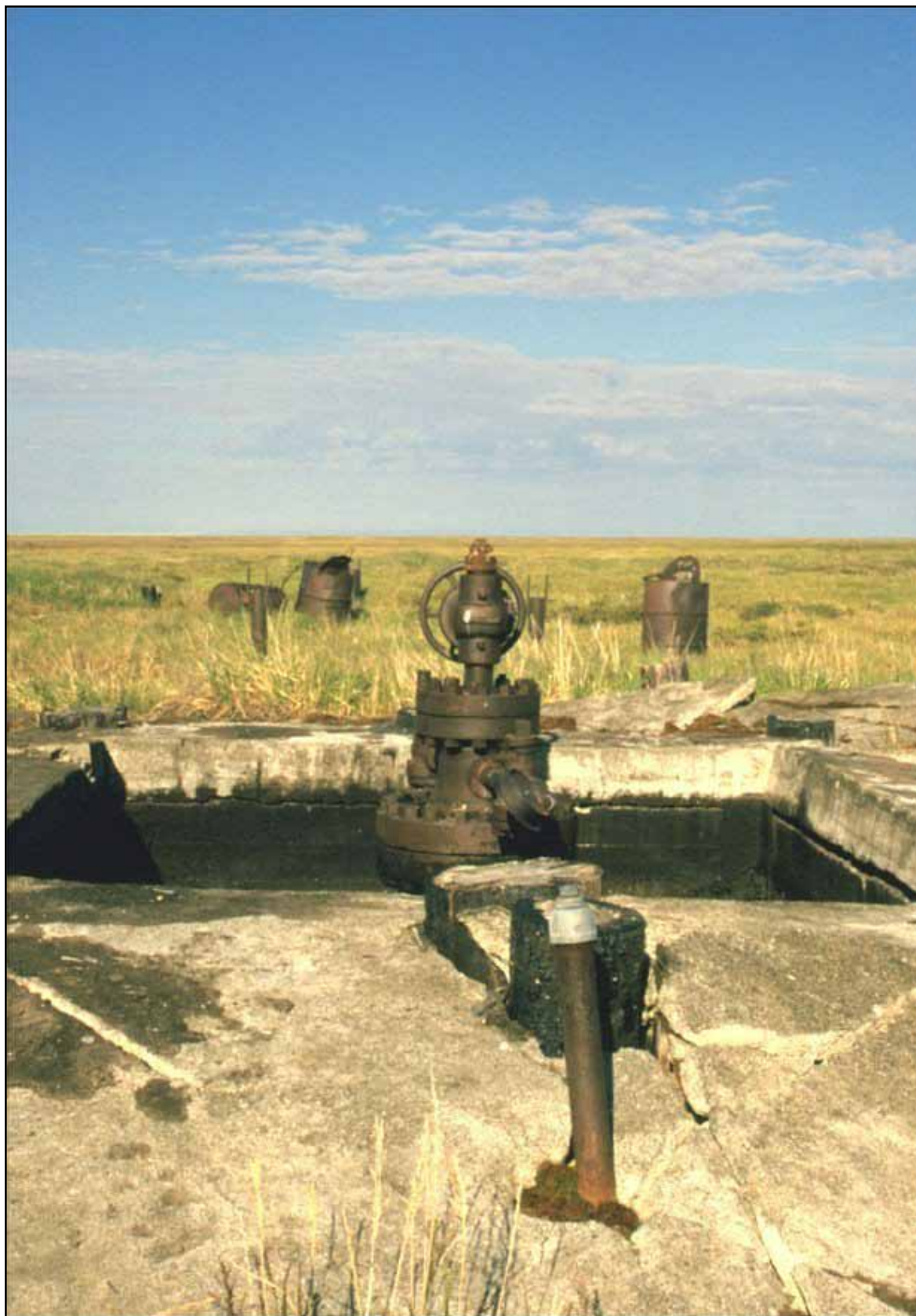
Figure 1: Fish Creek #1 concrete pad and wellhead (July 2002).
