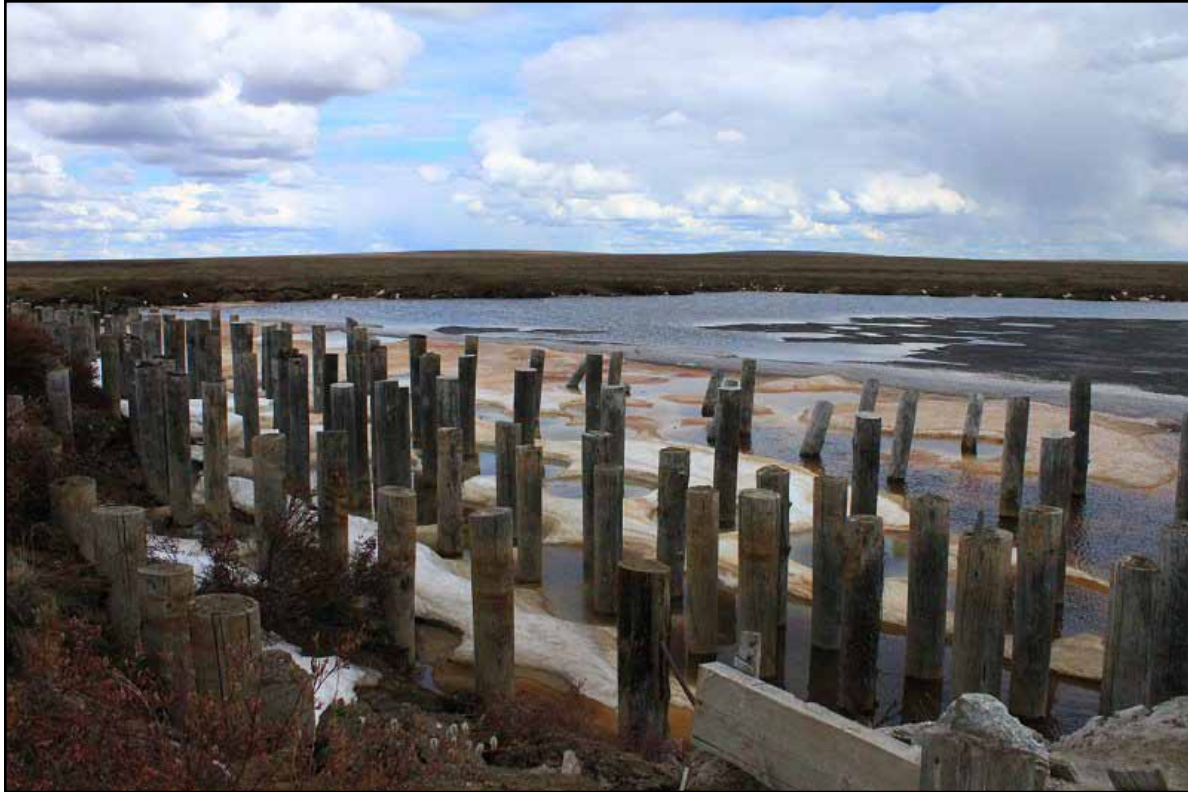
Figure 3: Pilings are now in Awuna #1's reserve pit (June 2012).
