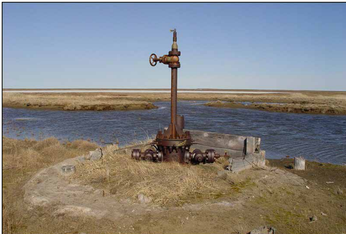
Figure 6: South Meade #1 wellhead during spring break-up (June 2003).
