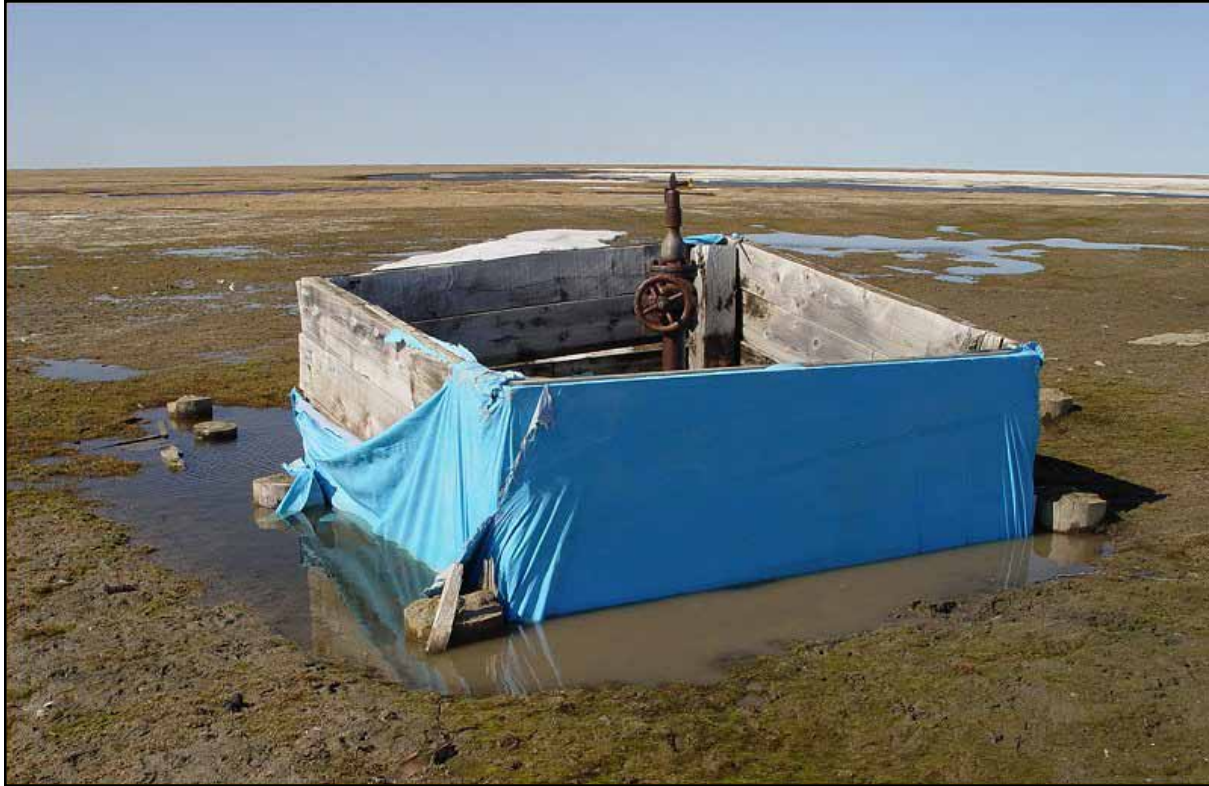
Figure 3: The blue tarp at East Simpson #1 was partially intact in this photo dated June 2003.
