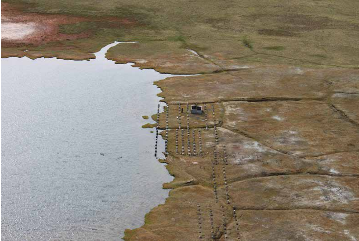
Figure 5: Pilings sticking out into the Peard #1 reserve pit (July 2012).
