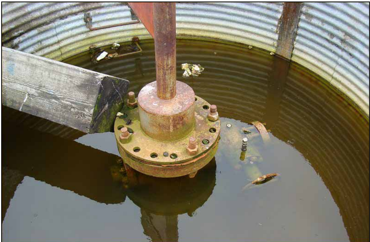
Figure 2: Standing water inside the Tunalik #1 cellar (July 2008).
