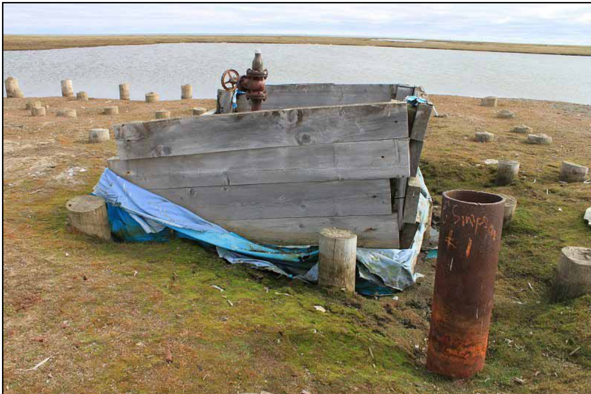
Figure 2: The cellar for East Simpson #1 has been thrust out of the ground due to permafrost action on the south side. The rat hole is outside of the cellar (July 2012).
