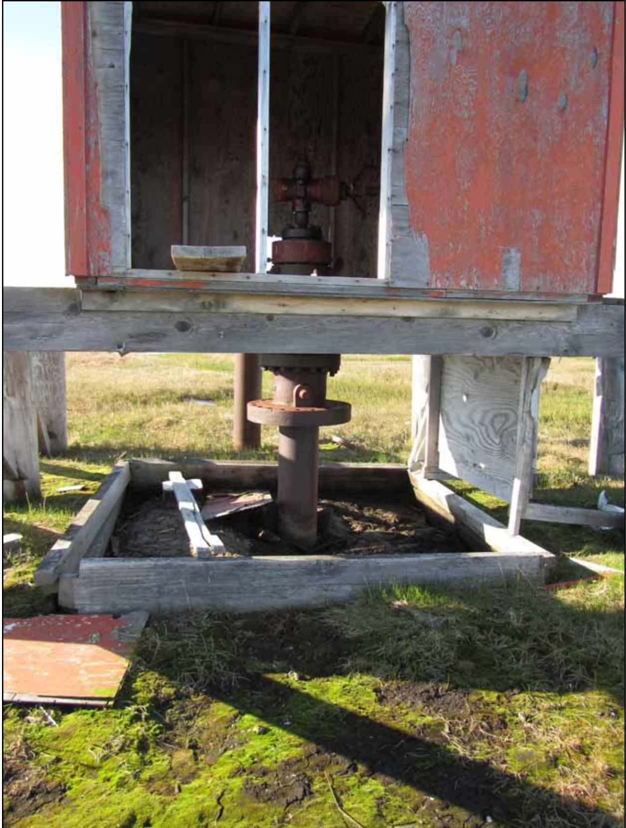
Figure 2: Iko Bay #1 wellhead, frame structure, and cellar.
