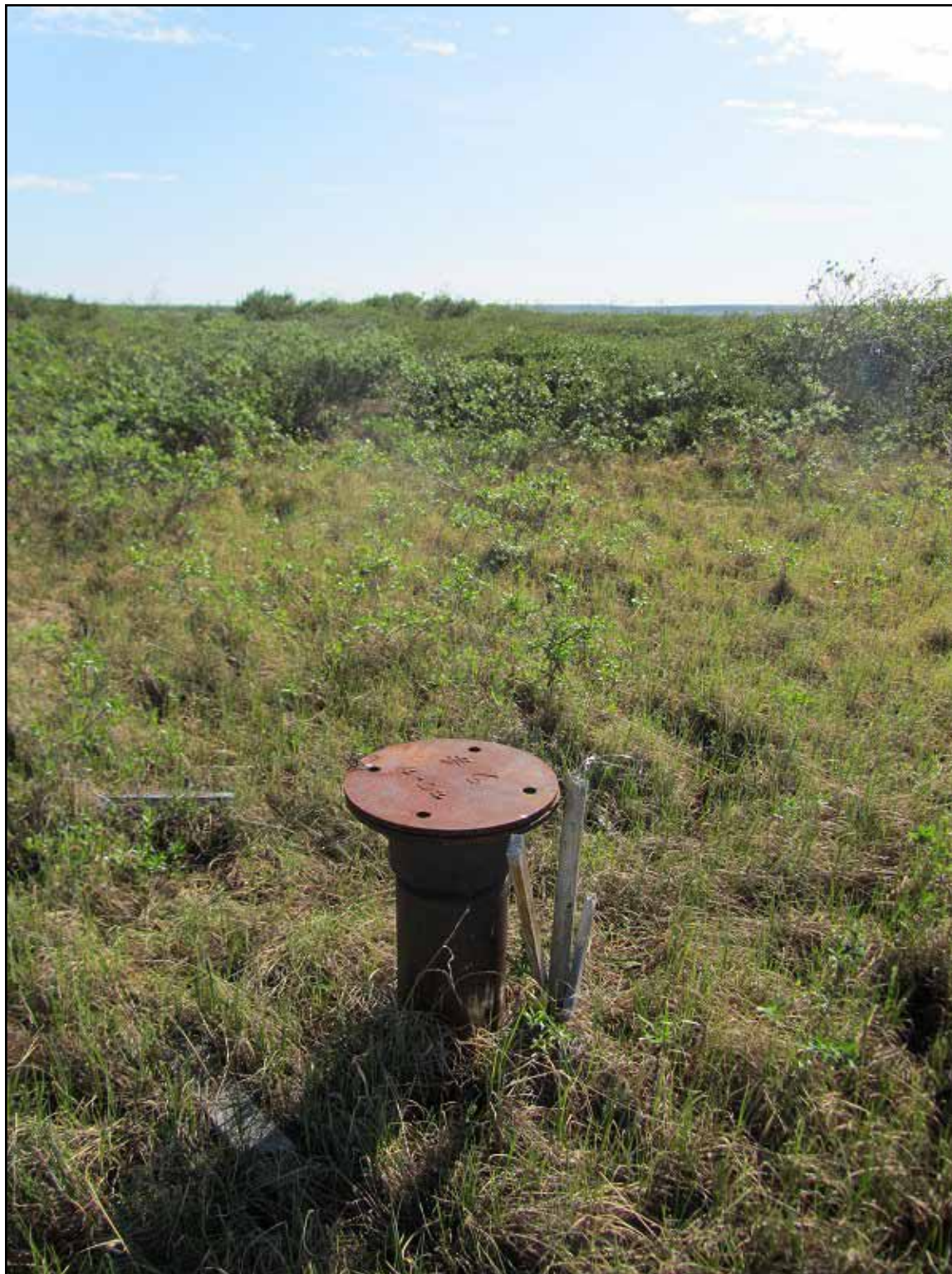
Figure 5: Umiat #6 after installation of the hinged cover plate and prior to plugging in 2012 (June 2011).
