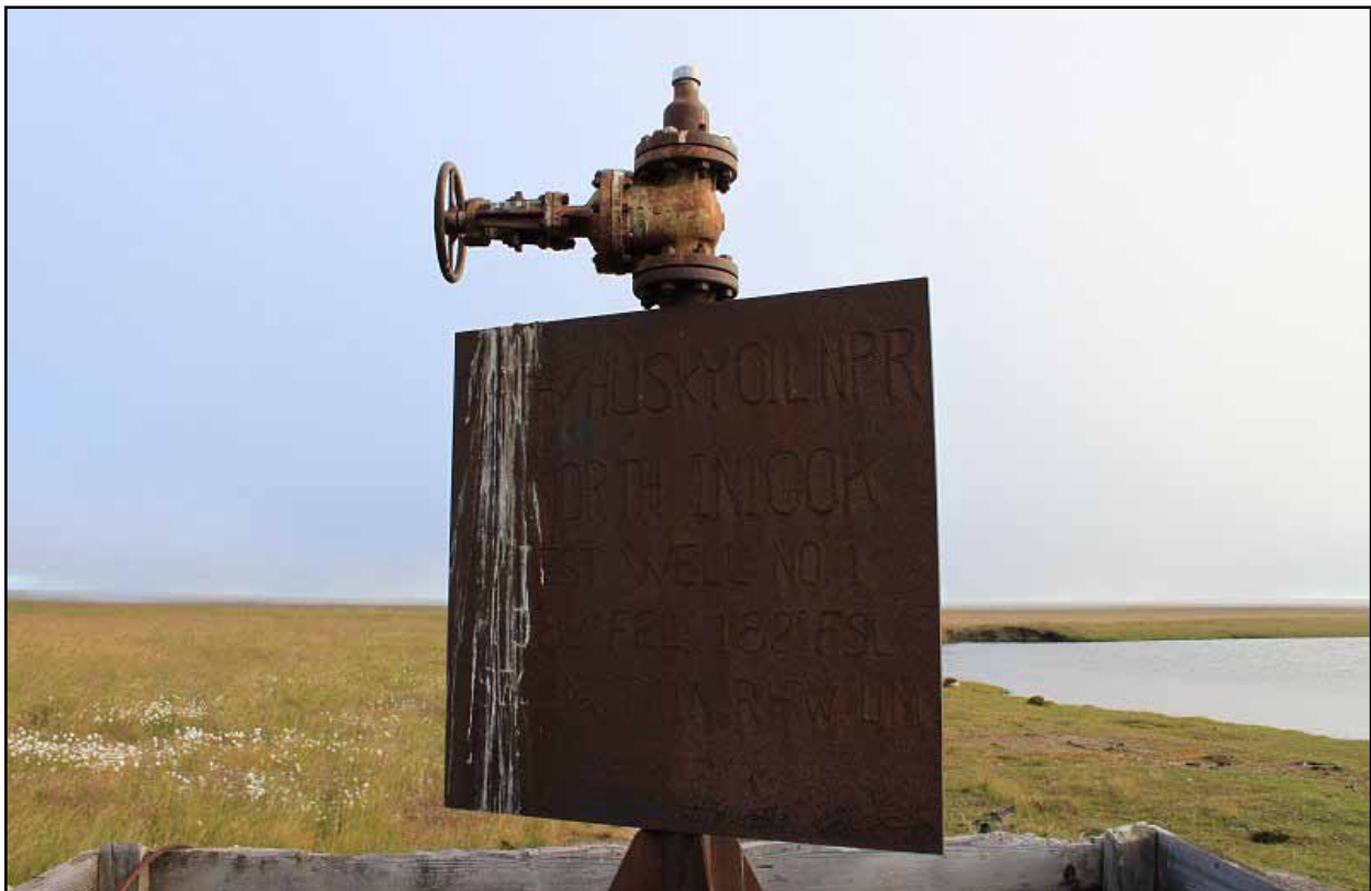
Figure 5: North Inigok #1 4-inch gate valve and cap (August 2010).
