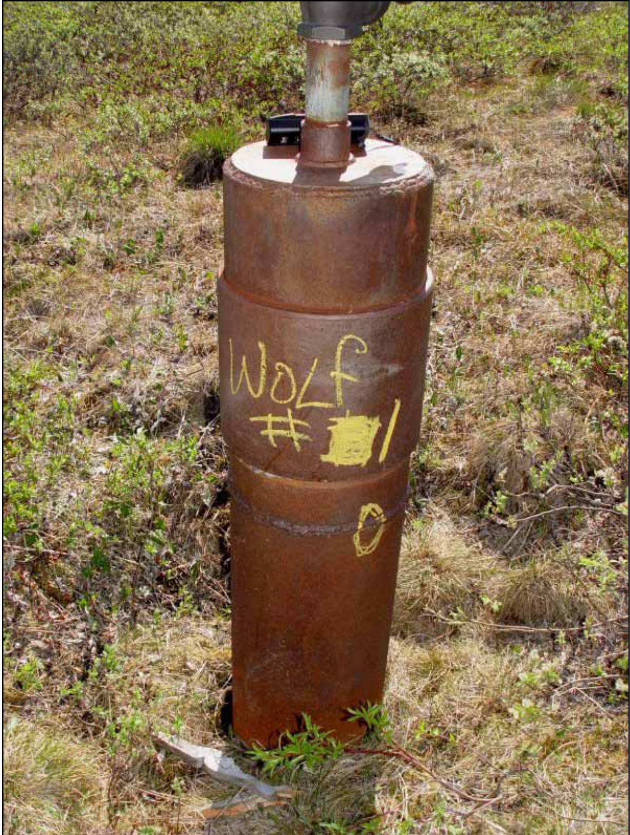
Figure 3: Wolf Creek #1 in 2008 - The circle on the weld identifies where the leak that was repaired in 2004.
