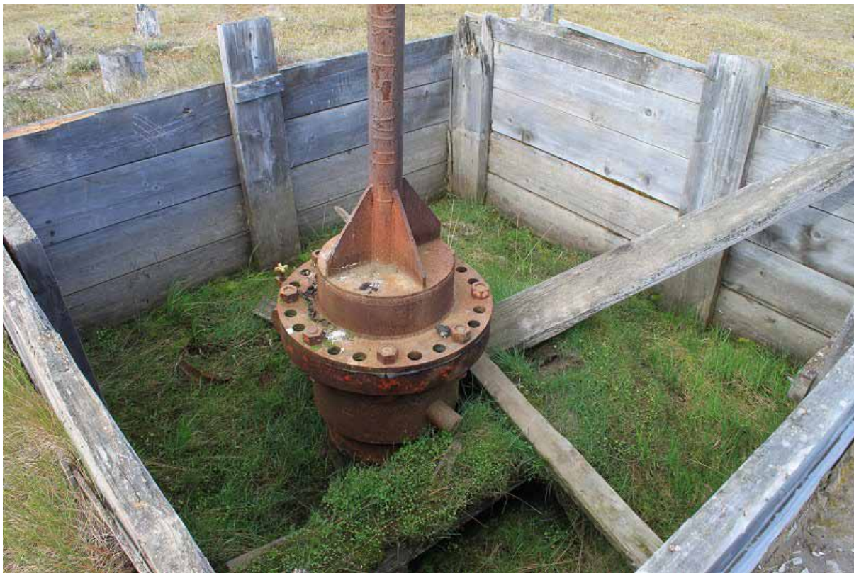
Figure 8: Inside the cellar for North Kalikpik #1 ( July 2012).
