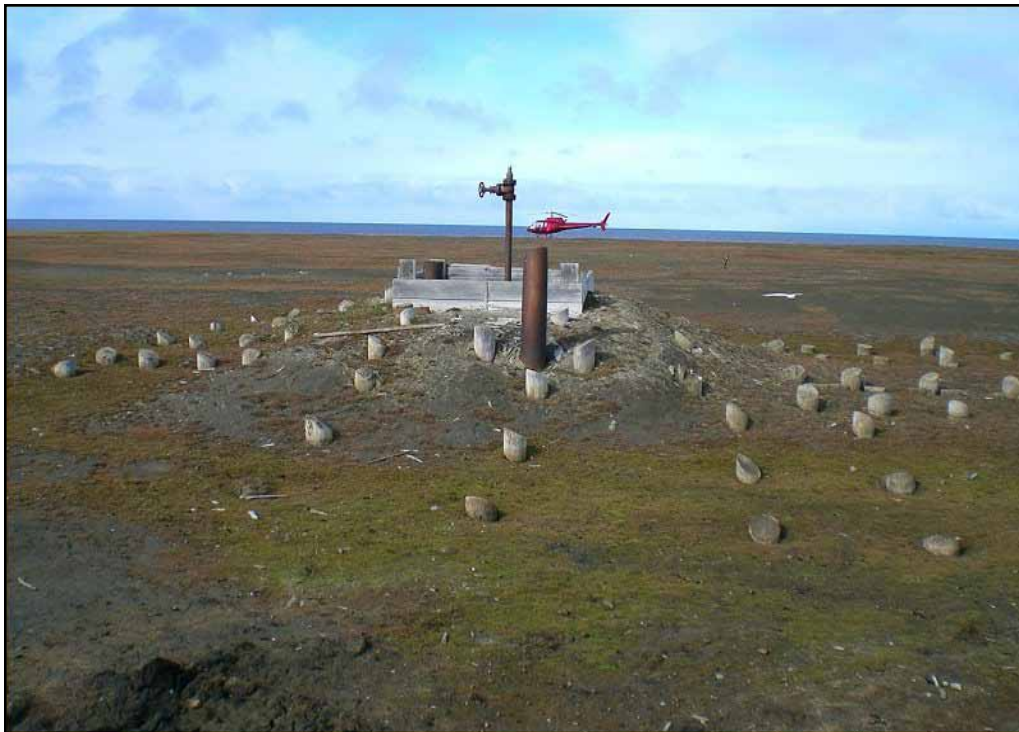
Figure 1: Drew Point #1 wellhead, cellar, pilings, rat hole and drilling pad prior to plugging (August 2006).
