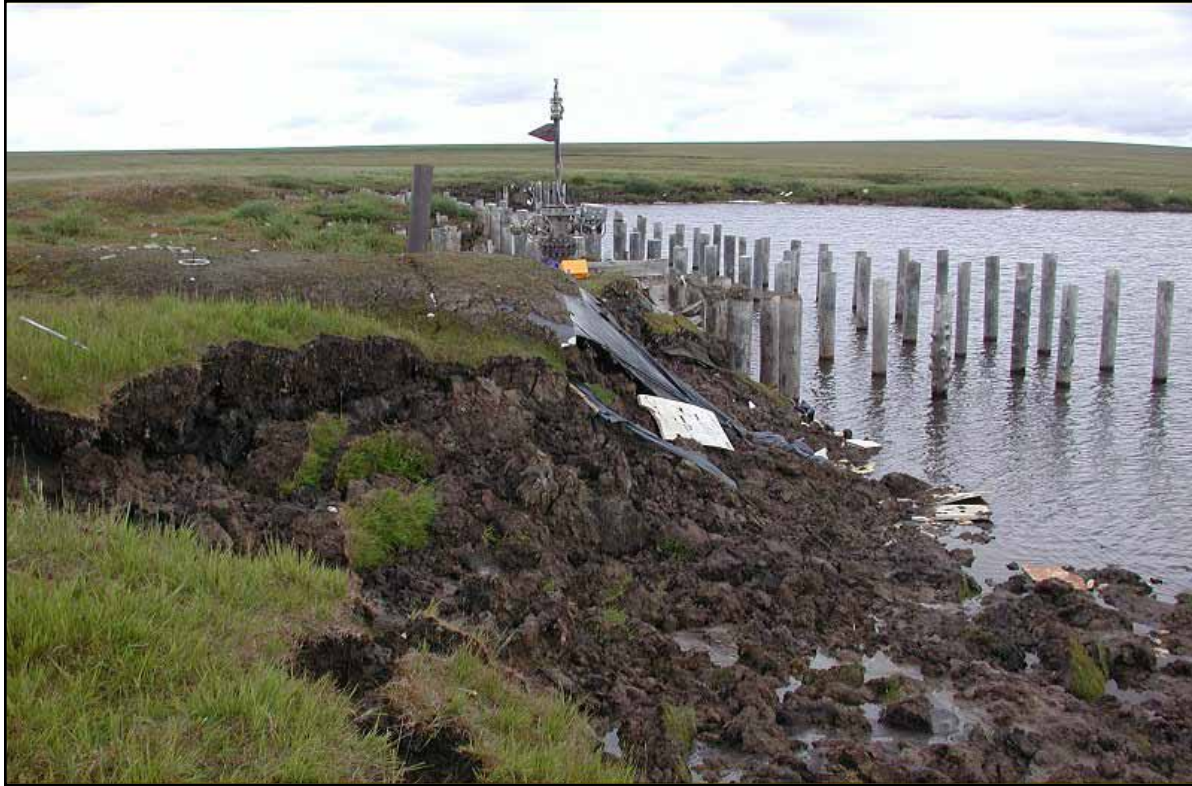
Figure 5: Condition of the Awuna #1 wellhead and pilings in August 2006.
