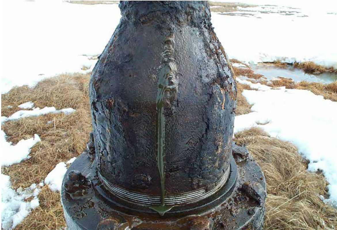
Figure 12: Simpson Core Test #31 leaking oil from the swedge (June 2000).
