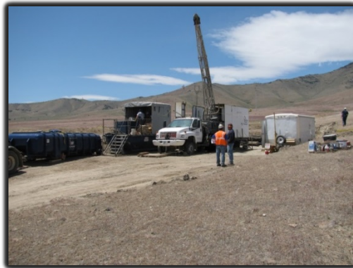
Exploration drilling conducted at Spring Valley
