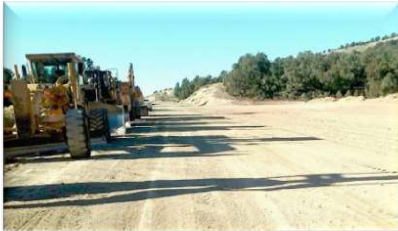
McEwen Mining vehicles line up to be ready for work just before the Record of Decision for the project was signed on November 7, 2017.
