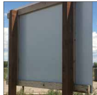
2x4 support structure, nut and bolt sign attachment.
