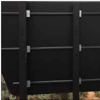
Extrusions attached to back of sign; mounted with angle irons on square posts.
