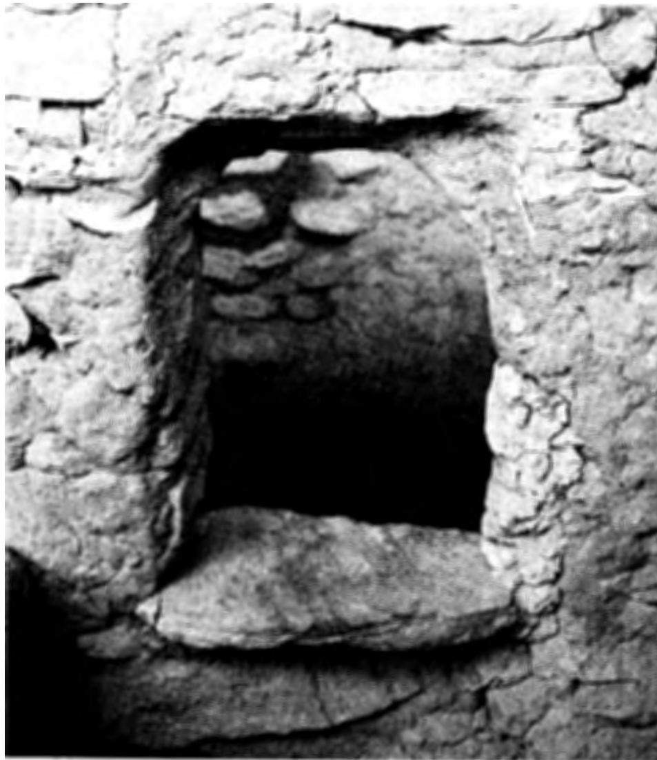
Figure 29 Window Detail in South Wall of Room 7 (from Room 9) (see Figure 24)
