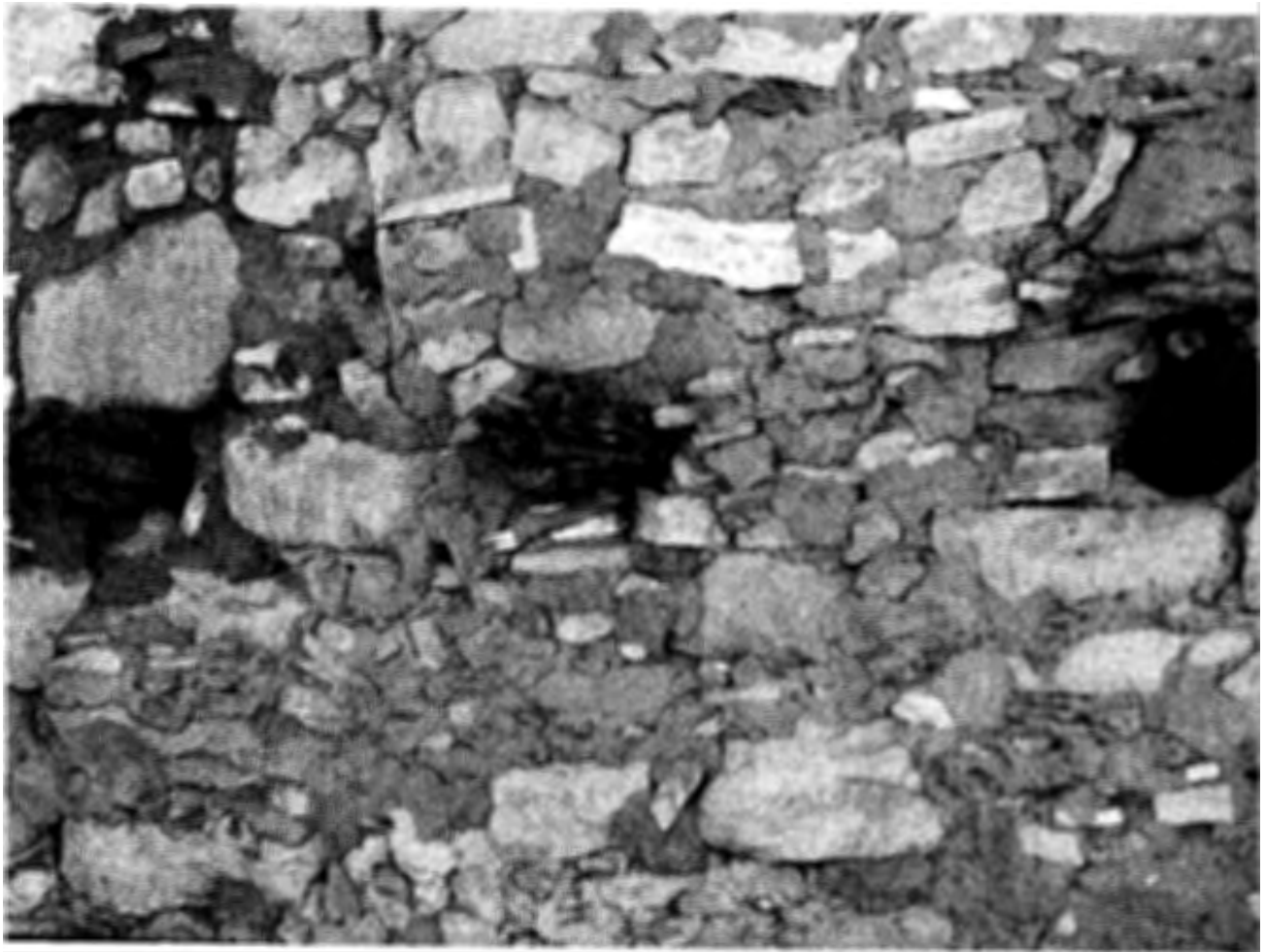
Figure 49 Detail of Late Stage Wall Construction of South Wall of Room 9, Showing Roof Beam Butts
