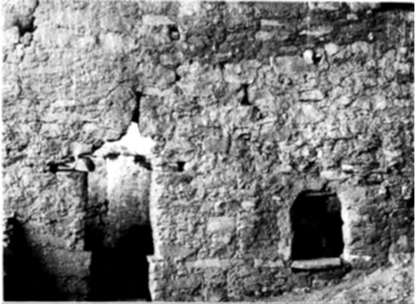
Figure 26 East Wall of Rooms 8 and 9 in Room Block B Showing Intermediate and Late Stage Construction (see Figure 25)
