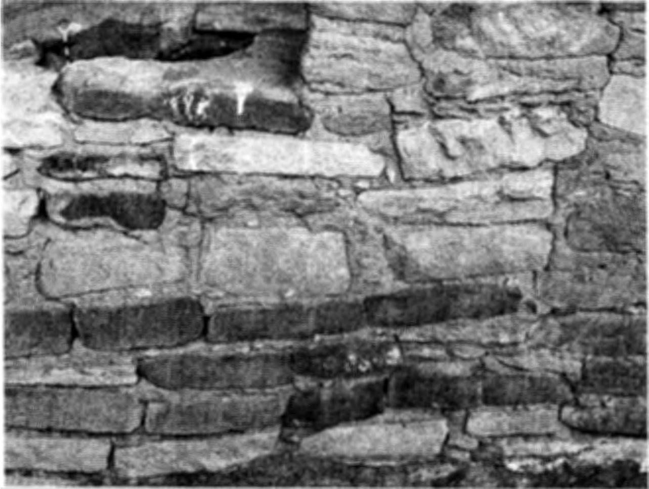
Figure 20 Closeup of the Masonry Construction of the Front Wall of Room 4
