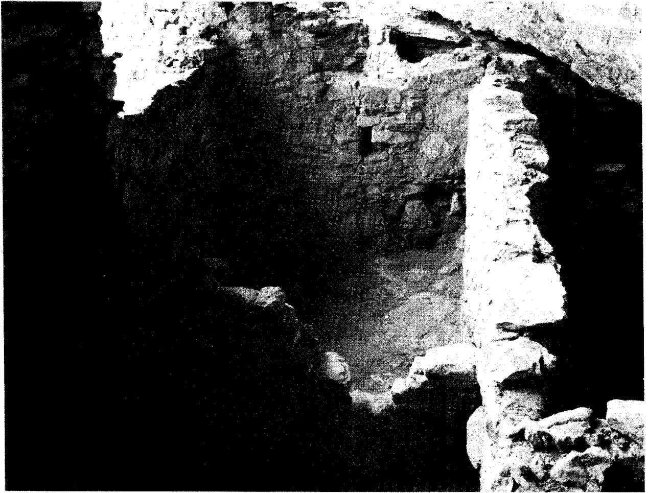
Figure 36 Room 10 Looking West toward Kiva
