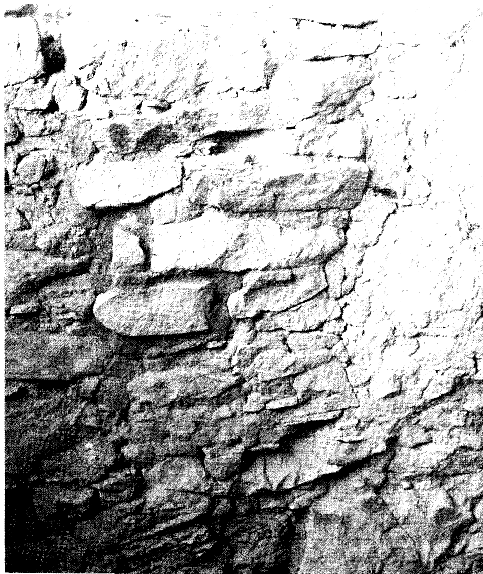
Figure 34 Plugged Entry in West Wall of Room 10
