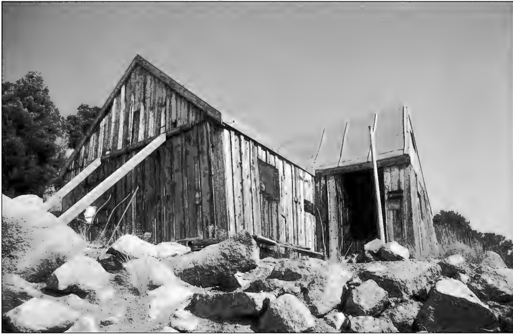
Figure 6.1. “Ridge Cabin,” Beveridge Mining District, Inyo County, after stabilization under the Adopt-A-Cabin in program, 1991 (photograph by Karen K. Swope).
