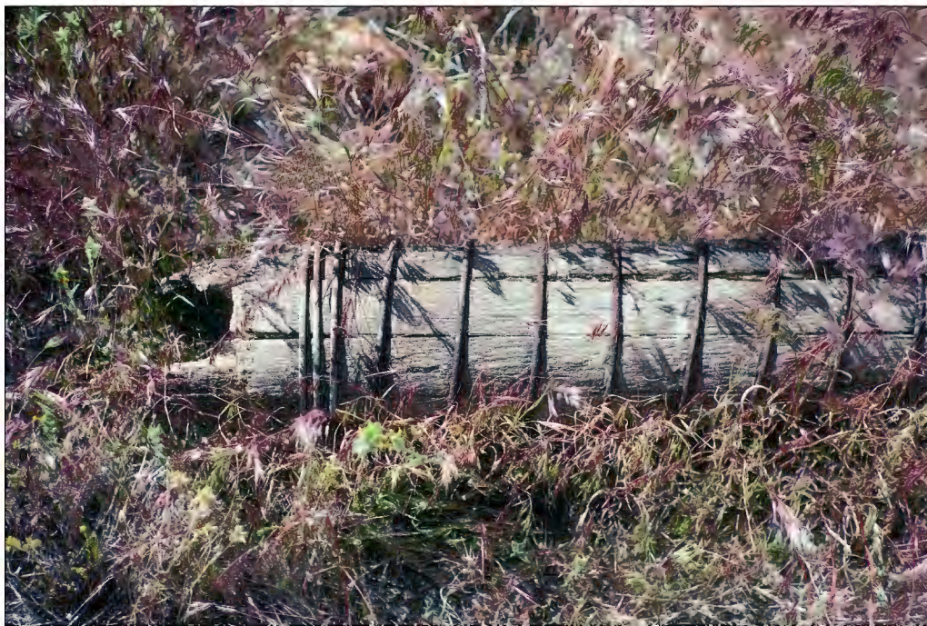
Figure 3.62. Wire-wrapped wooden water pipe, Yellow Aster Mine, Kern County, 1993 (photograph by Karen K. Swope).
