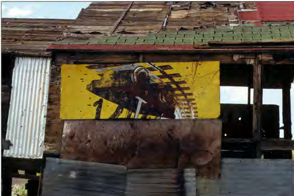
Figure 3.50. Recycled materials used in building construction, Masonic, Mono County, 1992 (photograph by Karen K. Swope).
