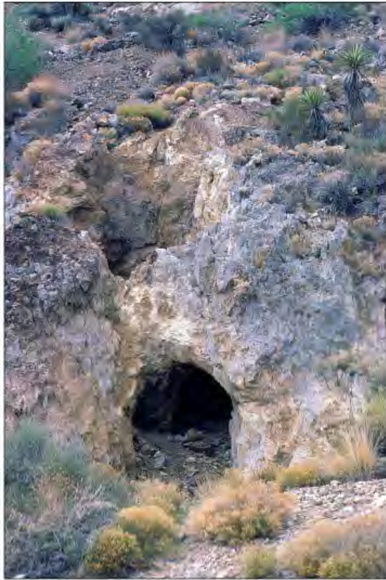
Figure 3.11. Unreinforced adit portal, C&K Mine, Providence Mountains State Recreation Area, San Bernardino County, 1989 (photograph by Karen K. Swope).
