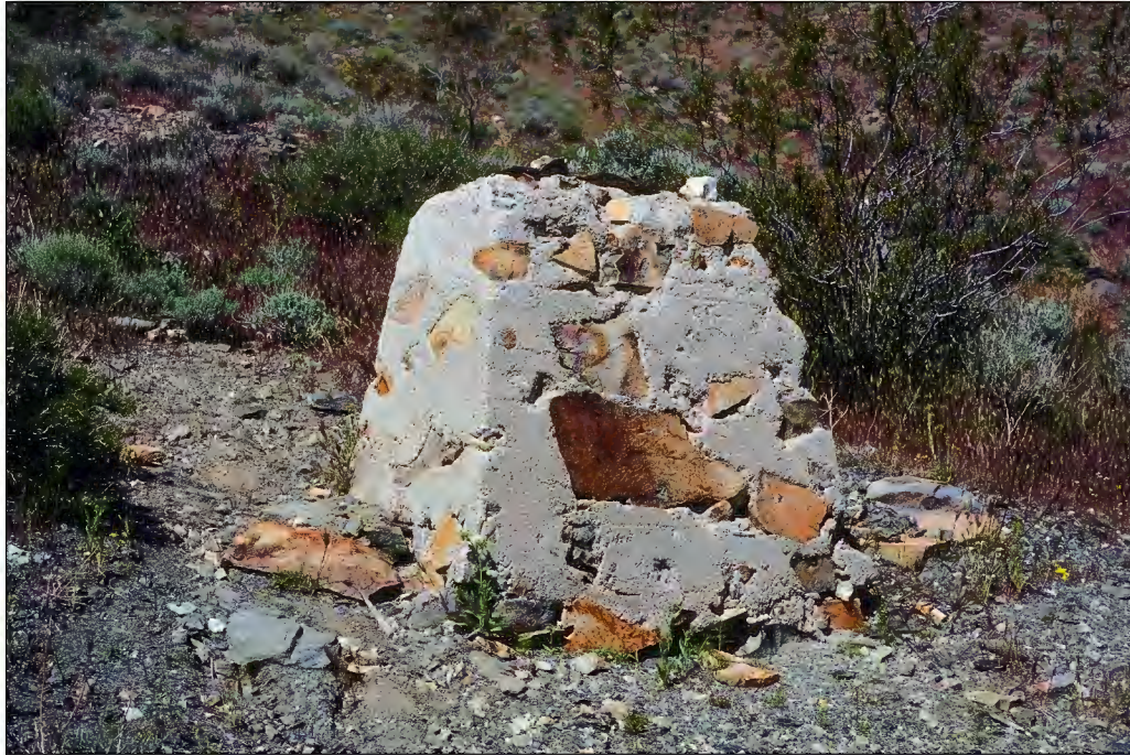
Figure 3.26. Machinery mount, Randsburg Mining District, showing the incorporation of very large rocks in the concrete construction, 1993 (photograph by Karen K. Swope).
