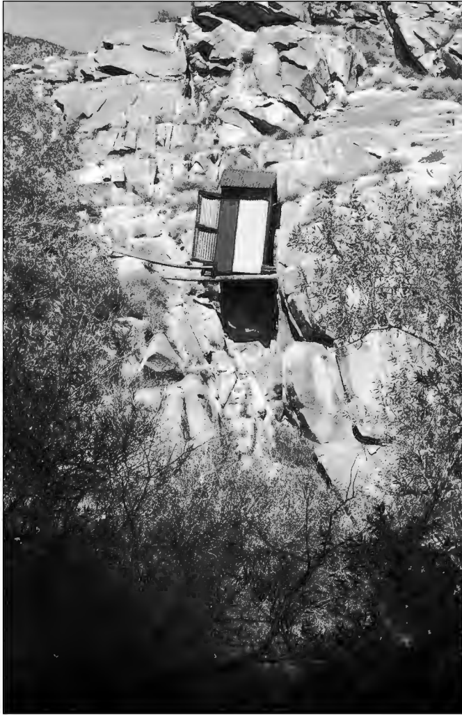
Figure 3.48. Outhouse built over an open drop instead of over an excavated pit, accessed by a suspended plank, Beveridge, Inyo County, 1991 (photograph by Karen K. Swope).
