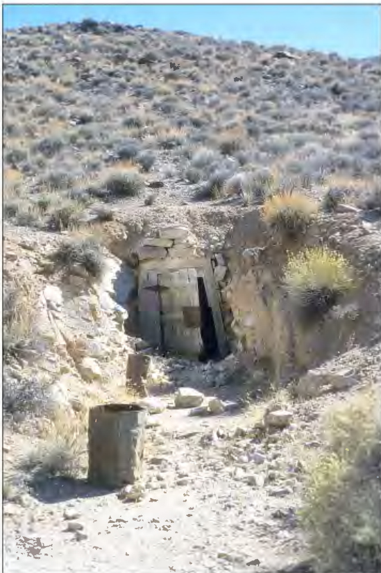
Figure 3.12. Reinforced adit portal, Skidoo, Death Valley National Monument, 1999, (photograph by Karen K. Swope).
