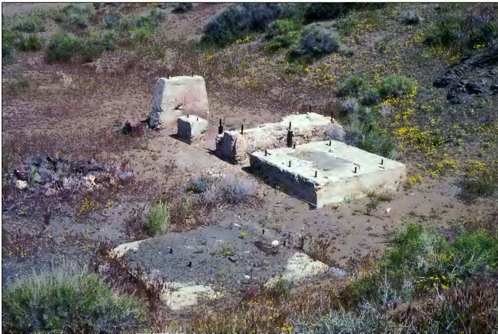
Figure 3.25. Poured-concrete machinery mounts, Rand Mining District, 1993 (photograph by Karen K. Swope).
