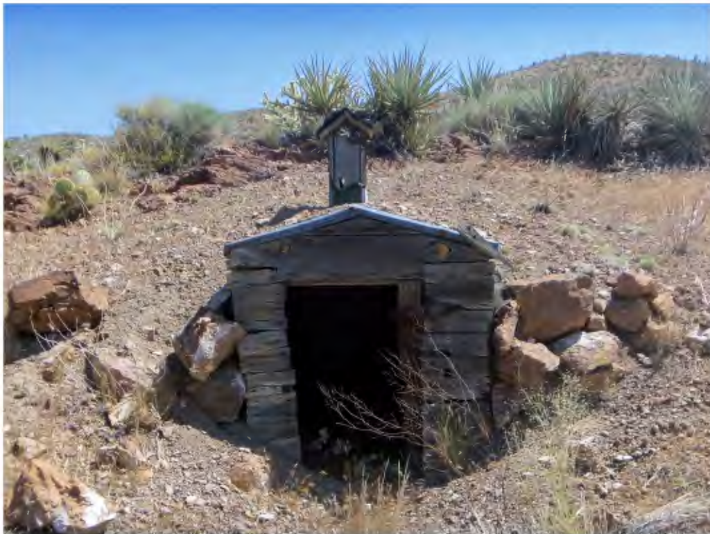
Figure 3.41. Dugout powder-storage facility, Birthday Mine, San Bernardino County, 2011 (photograph courtesy of Statistical Research, Inc.).
