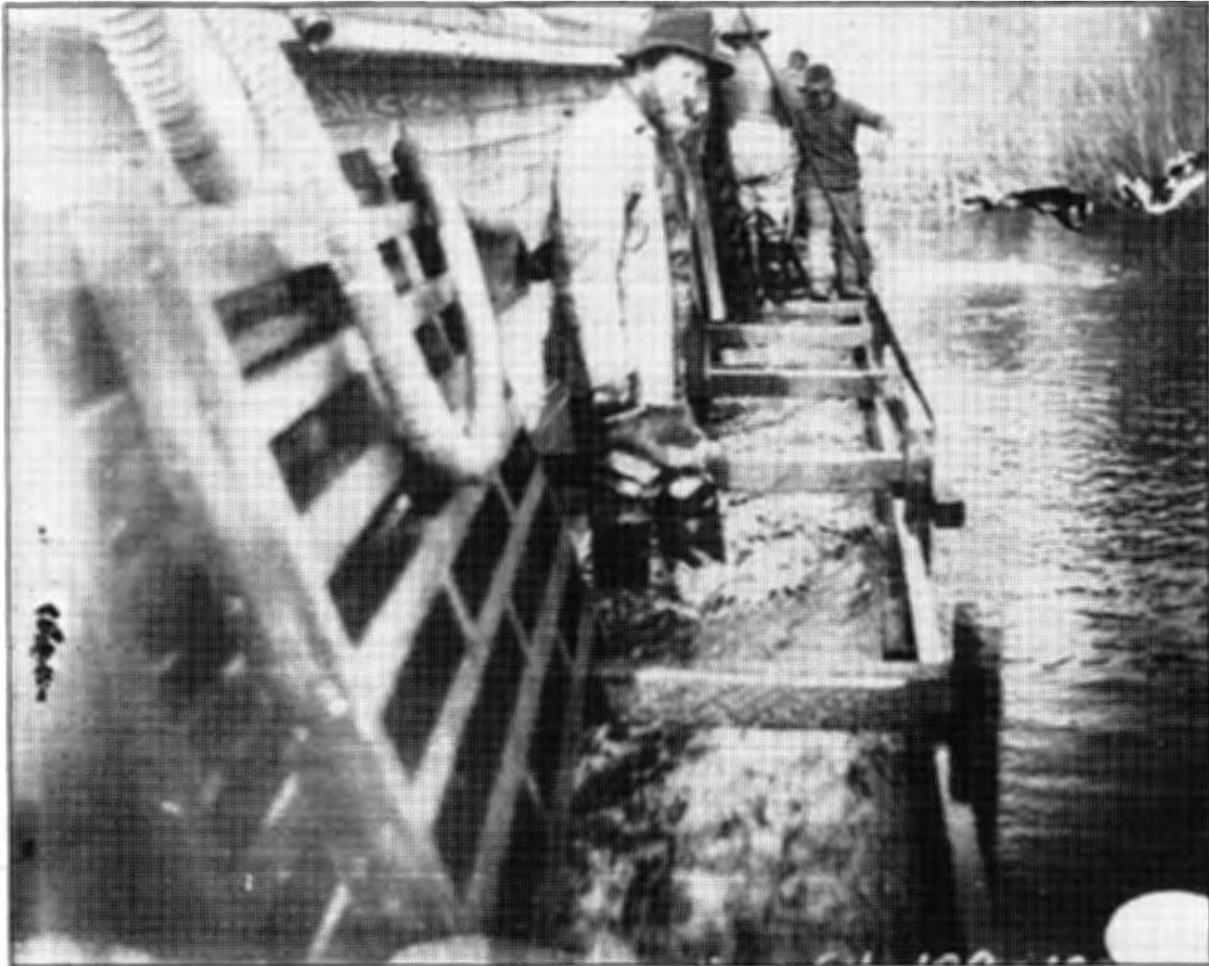
*Figure 7. Sluice attached to the Arctic Boy, which wintered in Mike Hess Creek, 1898–1899. Courtesy of the Merritt N. Murphy Collection, University of Alaska Fairbanks. Accession Number 64-100-103.*
