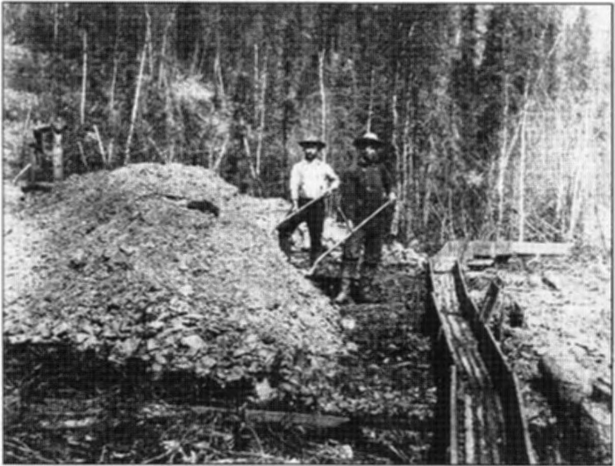
*Figure 6. Unidentified Rampart miners sluicing winter tailings, 1898. Courtesy of the George B. MacGowan Collection, University of Alaska Fairbanks. Accession Number 92-096-35.*
