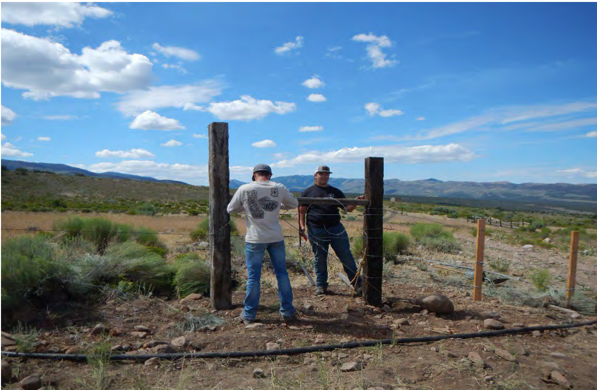
YCC Crew Members Working on a Fence in 2019
