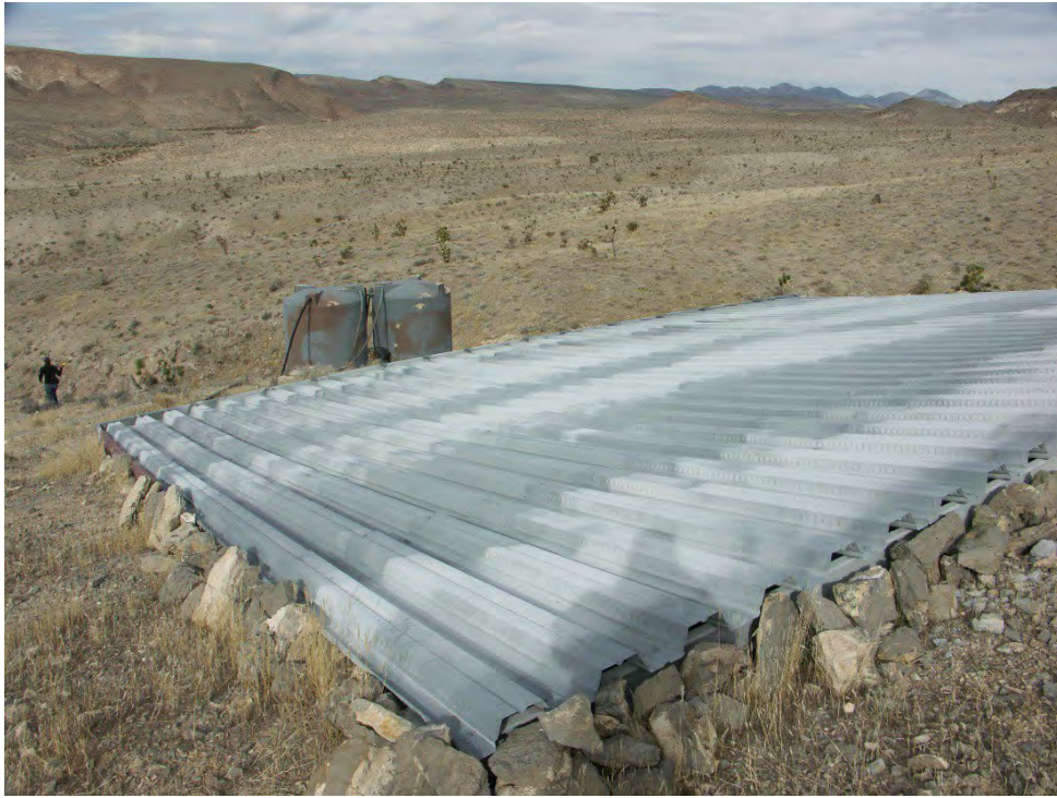
Figure 1. Existing apron and upright tanks at the Enclosure Ridge project. Both apron and tanks need to be replaced due to age and upgraded to create larger precipitation collection and storage capacity.
