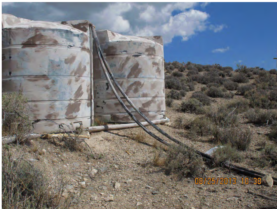
Figure 4. Existing tanks at the Saddle Mountain project. The tanks are in poor condition and the earth beneath the tanks is eroding away, the tanks will be replaced.
