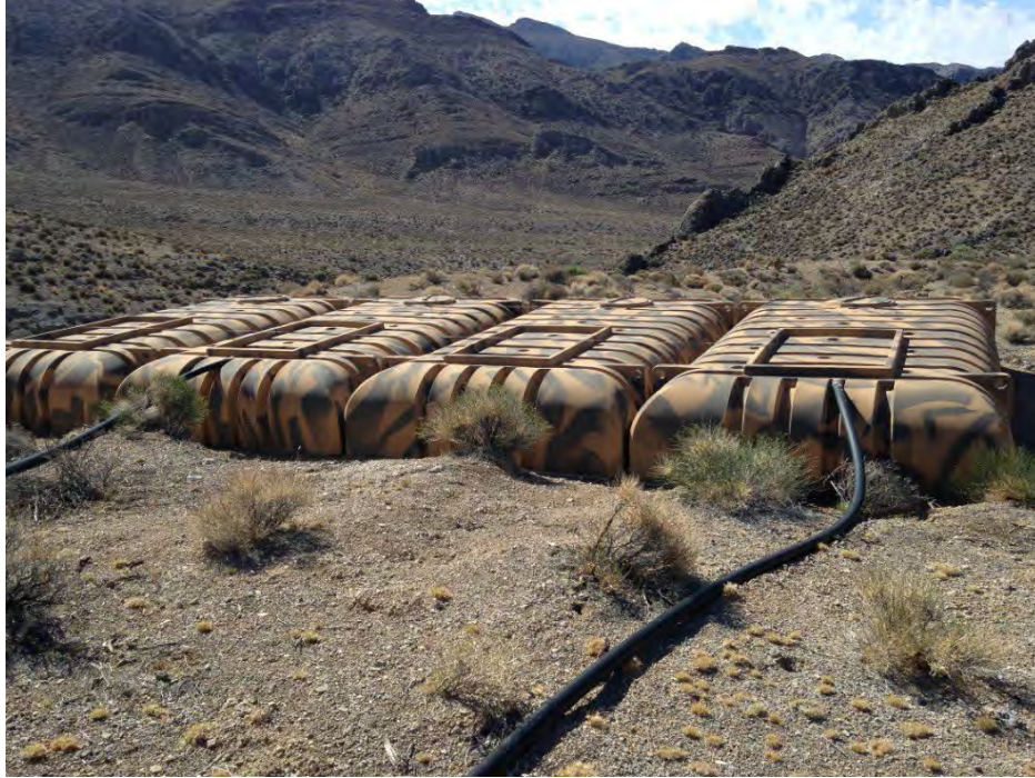
Figure 5. An example of the new, larger capacity flat tanks utilized in the modern guzzler design. These are the tanks at the already updated Joe May project.
