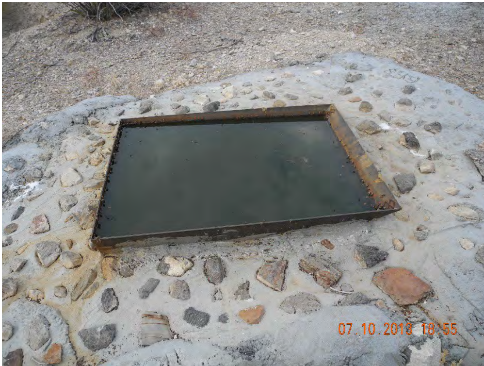
Figure 6. Example of a self-leveling drinker at the White Sage Gap project. There are no moving parts which lowers maintenance needs at this site. All upgrades and new projects will use this design.
