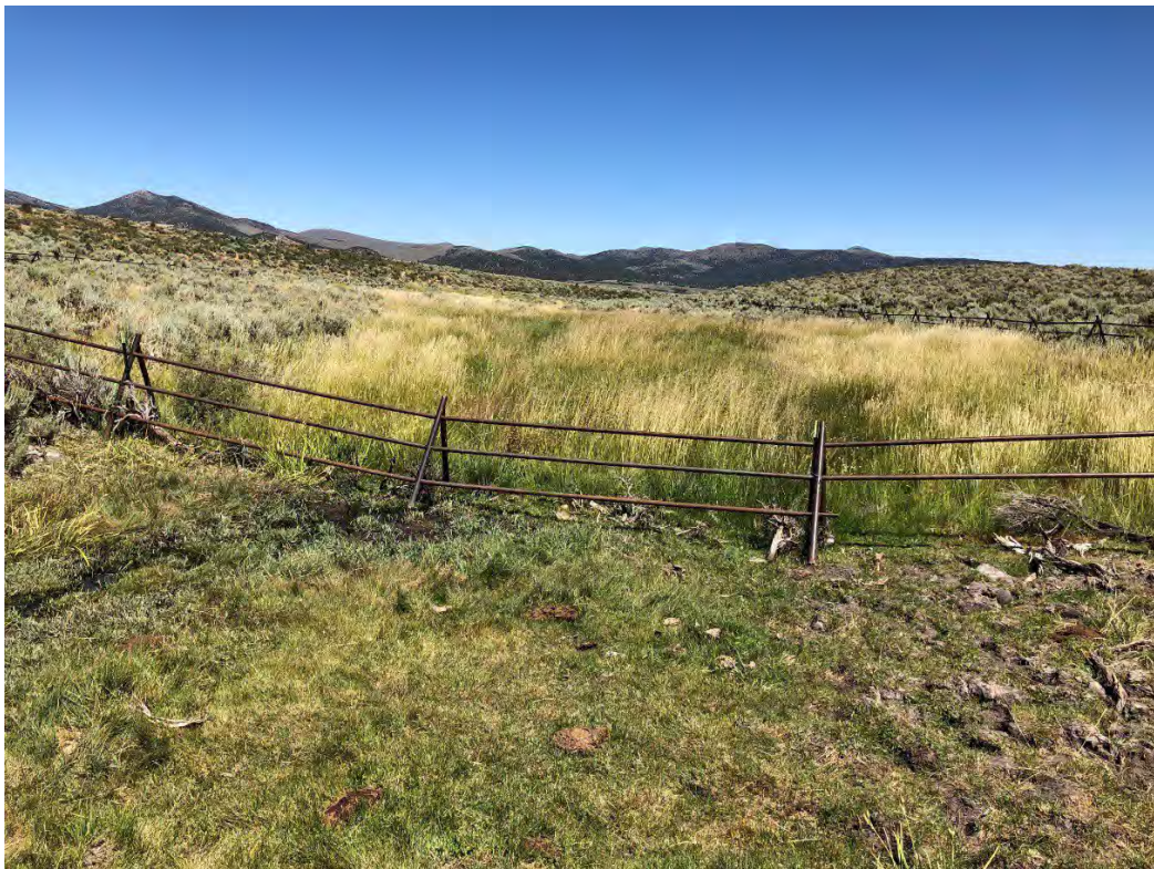
Pipe Rail Riparian Exclosure Fence Constructed by a YCC Crew
