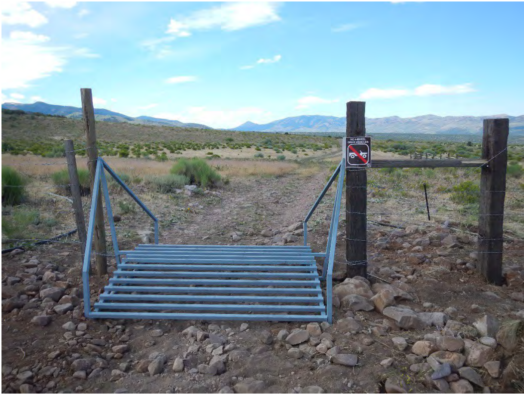
OHV Cattleguard Constructed By the 2019 YCC Crew
