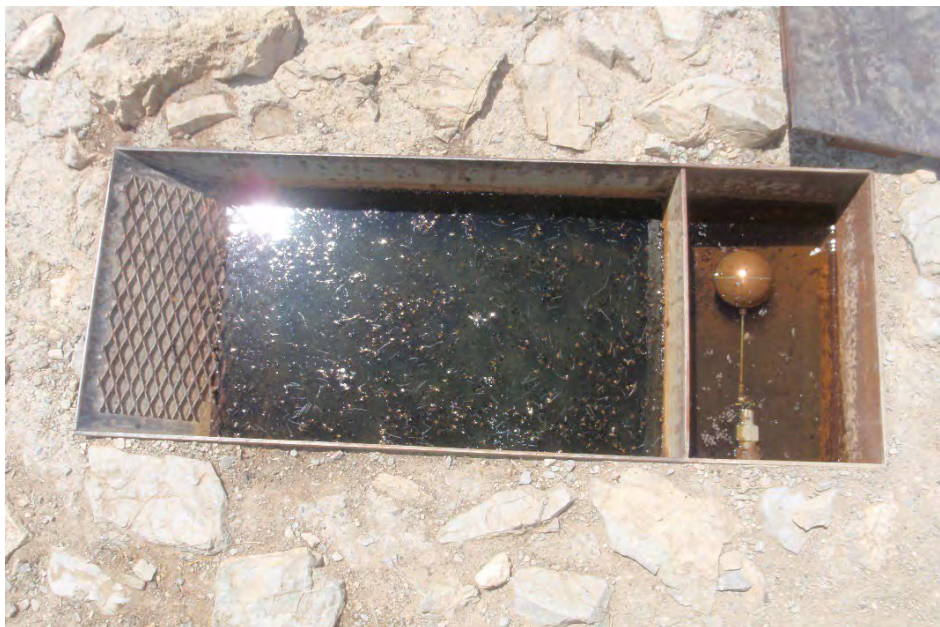
Figure 2. Old style float-valve drinker of the Enclosure Ridge project. The float-valve is the weakest link in this system, is prone to complete failure and requires regular replacement. The drinker will be replaced with a self-leveling drinker.
