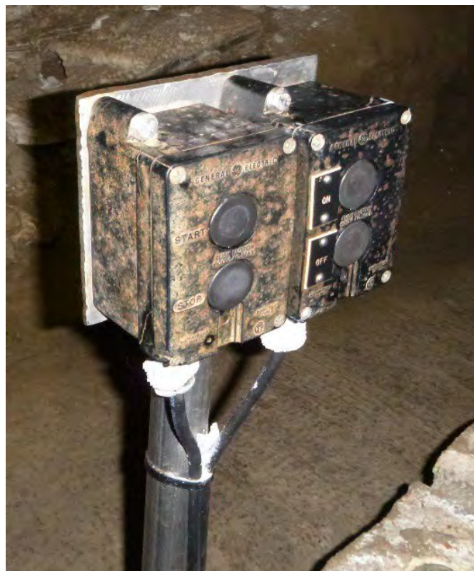
Photo 4. Switchboxes currently are corroding in the cave, and some do not even work anymore, causing sections of the lights to stay on all the time, which causes extra algae growth and heat. The new system will have easy toggle switches that are placed more frequently throughout the cave so that fewer lights are on at one time.
