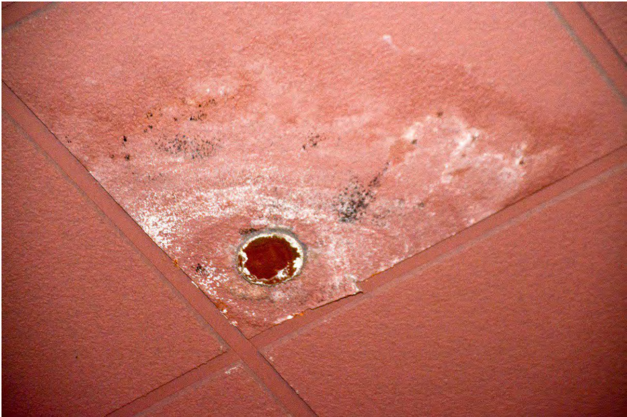
Photo 5. Photo of ceiling tile damage resulting from leaking fire sprinkler line above ceiling
