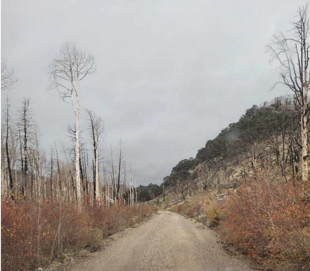
Road needing vegetation removal, regrading, and some base material added.
