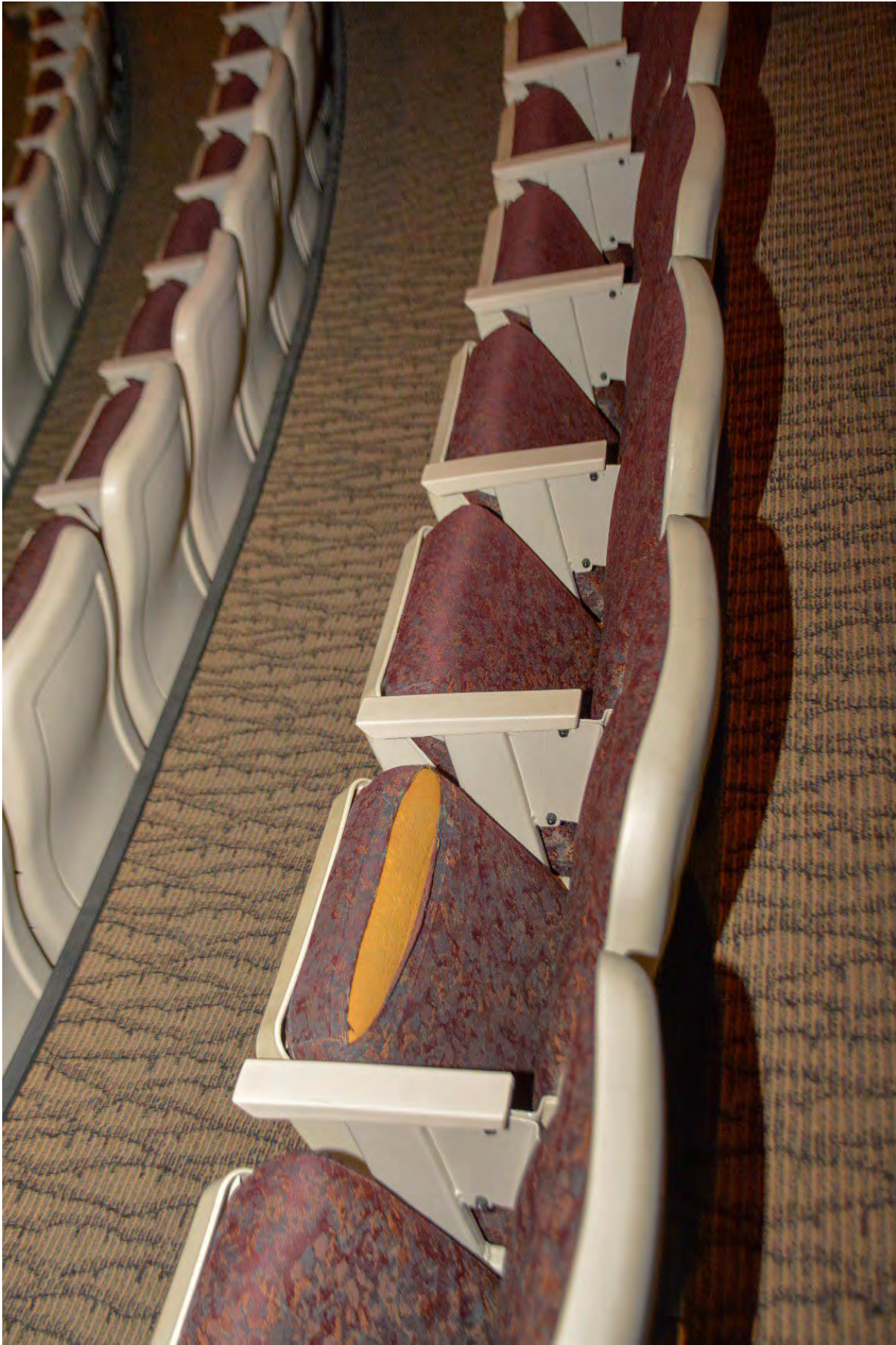
Photo 3. Photo of torn theater seating fabric and cushioning exposed
