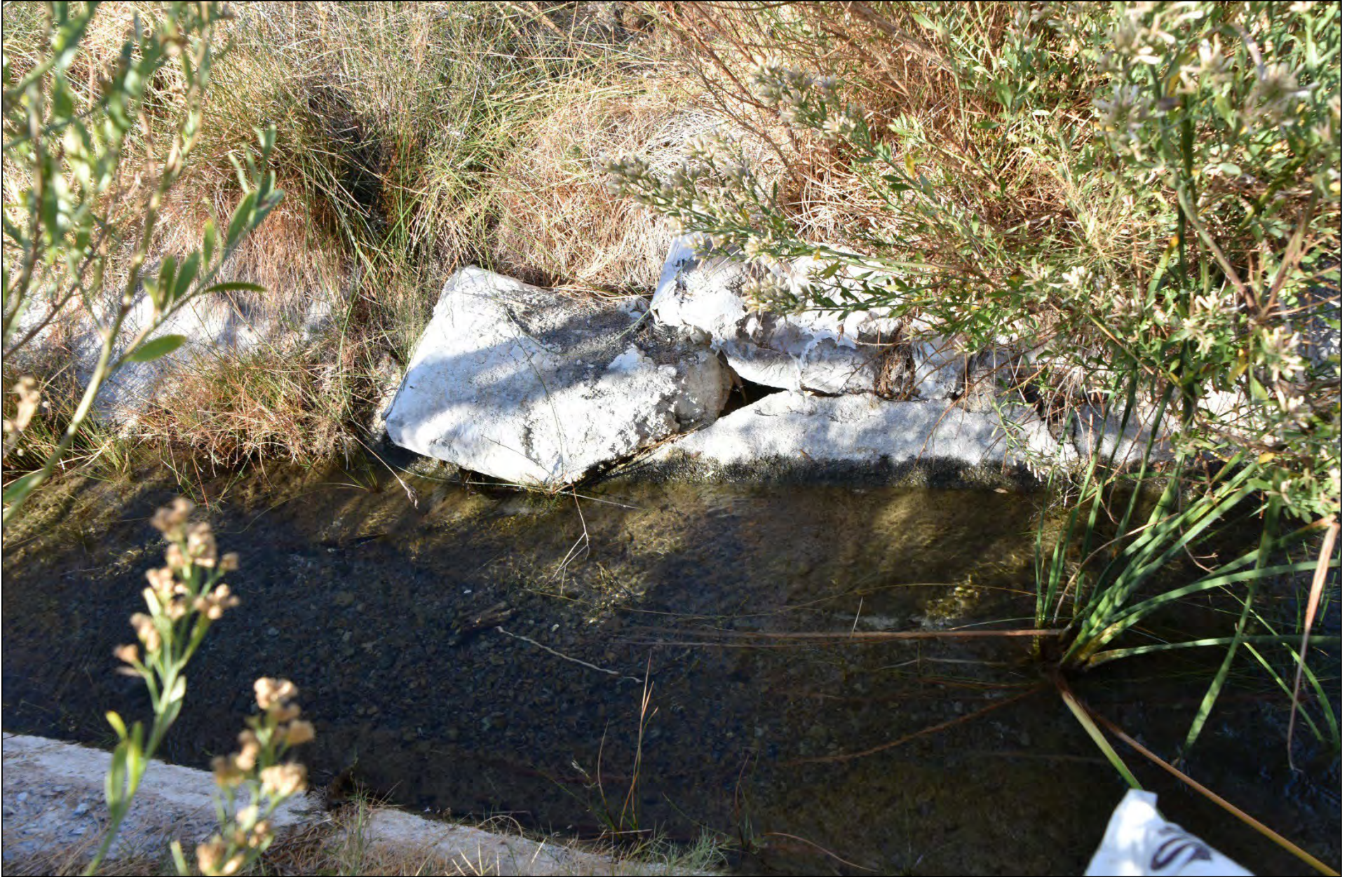
Figure 4. Example of deteriorating concrete irrigation ditch that is nearing the end of its lifespan. Breaches in these ditches cause road flooding and provide routes for movement of invasive species.
