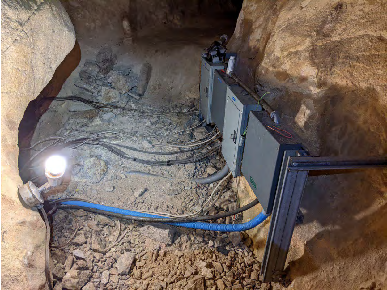
Photo 5. The four relay stations in the cave have heaters to help keep electrical components dry. They also add heat to the cave microclimate, causing the temperature to elevate about 8 degrees Fahrenheit and relative humidity to drop about 20% when the lights are on. The new system will eliminate the need for these heaters and help restore the cave climate to a more natural state.
