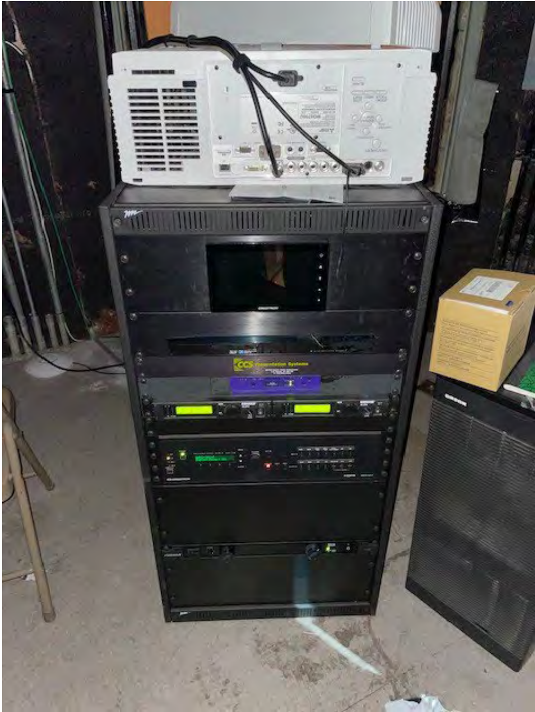
Photo 6. Photo of existing A/V equipment in projector room
