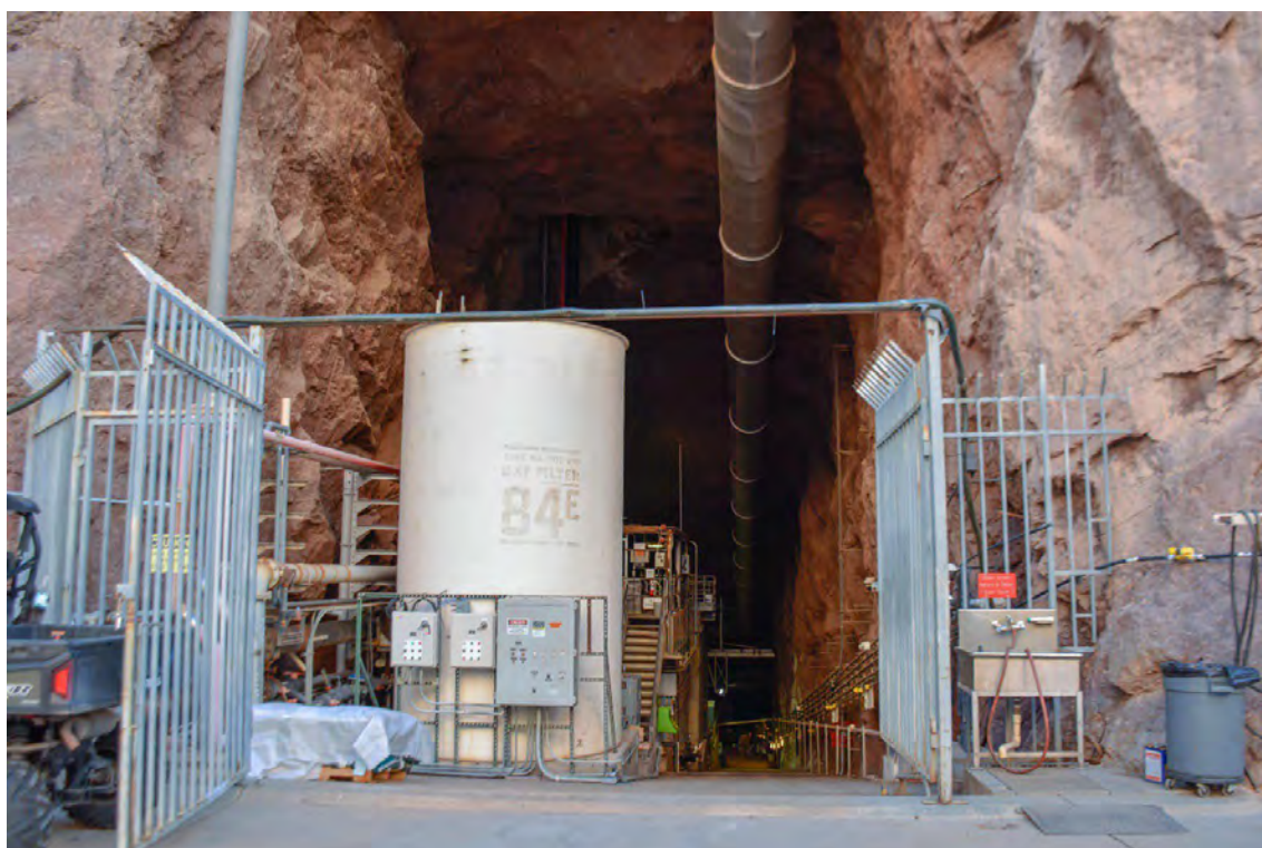
Photo 2. Wastewater tank currently in place
