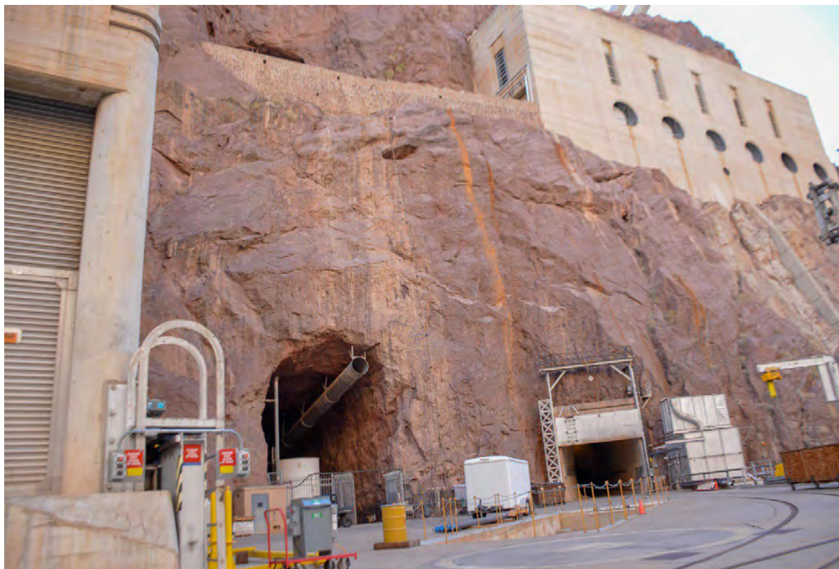
Photo 1. Tunnel in Arizona canyon wall where wastewater treatment system is located. Water treatment system is located in the upper Arizona valve house.
