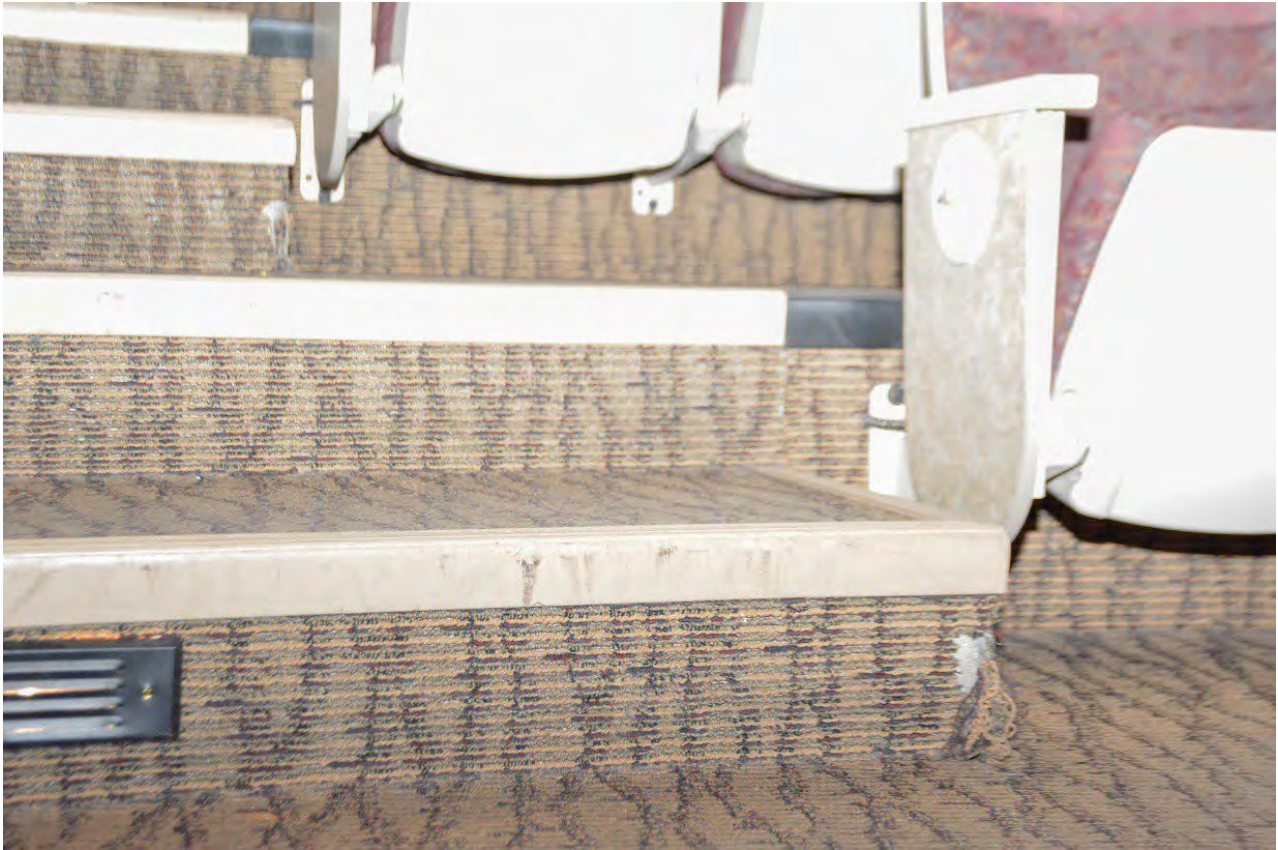
Photo 4. Photo of worn and torn carpeting at stair riser
