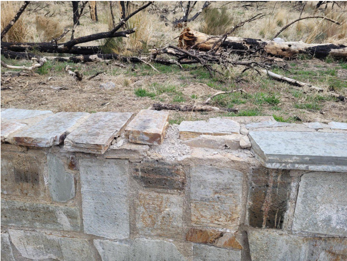
Rock wall that needs repair.
