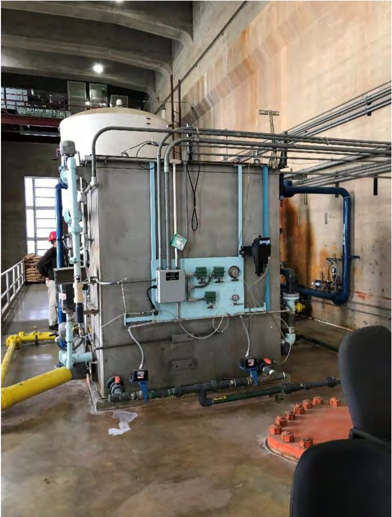
Photo 4. Water Treatment Plant Clarifier/Filter unit inside Arizona Valve House
