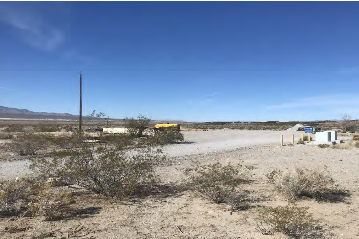
Nevada Zone Fire Complex Site Photo View North
