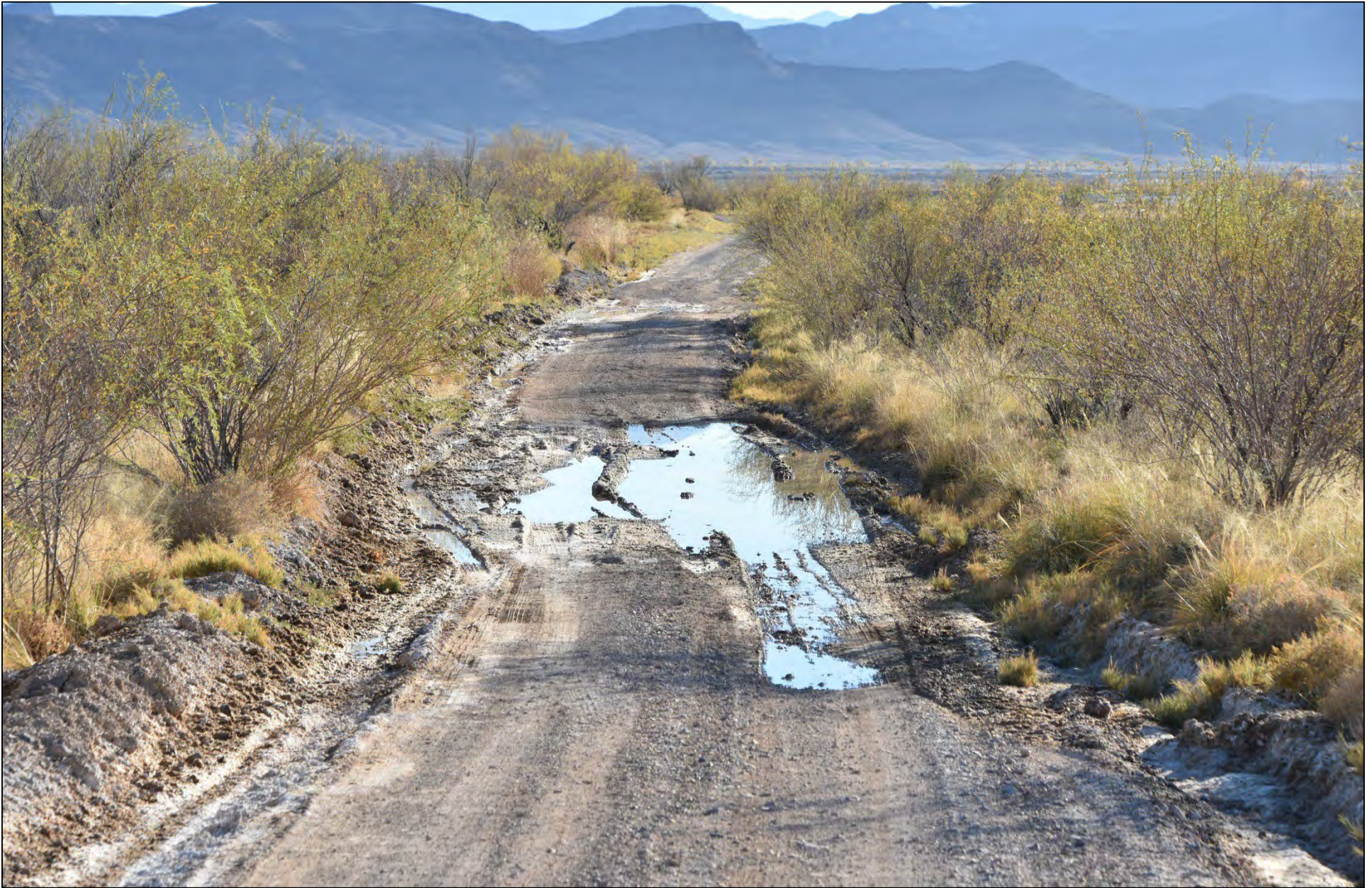
Figure 3. Example of road flooding caused by deteriorating concrete irrigation ditches in the Crystal Spring outflow system. Road improvements and reclamation of irrigation infrastructure will reduce these problems.
