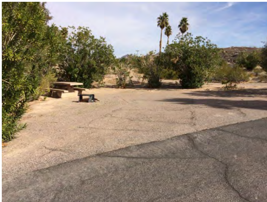
Existing Condition at Callville Bay Campground
