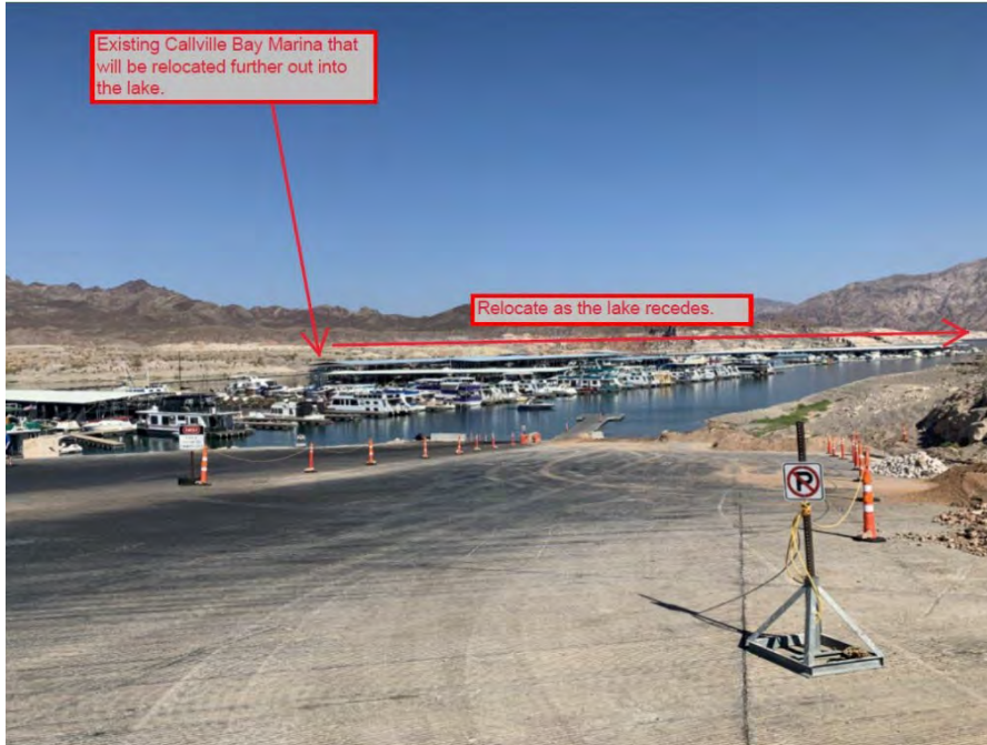
Relocation of Callville Bay Marina needed as the lake elevation recedes.
