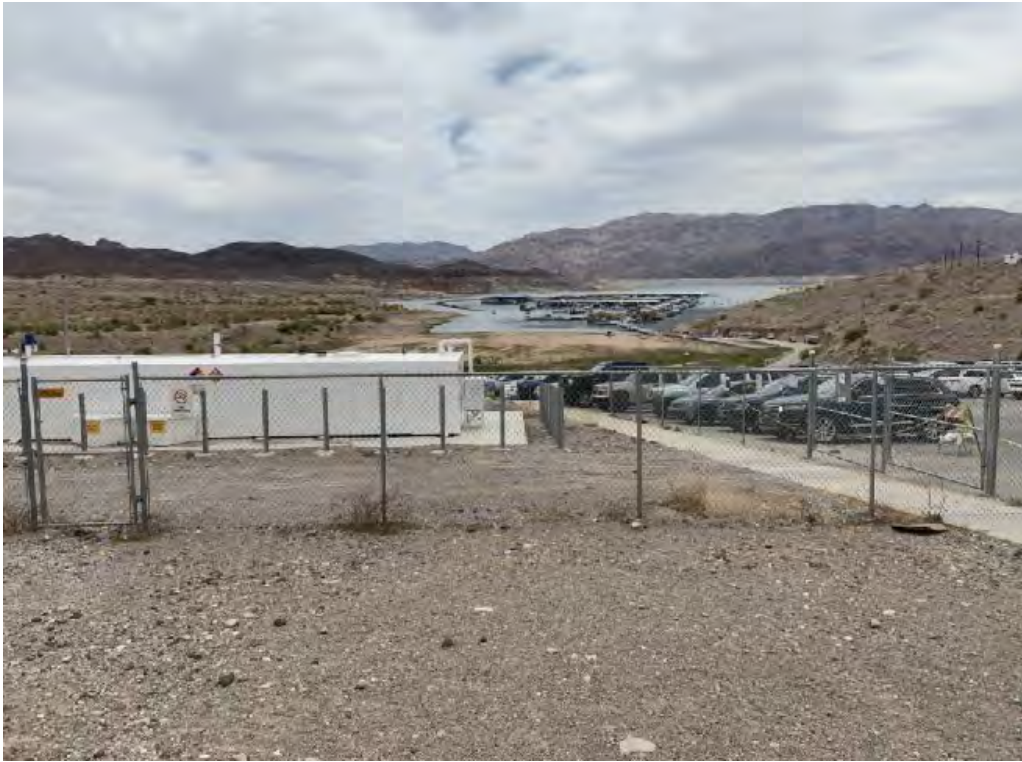
Existing Callville Bay Marina and Boat Launch at 1068 Foot Water Surface Elevation
