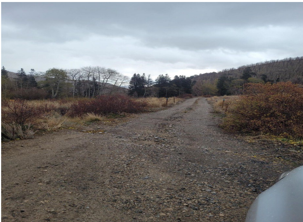
Road needing vegetation removal, regrading, and some base material added.
