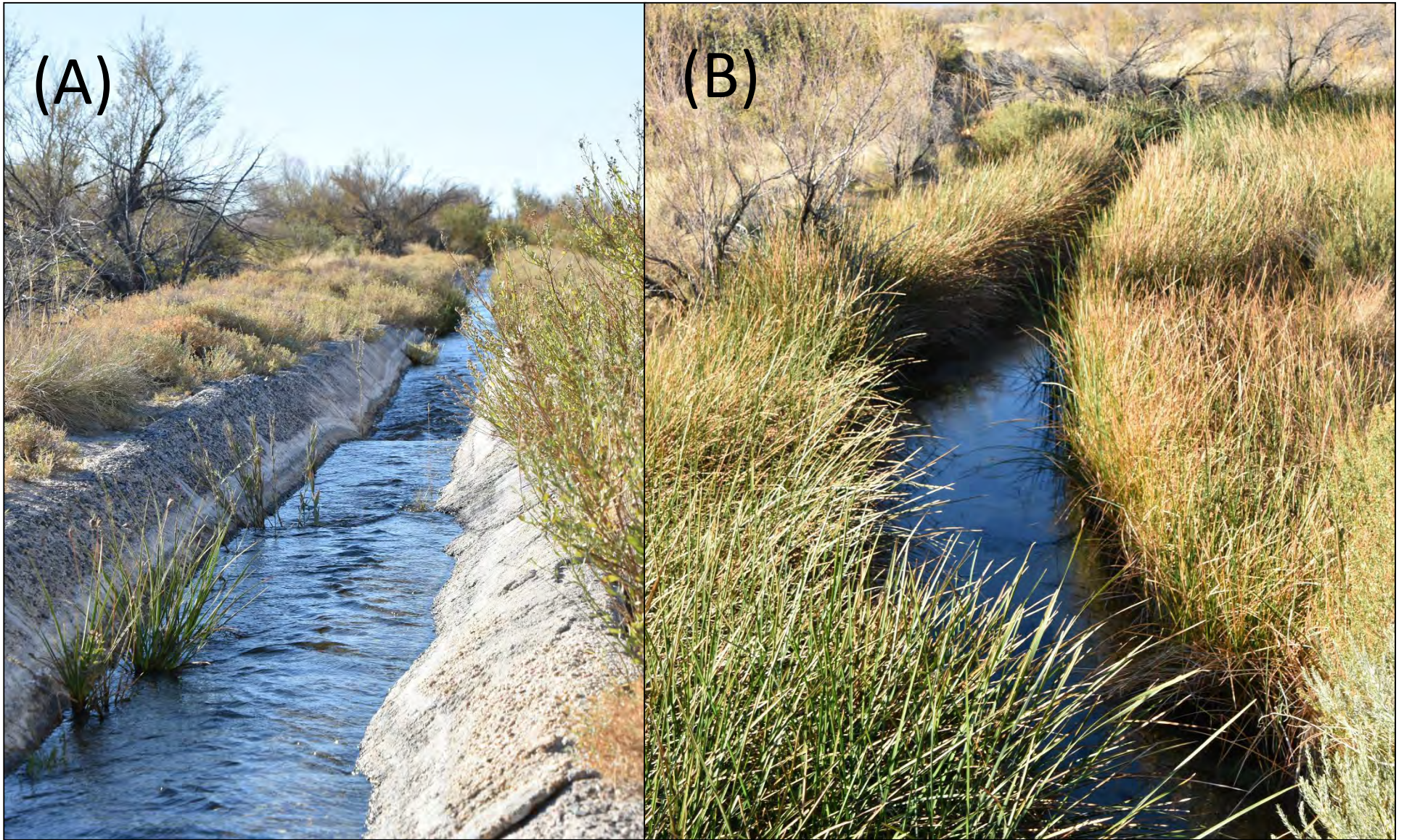
Figure 2. Existing concrete irrigation ditch (A) in contrast to restored spring outflow channel (B) from upper Crystal Spring outflow system. The current irrigation water delivery system has little habitat value for native species yet requires significant attention to limit road flooding and the spread of invasive species.
