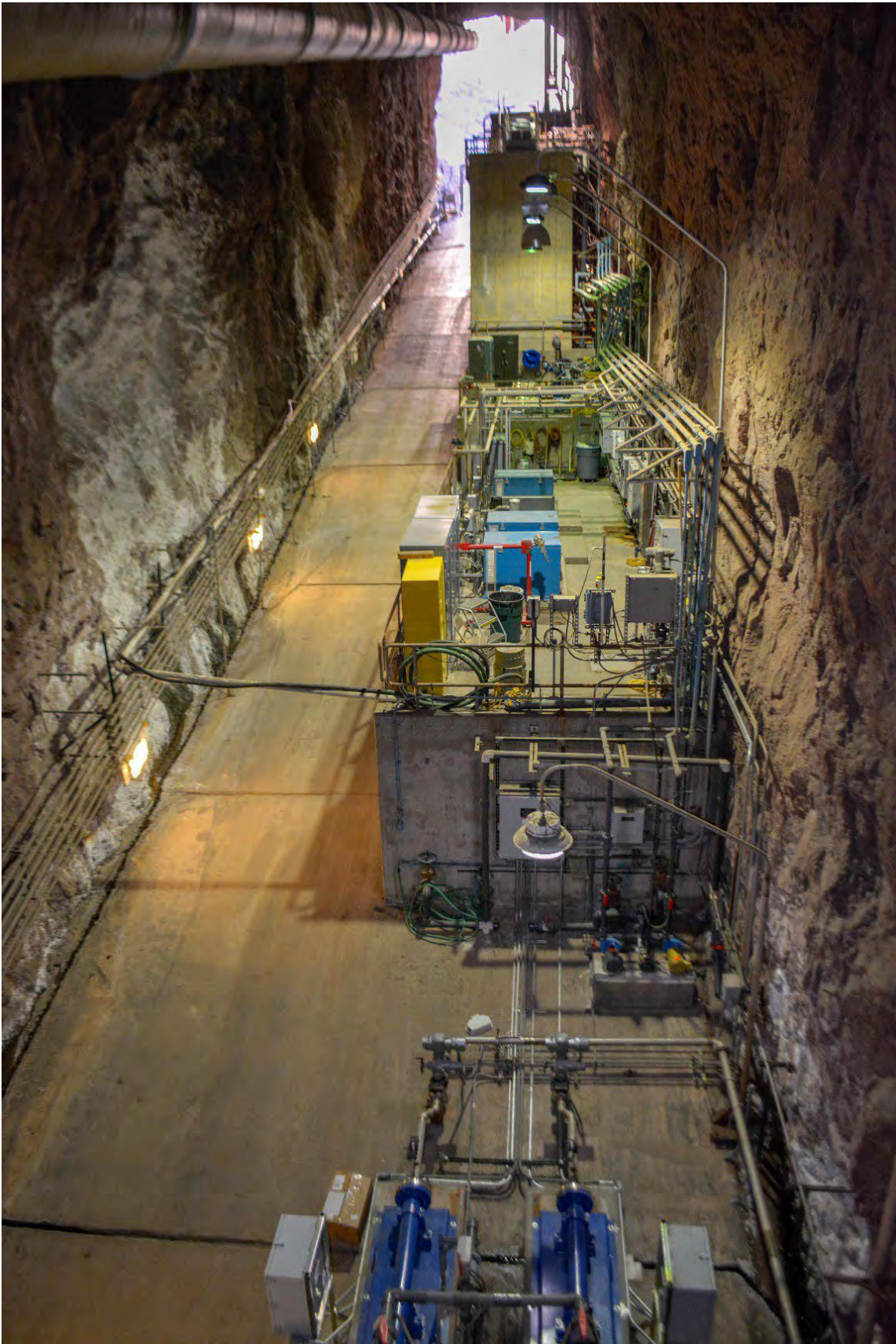
Photo 3. Photo of Wastewater treatment system from inside tunnel
