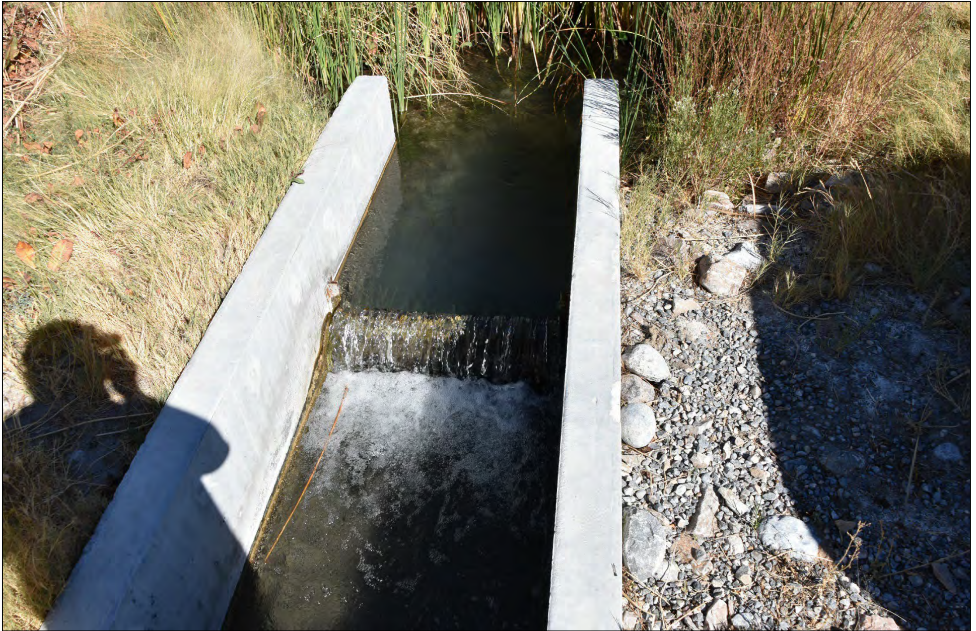
Figure 5. Example of removable fish barrier. Nonnative fish introductions have been common at Ash Meadows NWR. Barriers such as these will help manage current infestations and contain future introductions.
