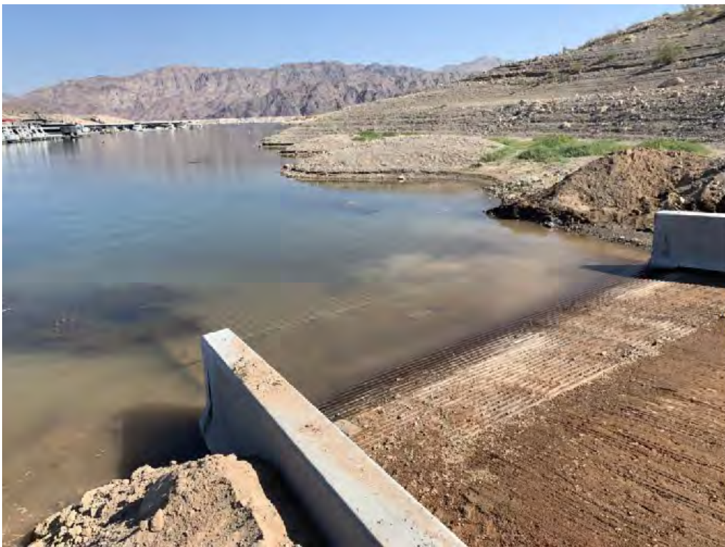
Existing Boat Launch with receding lake elevation. NPS uses pipe mat to connect the existing concretelaunch to the launch-able elevation. This launch will become unusable and dry at 1063-foot water surface elevation.
