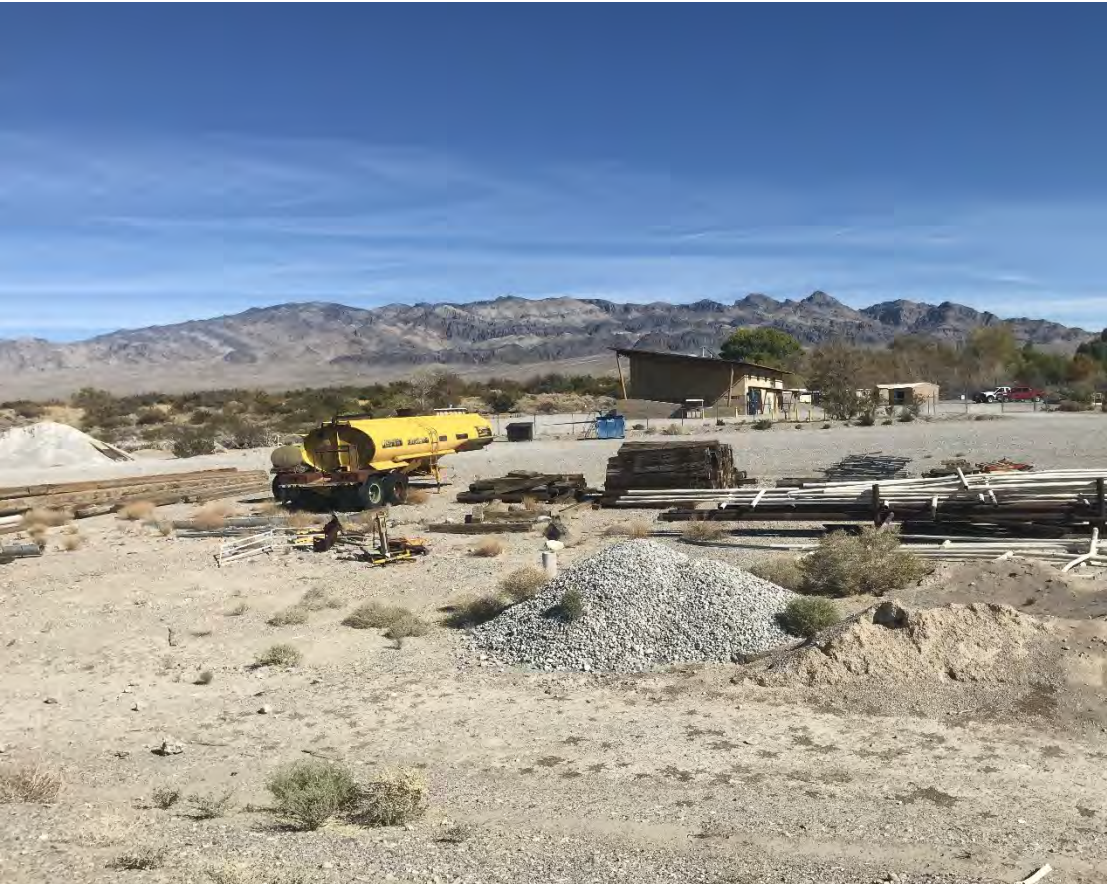
Nevada Zone Fire Zone Site Photo View East
