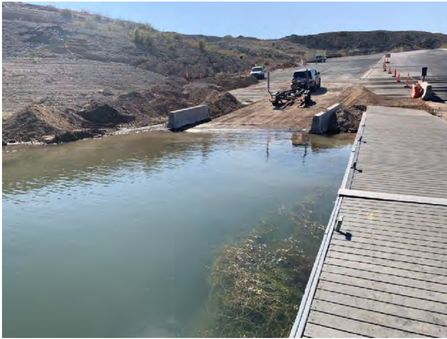
Existing Condition at Callville Bay – Reduced lanes at the Boat Launch using pipe mat as a temporary connection to a launch-able elevation.
