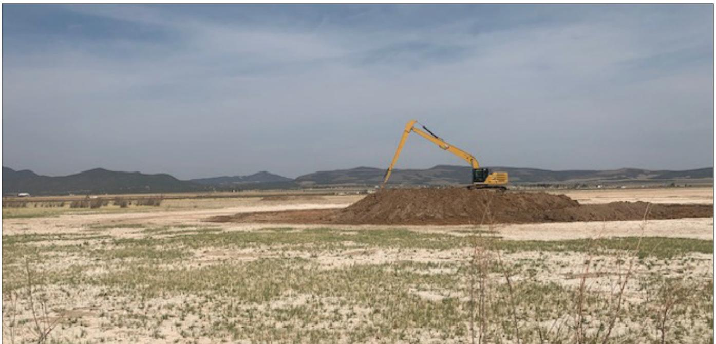
*Figure 12. Excavator beginning work on a retention pond in the dry lakebed of Quichapa Lake.*
