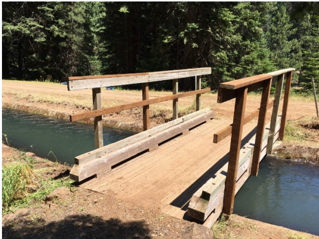
New railing on PCT bridge.
