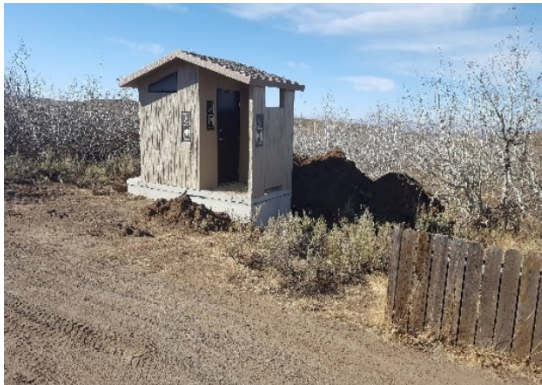
New vault toilet at Fish Lake Campground.
