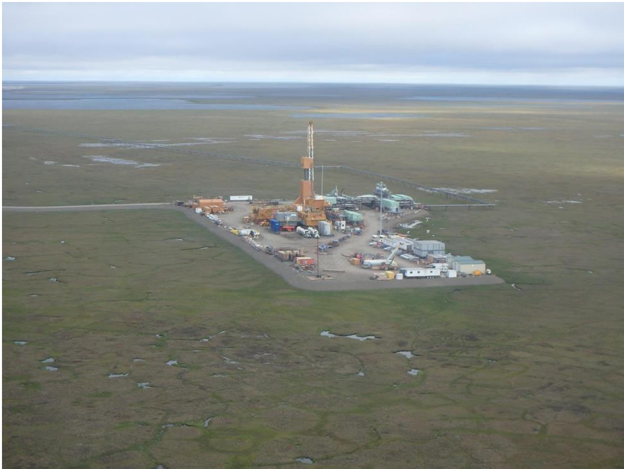
Figure 13. GMT1 drill site, pipeline, and road.
