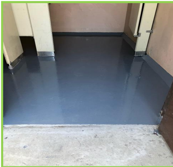
New flooring for vault toilets that improves the ability to clean and remove water out of the structure. Funded with appropriated funds. [2019]
