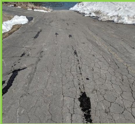
Asphalt cracking at the top of the boat ramp. BLM received appropriated funds to reseal the asphalt in 2019. [2019]
