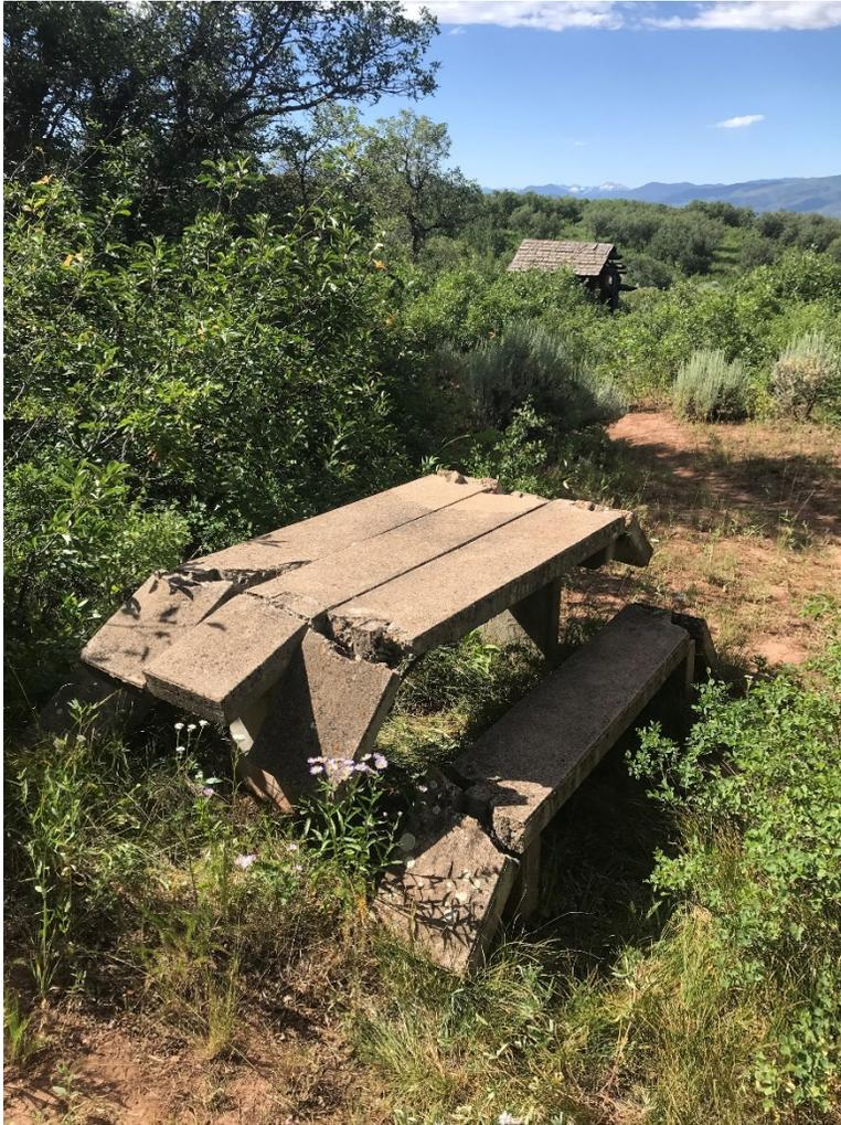
*Figure 2. Concrete picnic table: one of three identical tables to be historically reconstructed.*
