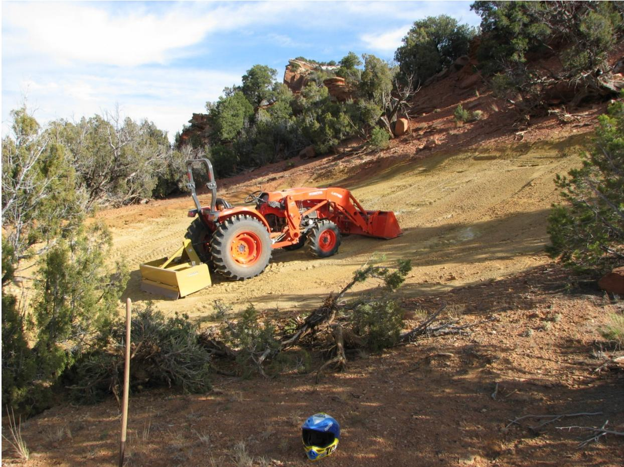
**Borrow area with heavy earth moving equipment used in backfilling operations.**
