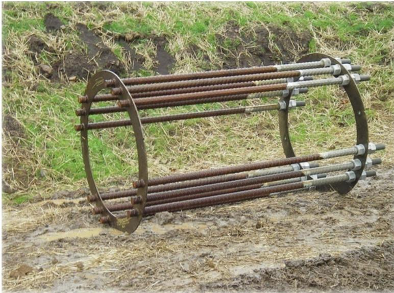
**Figure 5-16.** Mounting Bolt Cage with Concrete Forms
