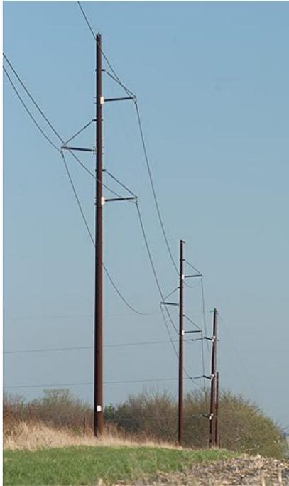
**Figure 5-5.** Single-pole Steel Dead-end
