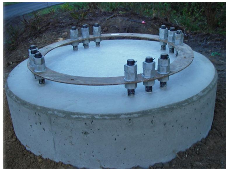
**Figure 5-18.** Single-pole Steel Structure on Concrete Pier Foundations
