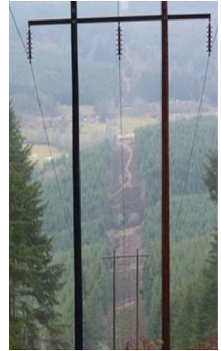
Disadvantages of wood poles include generally shorter life spans than steel poles or lattice poles, less control over the quality, higher susceptibility to fire damage, and increased risk of damage from wildlife. The high probability of damage from woodpeckers and insects can affect the decision on whether wood versus steel should be used for a given transmission line.
