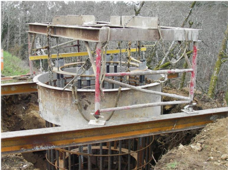
**Figure 5-17.** Concrete Pier Foundation
