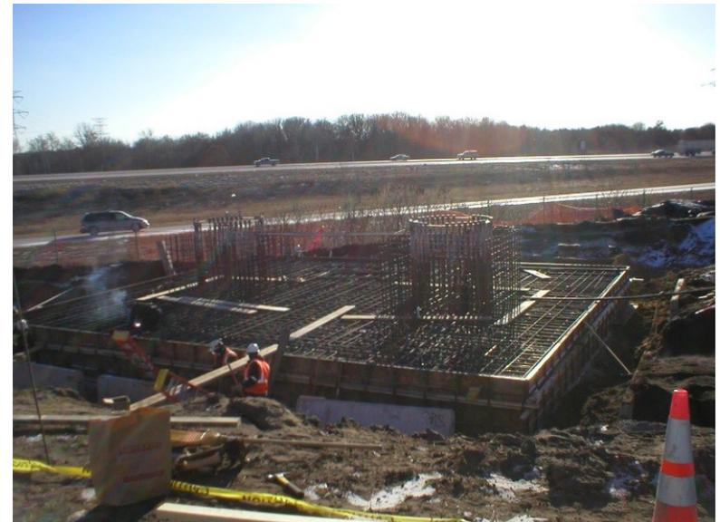
**Figure 5-21.** Grillage Foundation in Form
