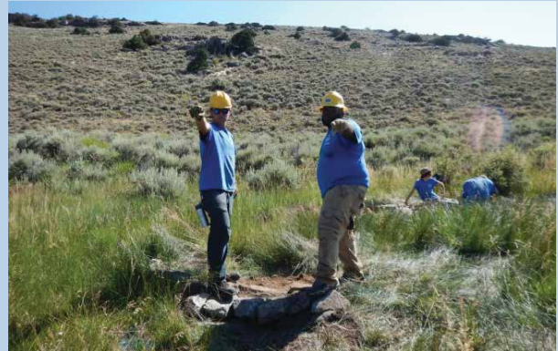
Instream structures installed in Chance Gulch by the Western Colorado Conservation Corps.
