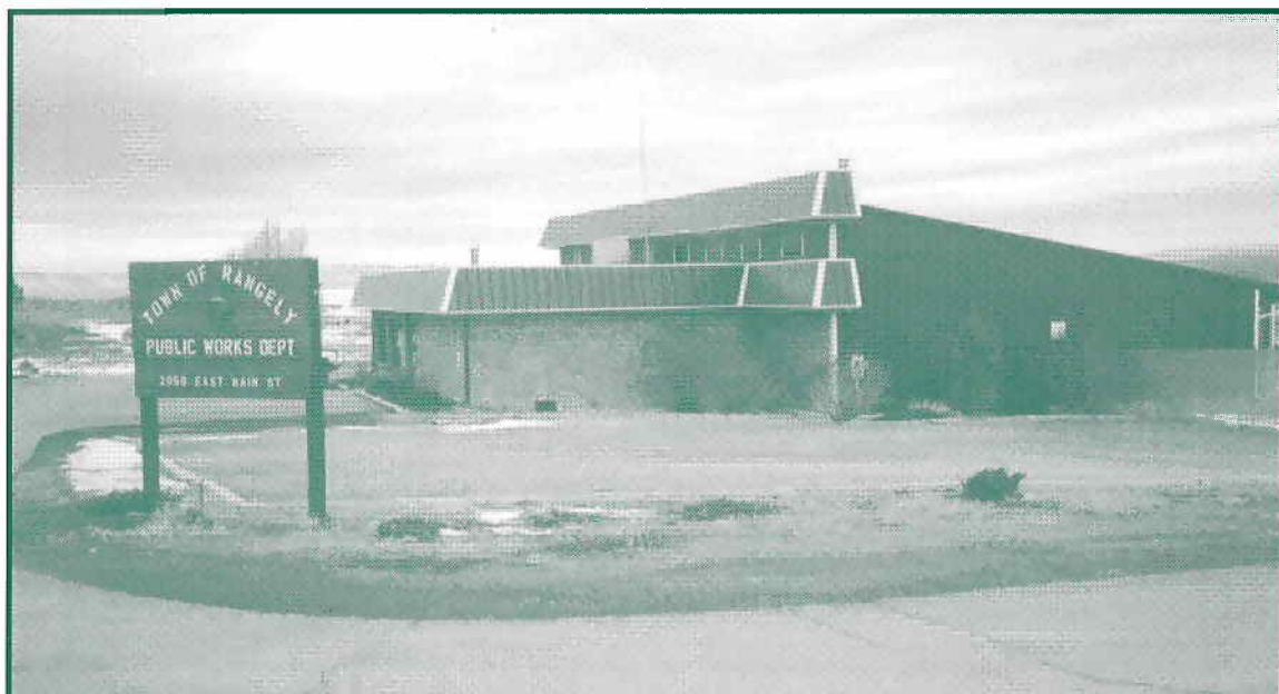
—Public Works Building, Rangely, Colorado
