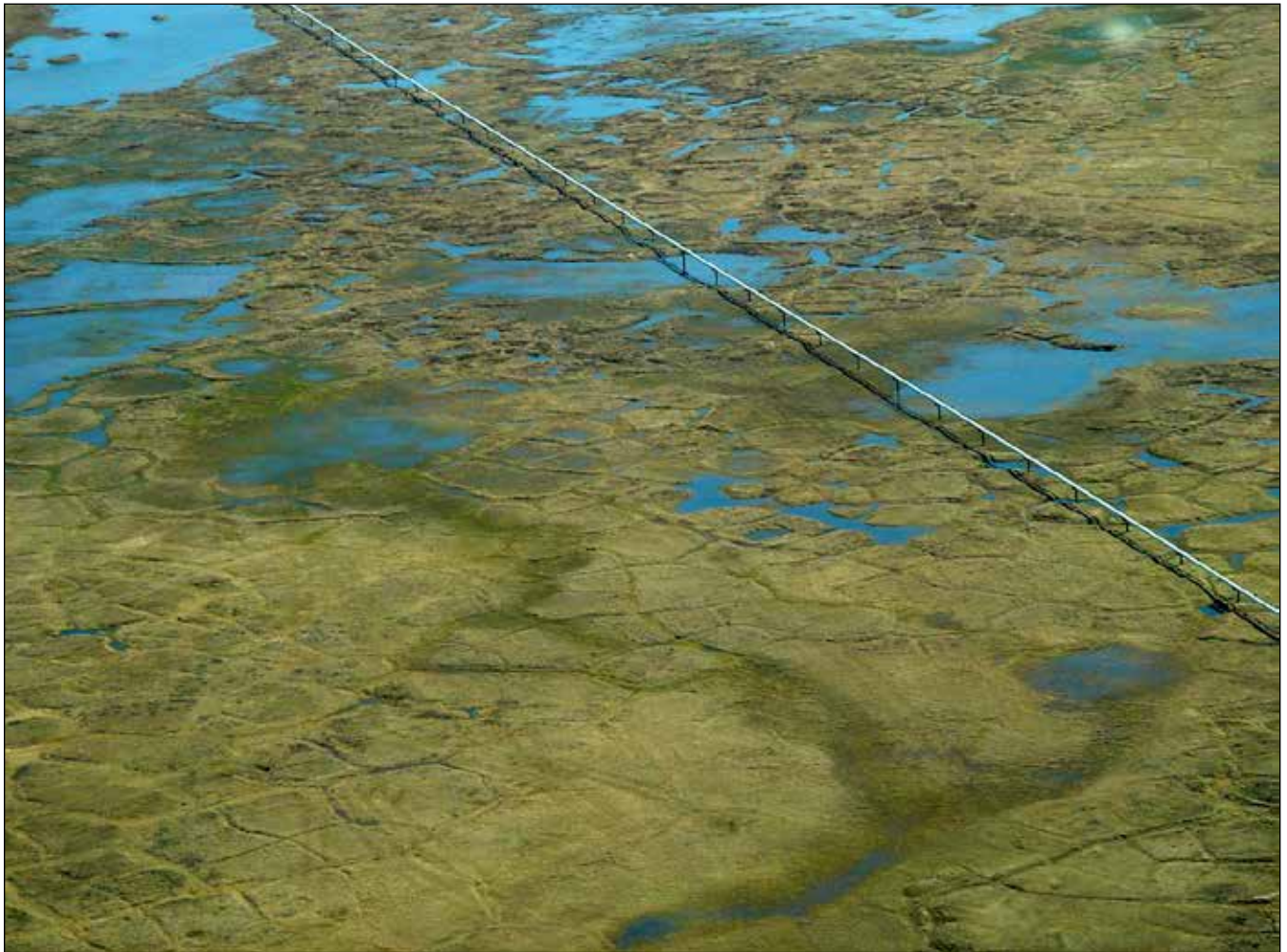
Pipeline over tundra. (USGS)
