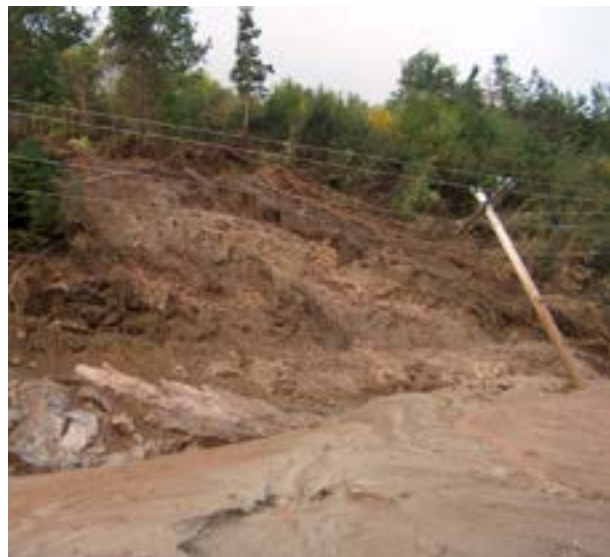
Warford, Jim. Landslides: Riverside Drive, Corner Brook. 2005. Corner Brook. Newfoundland Labrador Dept of Natural Resources. Web. 15 Feb. 2016.
