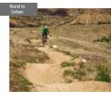
PBR Trail: Small/gentle rollers and berms, shape supported with rock materials, lots of undulations and meanders, flow adjusted to reduce speeds (to reduce breaking, sliding), soil amendments for tread shaping
