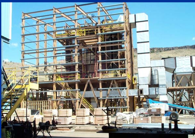
Warm Springs Forest Products Mill with Cogeneration plant.
